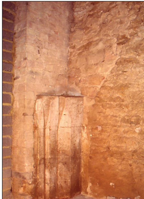
Plate 8. Springing of removed vault at south-west corner of corridor adjacent to Room G4 (X on Figures 2 & 7).
