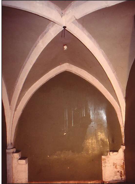
Plate 7. Room G11 vault and springing of removed canopy to entrance in south wall.
