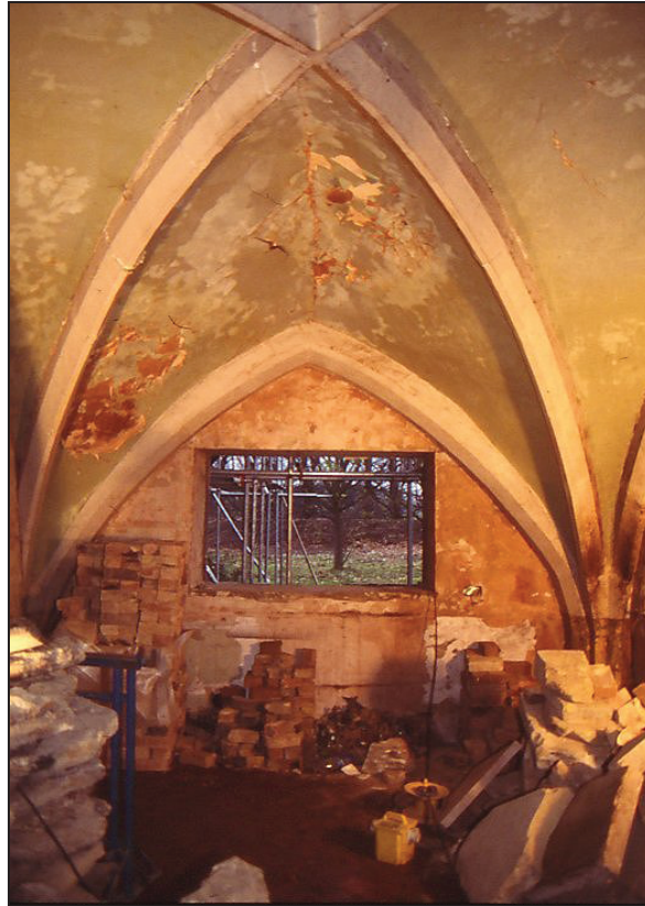
Plate 5. Vault over Room G6 with rendered 19th century brick between the stone ribs.
