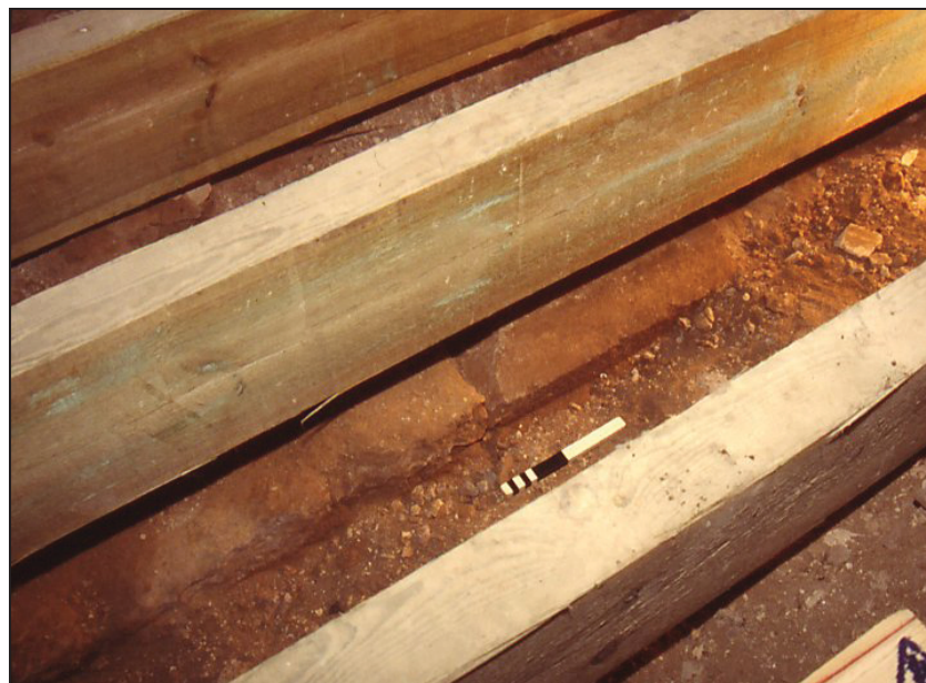
Plate 2. Chamfered stone plinth course exposed beneath modern floor joists in Room G14. To the left of the 0.2m photo scale is rubble stone blocking of what may have been an original entrance.
