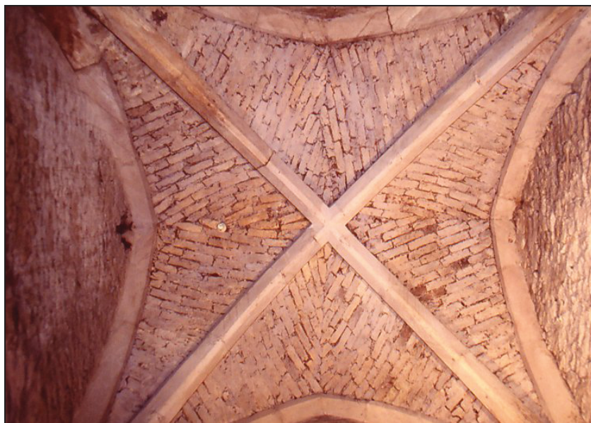
Plate 6. Vault over Room G13 with ?18th century brickwork.
