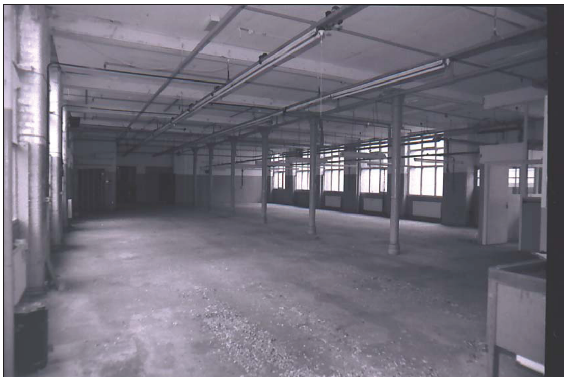
Plate 12: Yeoman Street Range, first floor. Looking northeast.
