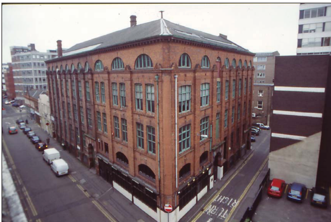
Plate 1: 17-19 Yeoman Street. Looking southwest (taken from 2nd storey of adjacent multi-storey car park).
