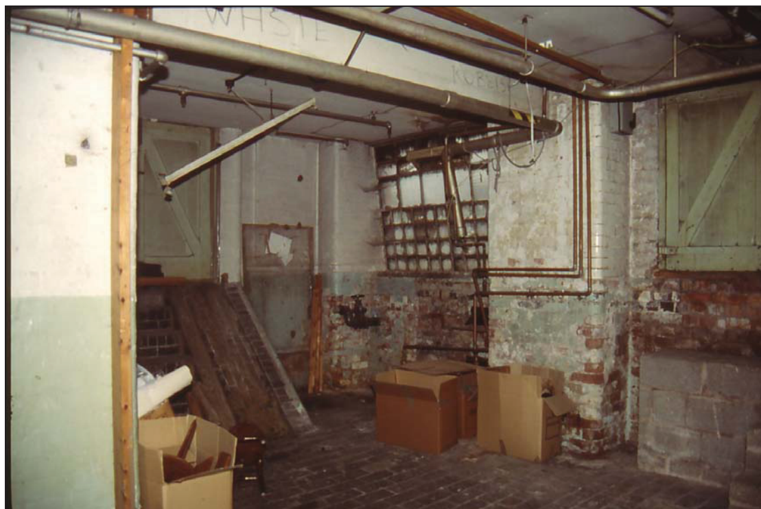
Plate 8: Yeoman Street Range, basement area. Looking north-east.
