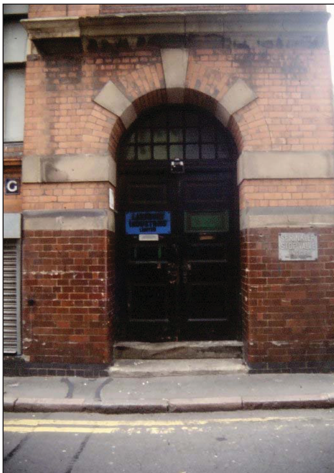
Plate 7: Pedestrian entrance on Yeoman Lane. Looking south.
