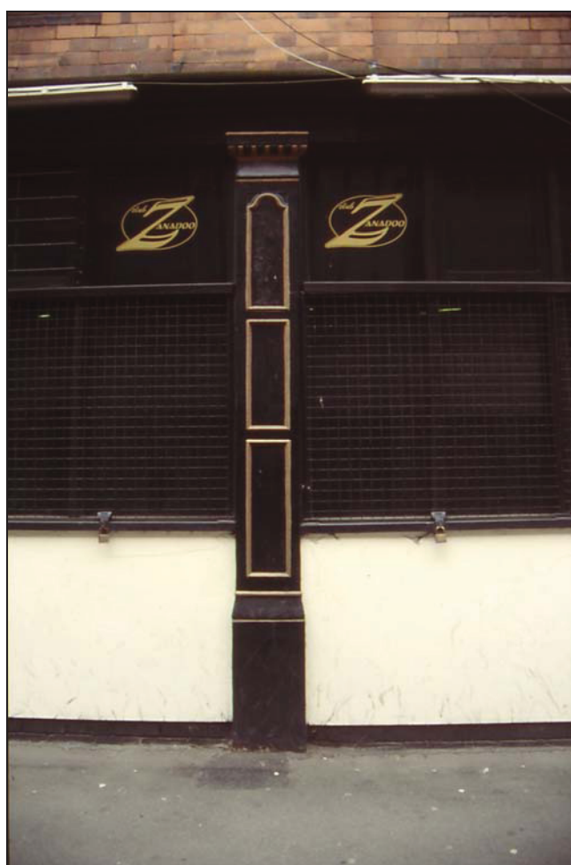
Plate 6: Detail of early cast iron column. Looking west.
