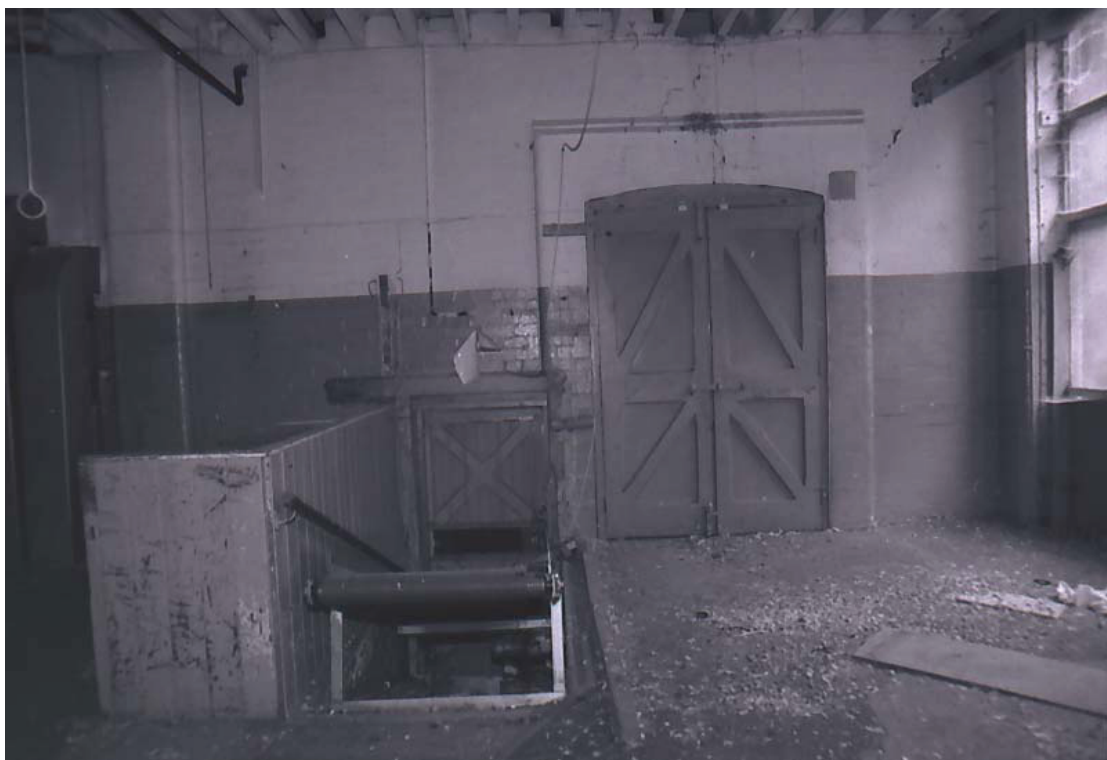
Plate 11: Yeoman Street Range, ground floor loading doors. Looking north
