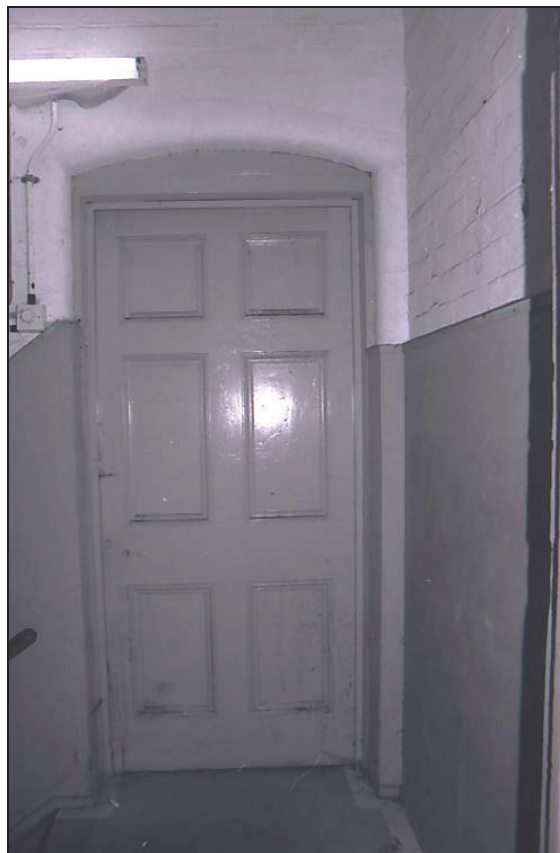
Plate 20: Yeoman Lane, ground floor: early six-panel door off stairwell. Looking east.
