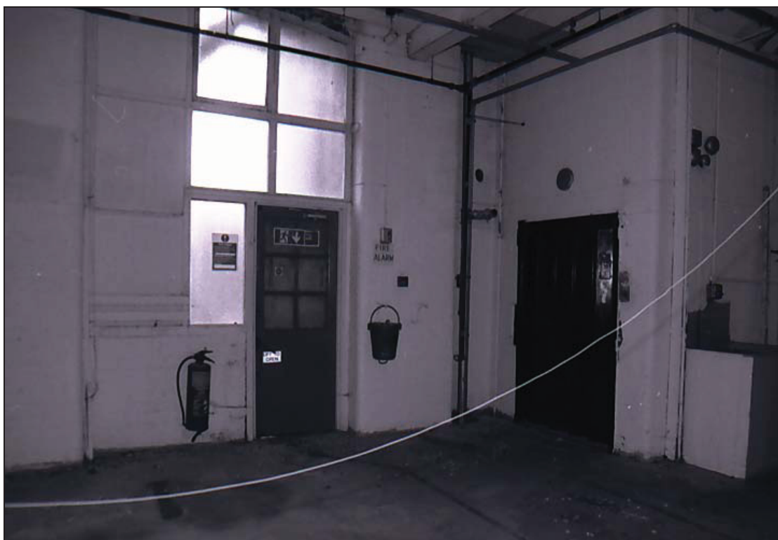
Plate 14: As above, early fire doors. Looking northwest.
