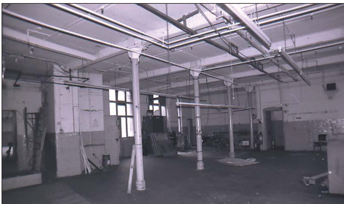
Plate 21: Yeoman Lane, 1st floor level. Looking southwest.
