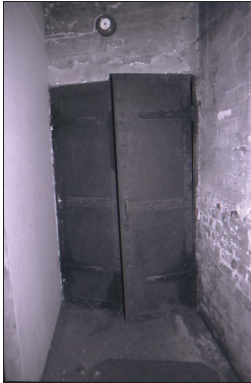
Plate 19: Yeoman Lane Range, early cast-iron, lift-shaft fire doors. Looking east.
