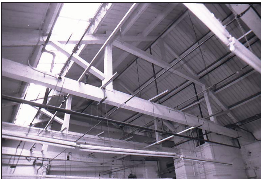
Plate 22: Yeoman Lane Range, 3rd floor roof structure.
