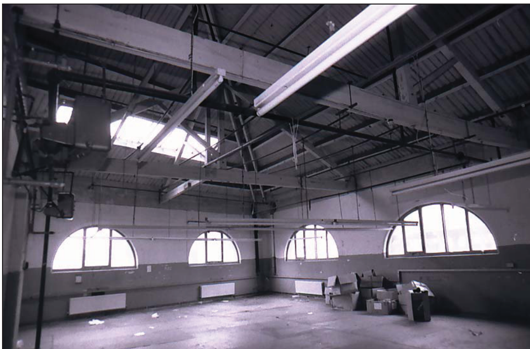
Plate 17: Corner Block, 3rd floor roof structure. Looking northeast.
