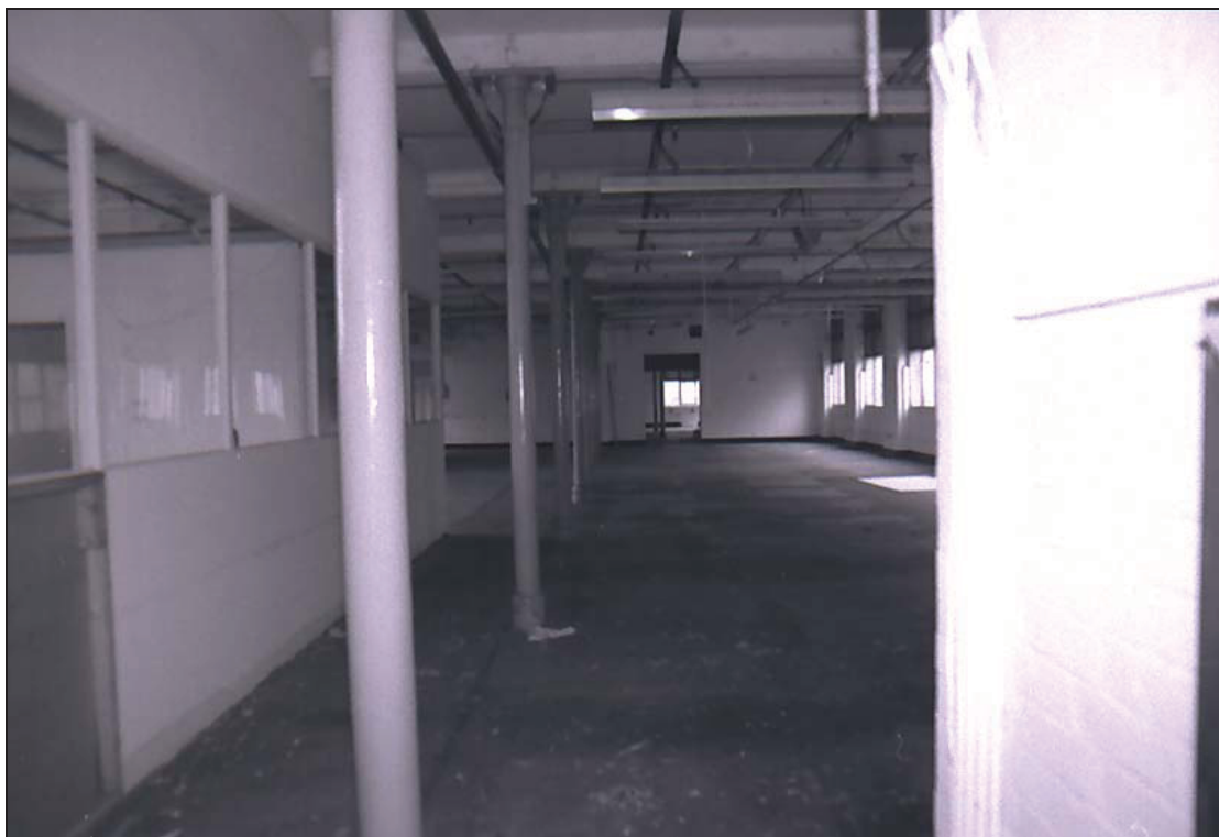
Plate 13: Yeoman Street Range, 2nd floor. Looking north.
