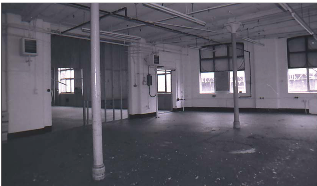
Plate 16: Corner Block, 2nd floor. Looking northwest.
