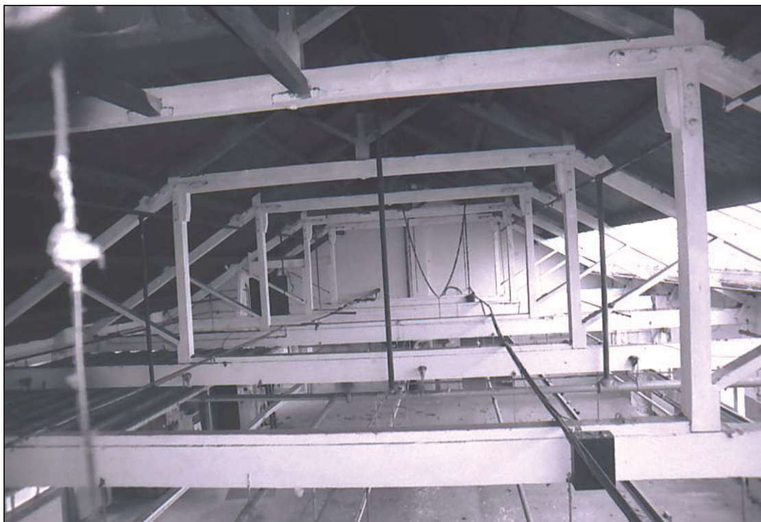
Plate 15: Yeoman Street Range, 3rd floor roof structure. Looking north.
