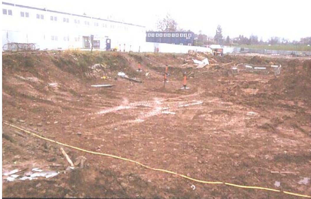
Plate 1 Excavated slope of site looking south west
