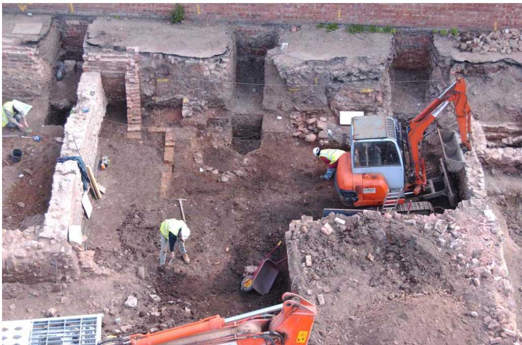
Plate 3: Area 2: machining in progress, viewed northeast
