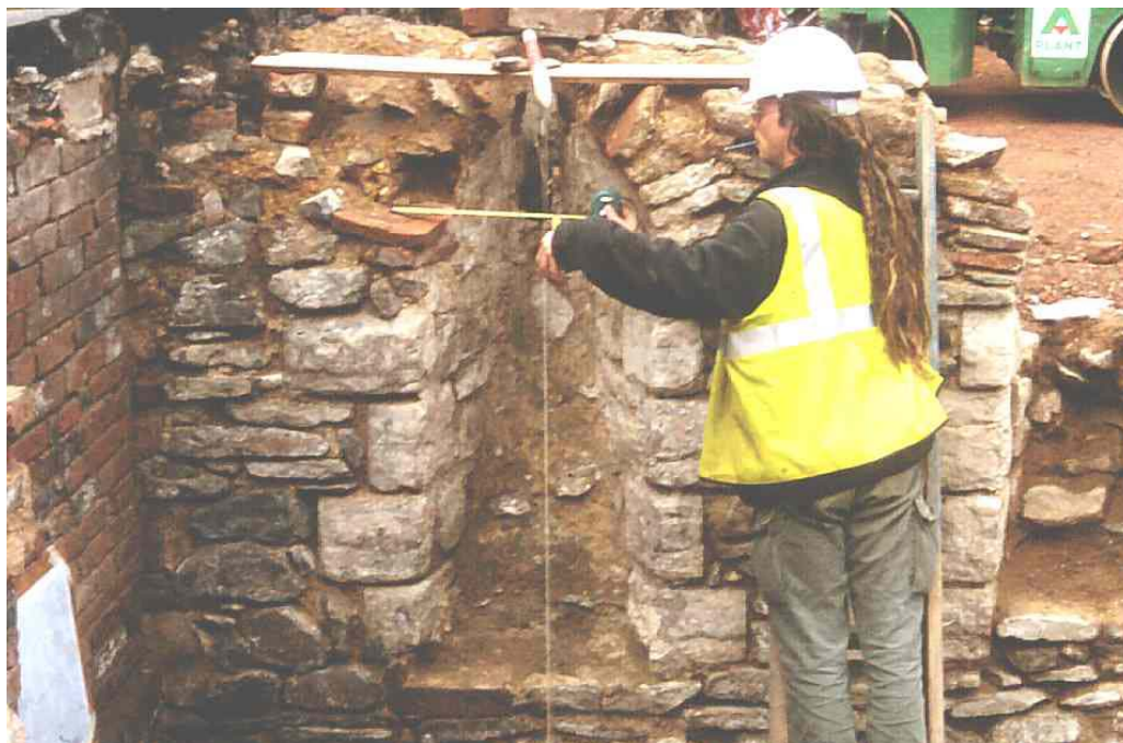
Plate 10: Recording splayed window in the west wall of the undercroft (view south-west)
