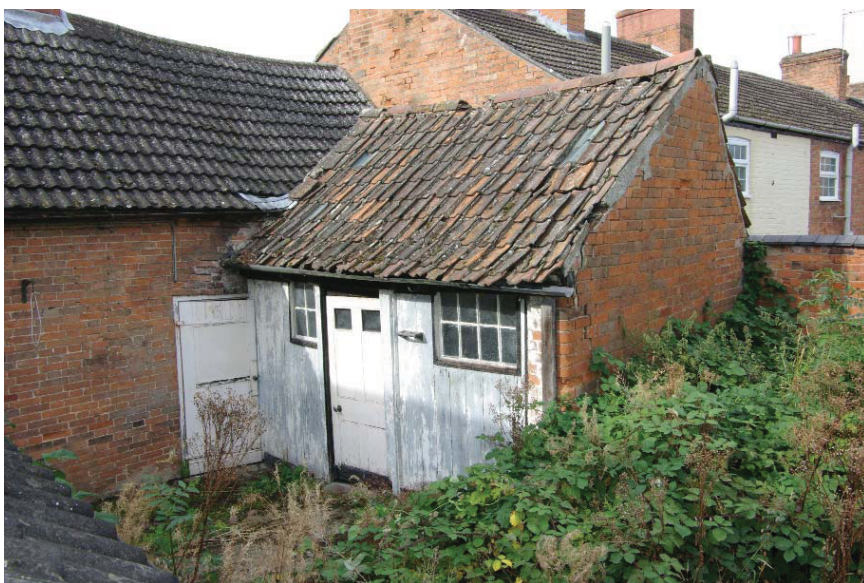
Photo 11. Range D washhouse exterior, looking north-west
