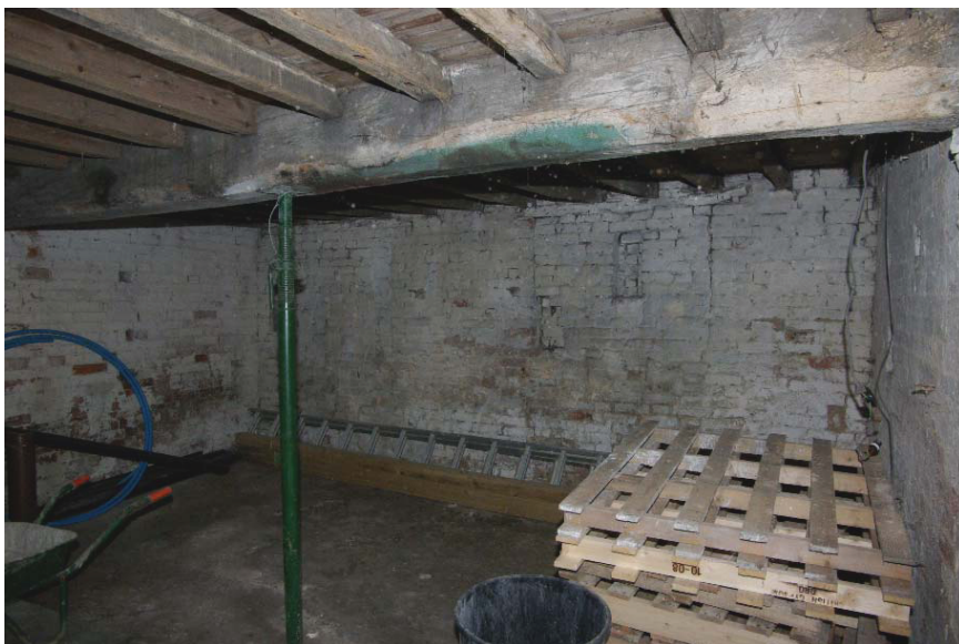
Photo 13. Range E stable-block ground floor interior, looking south-east
