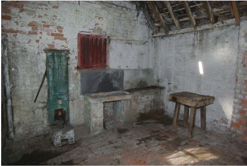
Photo 12. Range D washhouse interior, looking north-west
