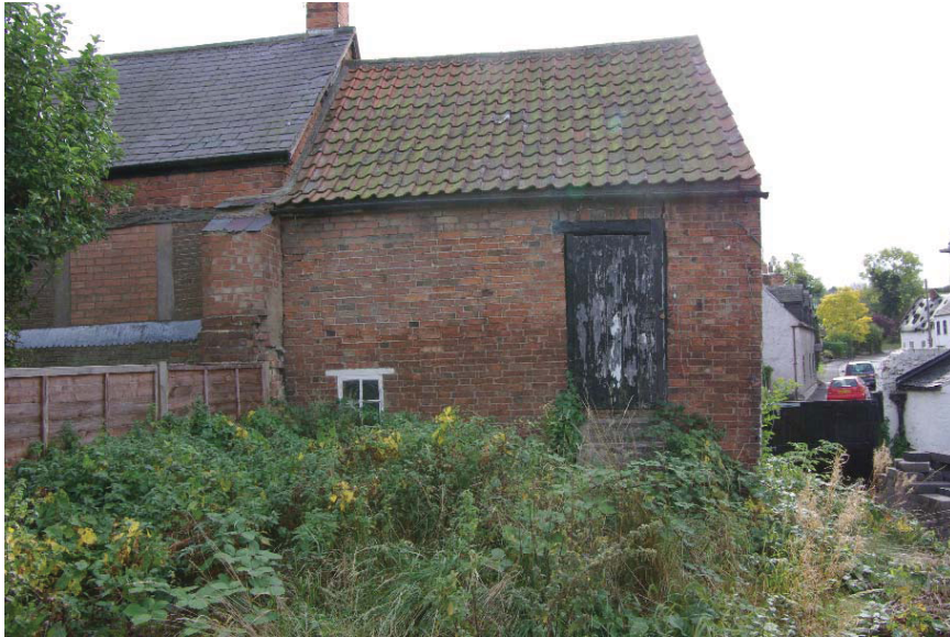
Photo 14. Range E stable-block north elevation and first floor access, looking south
