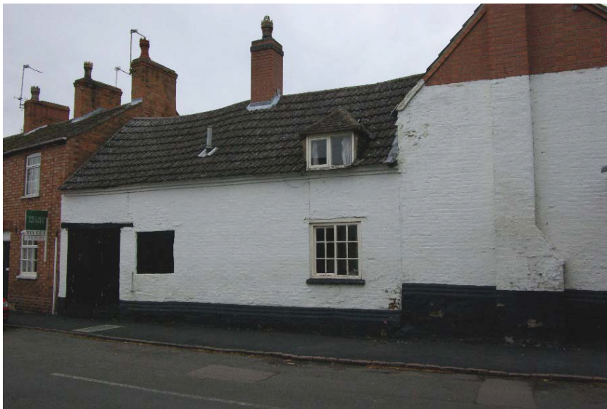
Photo 8. Water Lane elevation of Range B, looking north-east
