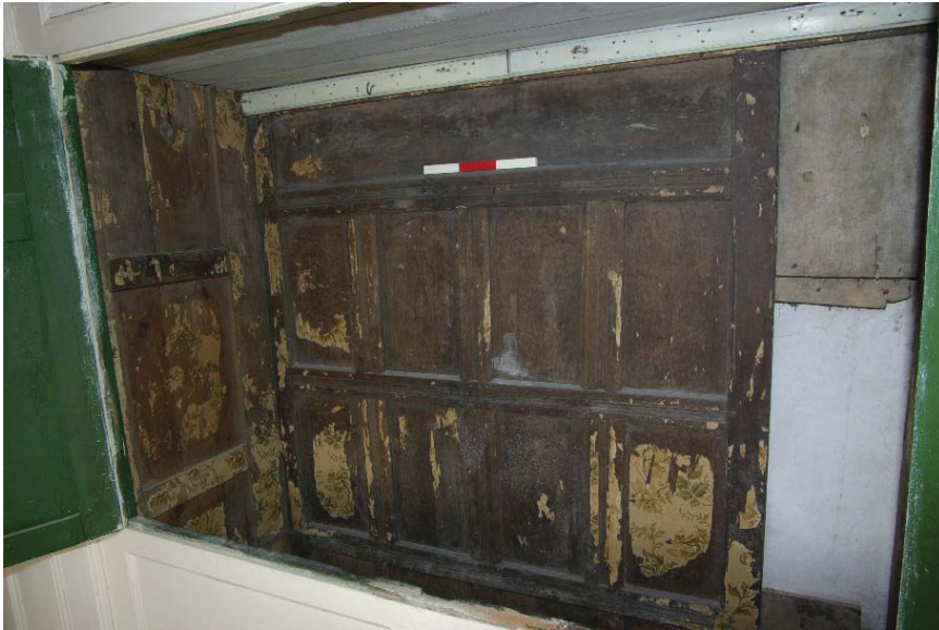
Photo 6. Range A reused panelling in landing cupboard, looking north
