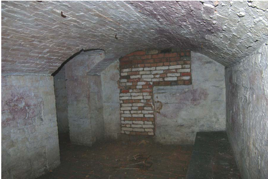
Photo 5. Range A cellar showing blocked original entrance, looking north
