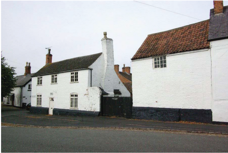
Photo 1. Main Street elevation of Old Star Cottage with former stable-block to right
