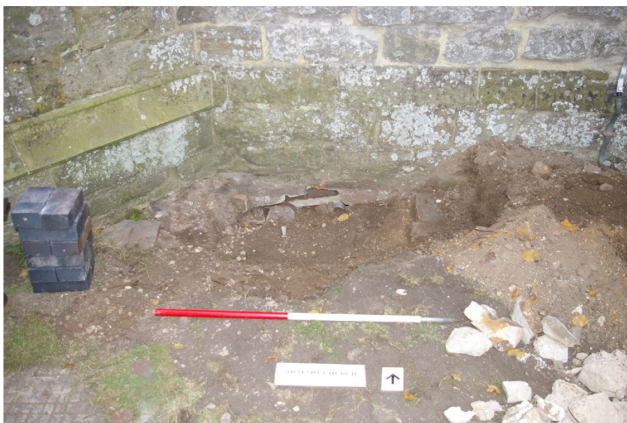
Figure 2 Pipework exiting south wall of west tower.
