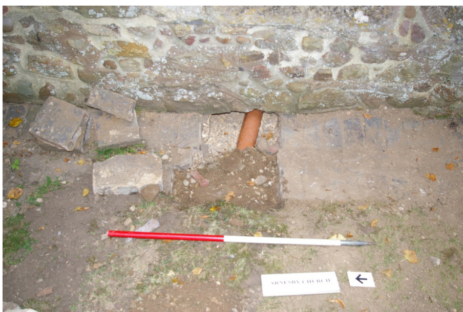
Figure 3 Pipework exiting west wall of south aisle.
