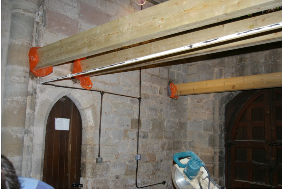
Figure 4 Joist holes in south wall of west tower.
