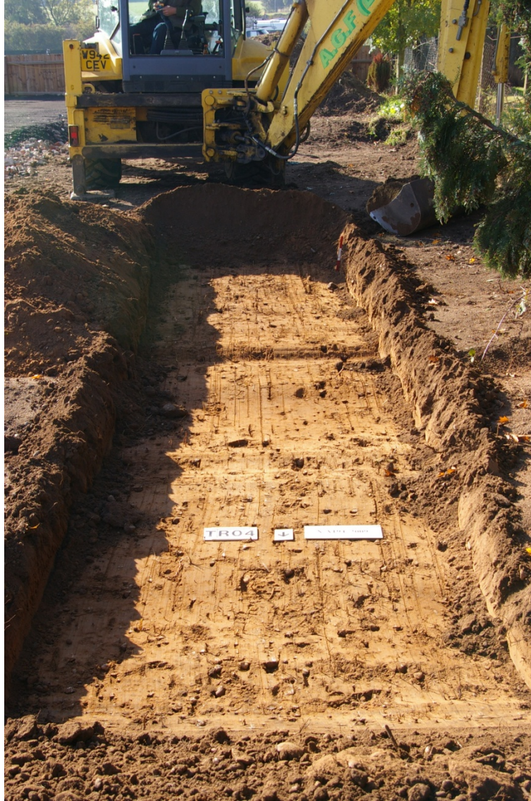
Figure 4 Exposed substratum Within Area 4.
