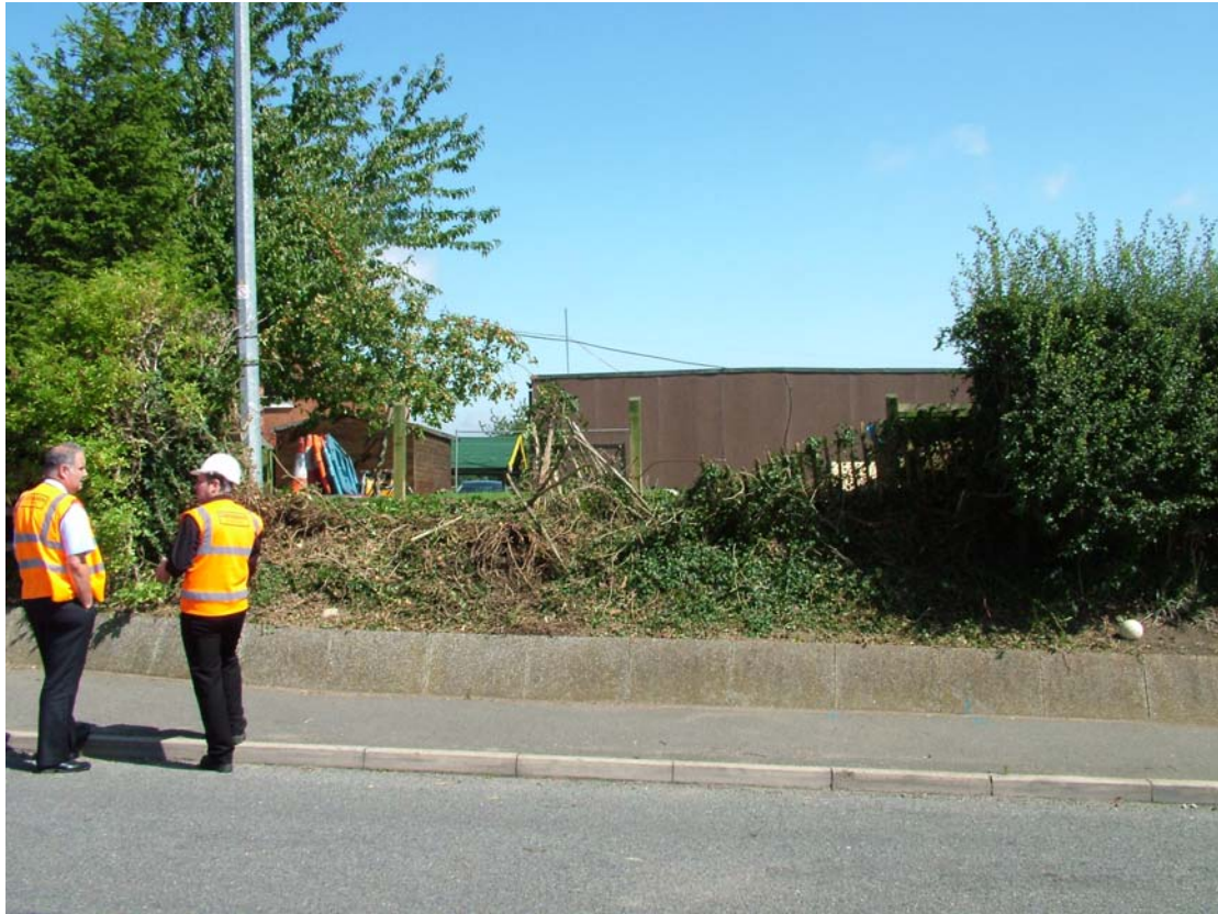
Plate 1: The street frontage after removal of the hedge, looking north-east
