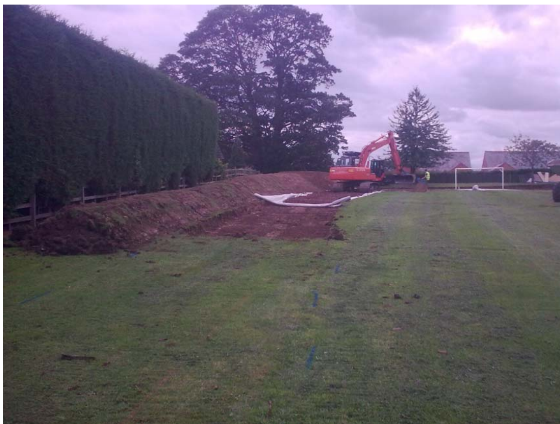
Plate 9: Work in progress on access road
