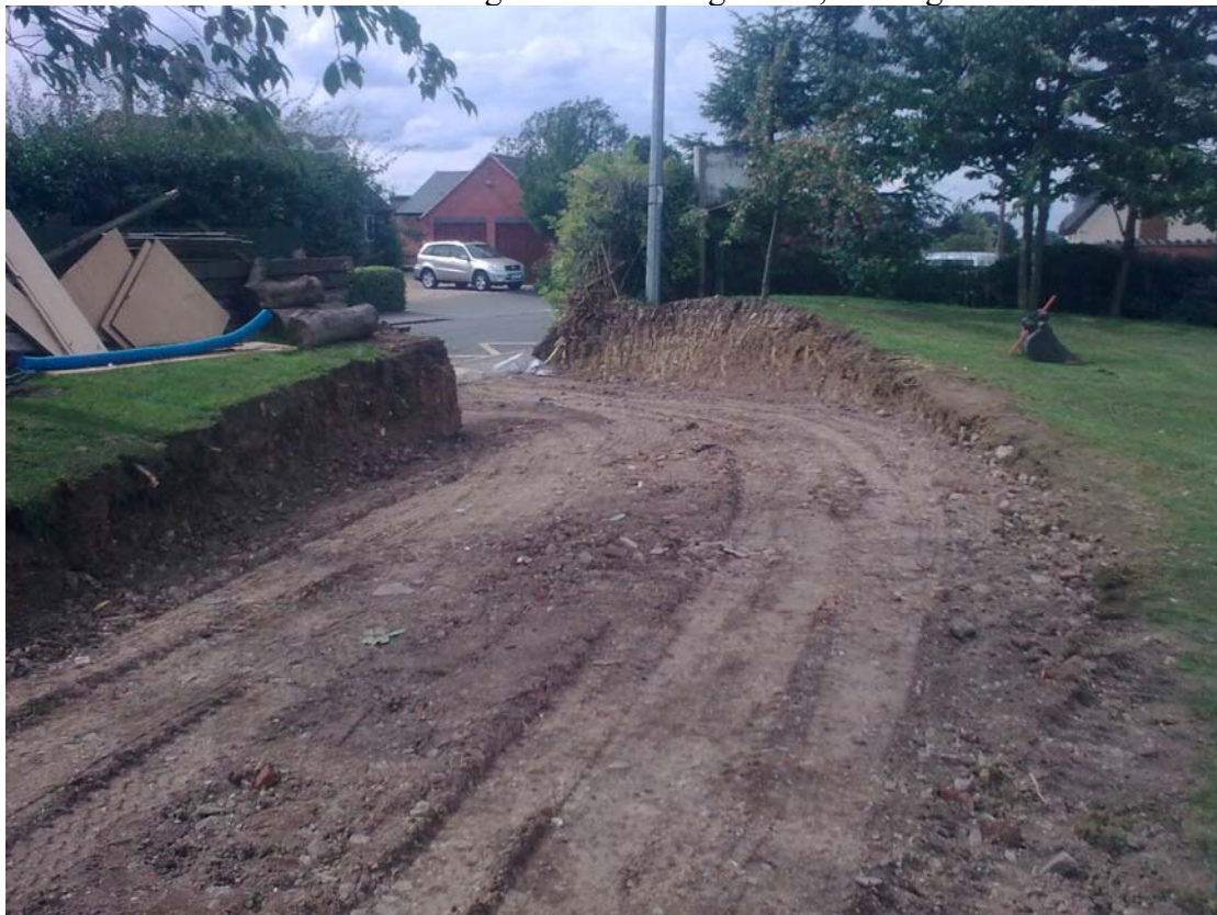
Plate 8: Access road leading from entrance, looking north-west
