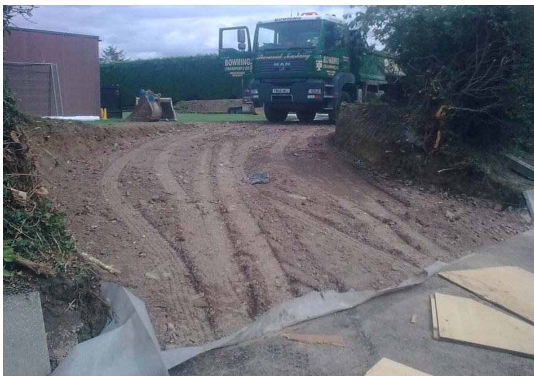
Plate 5: Frontage after removal of bank, looking east
