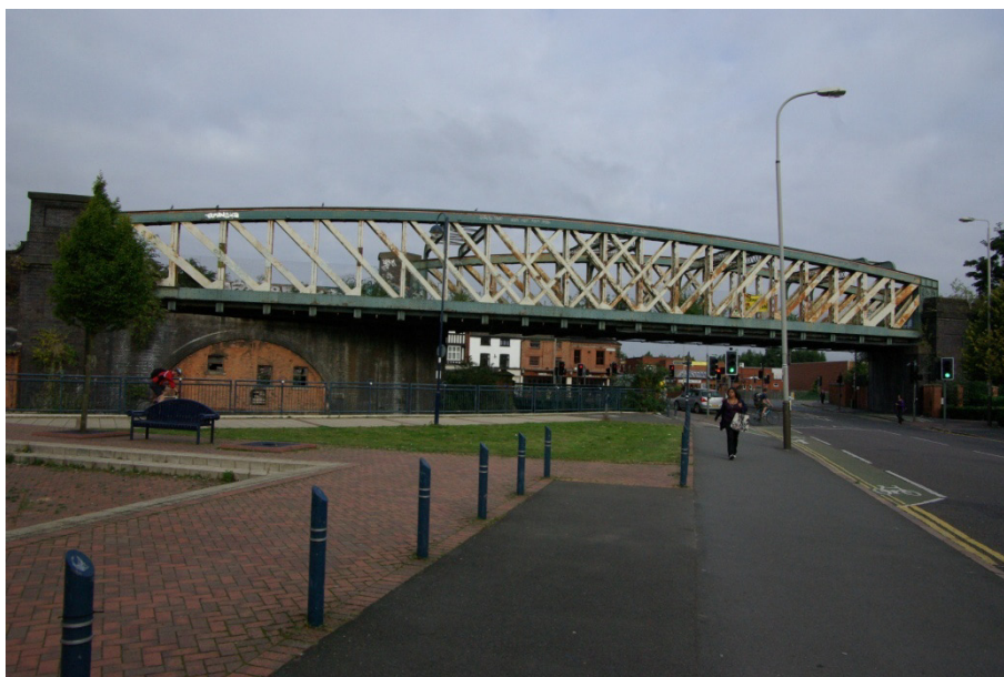
Figure 3 Bridge (Looking West).
