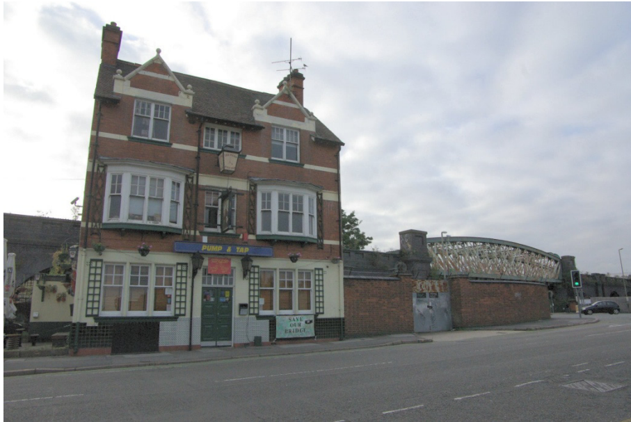
Figure 4 Pump & Tap with the Bridge in the Background.
