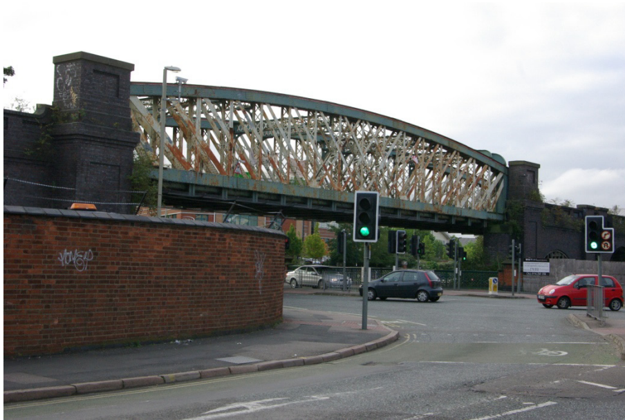
Figure 2 Bridge (Looking South East).
