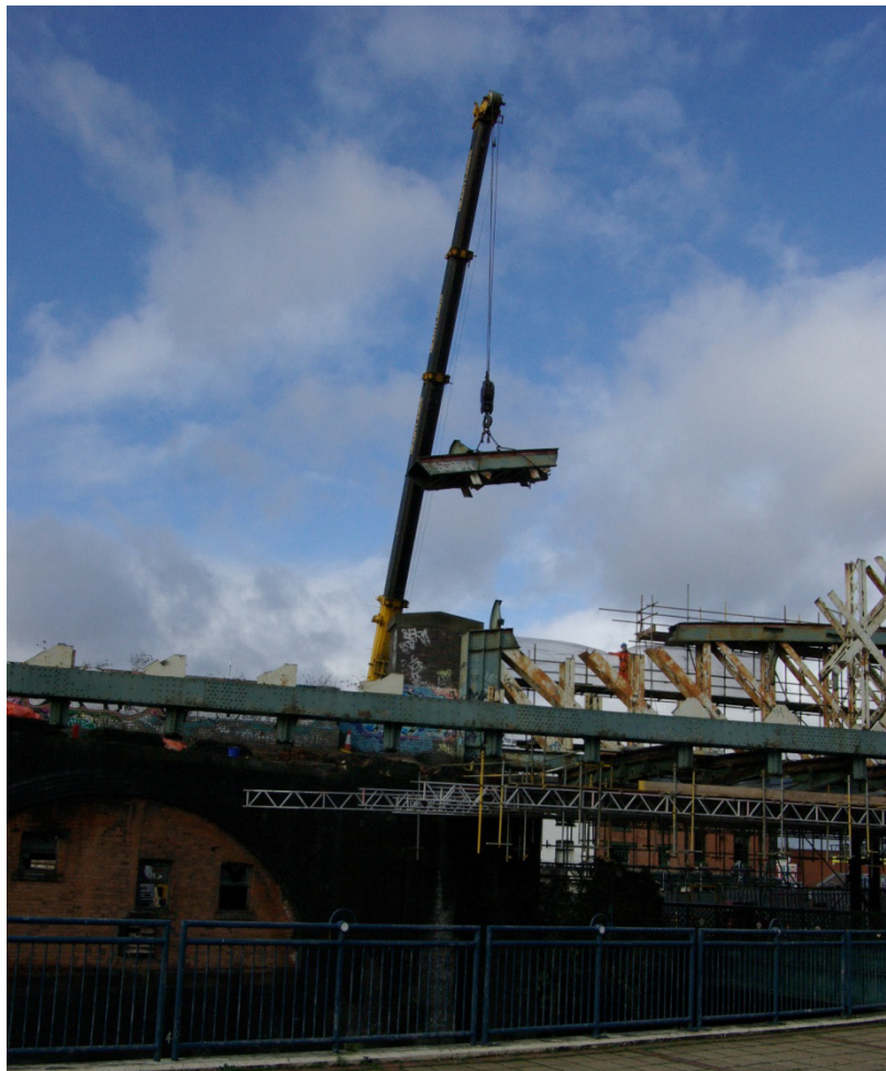
Figure 7 Dismantling in Progress.
