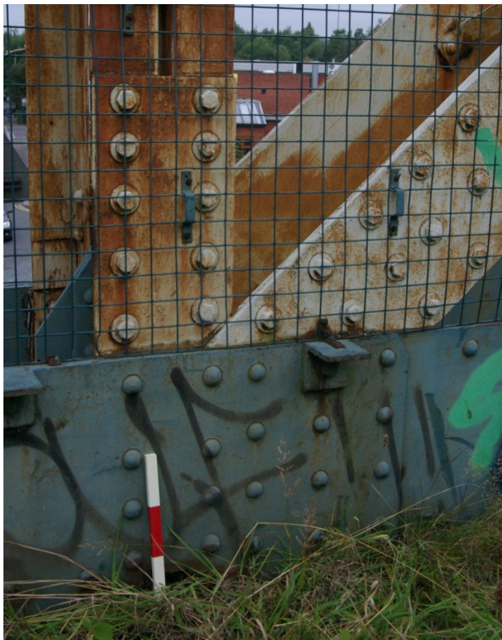
Figure 5 Bolted Strengthening Plates.
