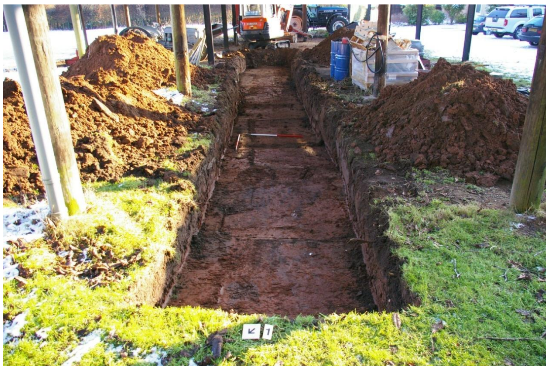
Figure 7 Trench 01 Looking south-east. 2 x 1m scales Note that apparent dark feature near to scale is a shadow cast by the barn posts.
