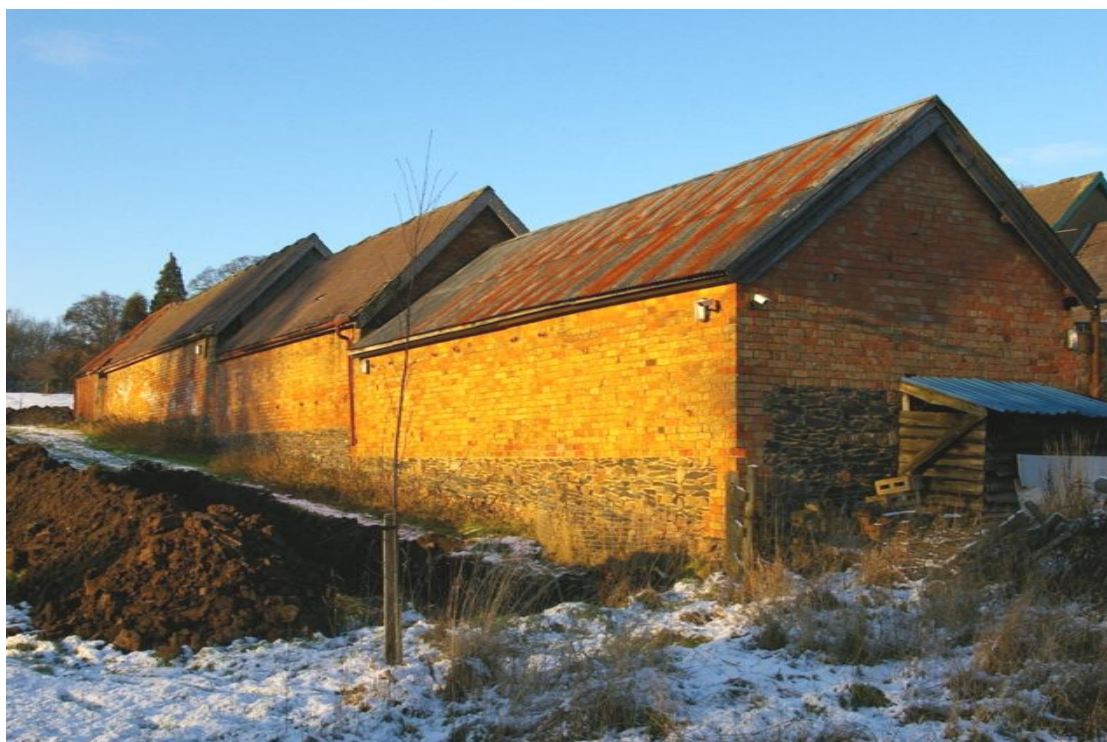
Figure 10 Trench 03 location Looking north
