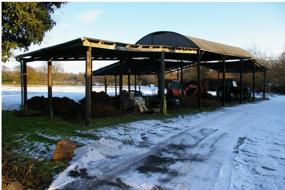
Figure 6 Trench 01 location within barn Looking south-east
