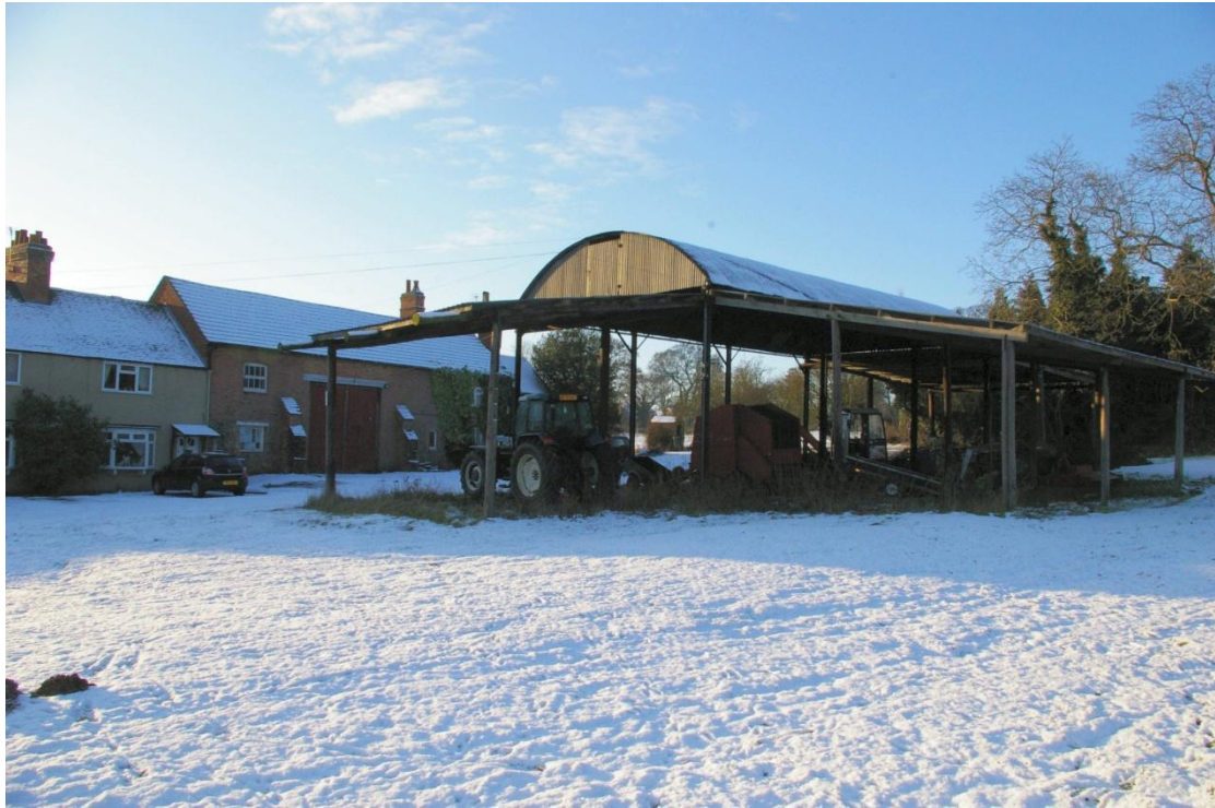
Figure 4 Farm buildings and Dutch barn Looking north-west
