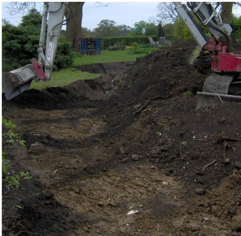
Figure 4: Removal of the topsoil and subsoil
