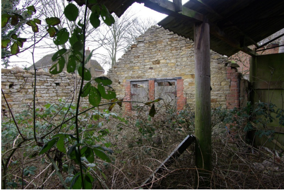
Figure 7 Southern Gable Wall of Building 3 (Looking South East).
