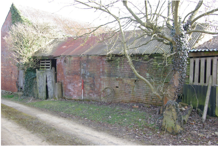
Figure 5 Building 2 (Looking North East).
