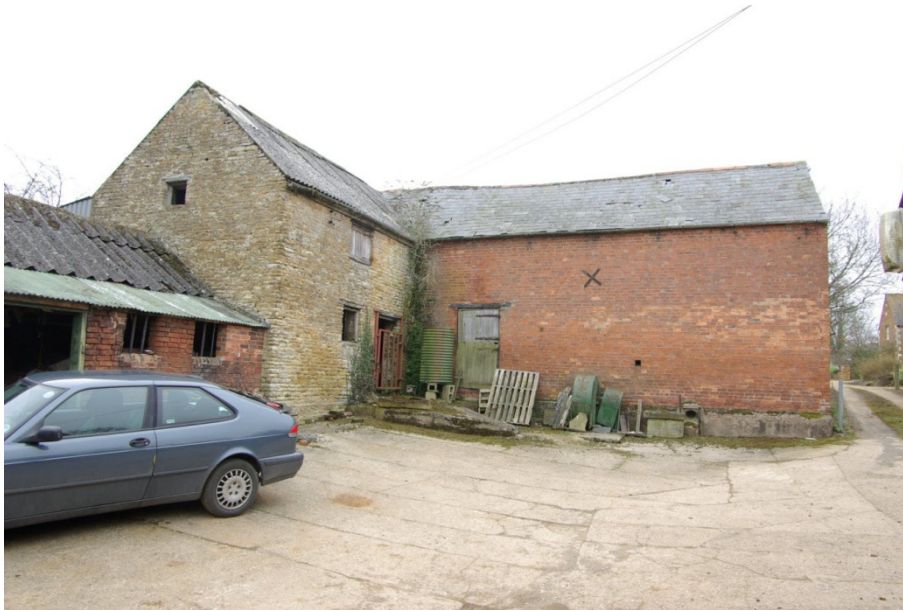
Figure 3 Buildings 1 & 3 (Looking South East).
