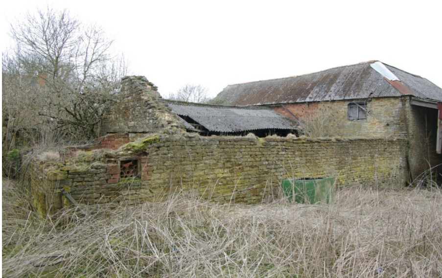
Figure 4 General View (Looking North West).
