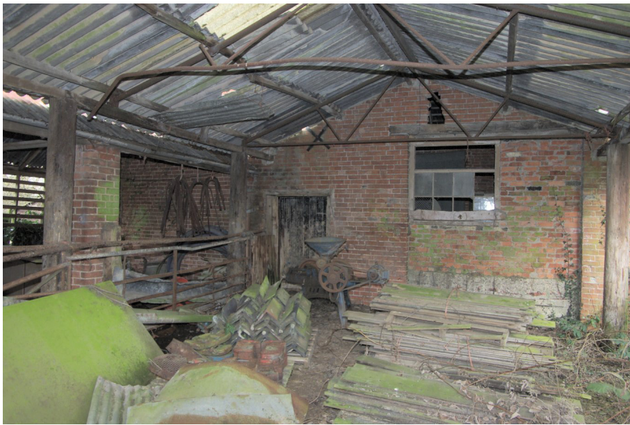
Figure 6 South Facing Elevation of Building 1 & Roof Trusses of Building 4.
