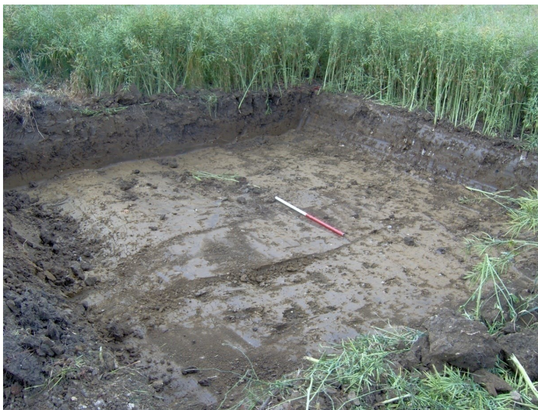
Figure 3: The Turbine footing stripped down to natural clay. Looking west.
