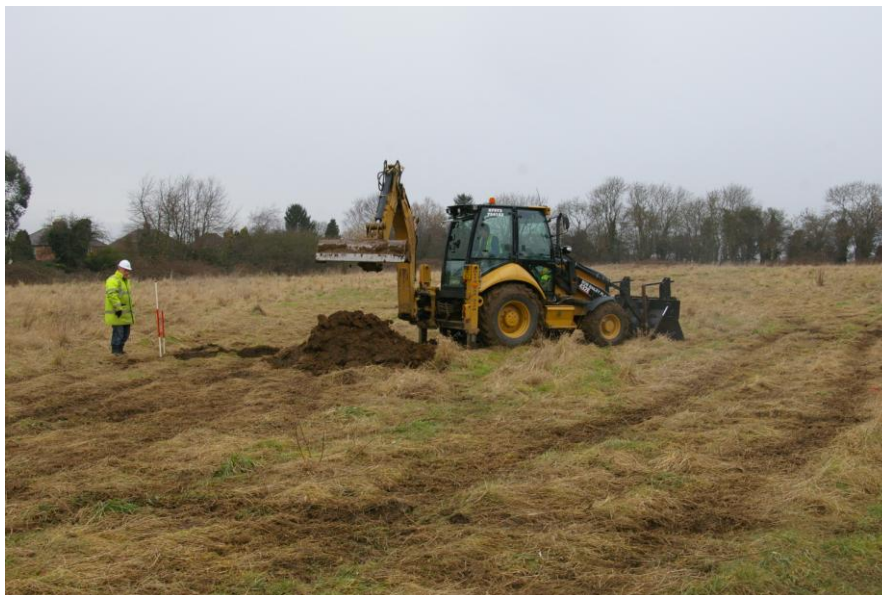
Figure 5: Machining in progress, Area 1: view looking north
