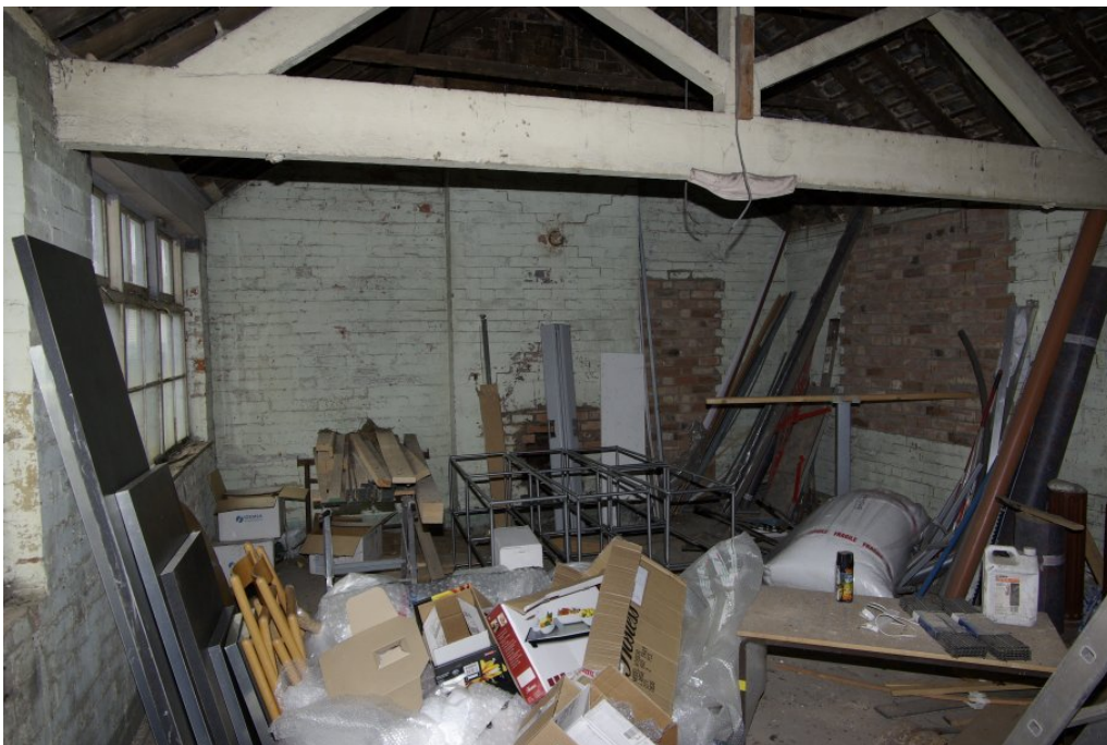
Plate 6 General view of interior, Building B, first floor.
