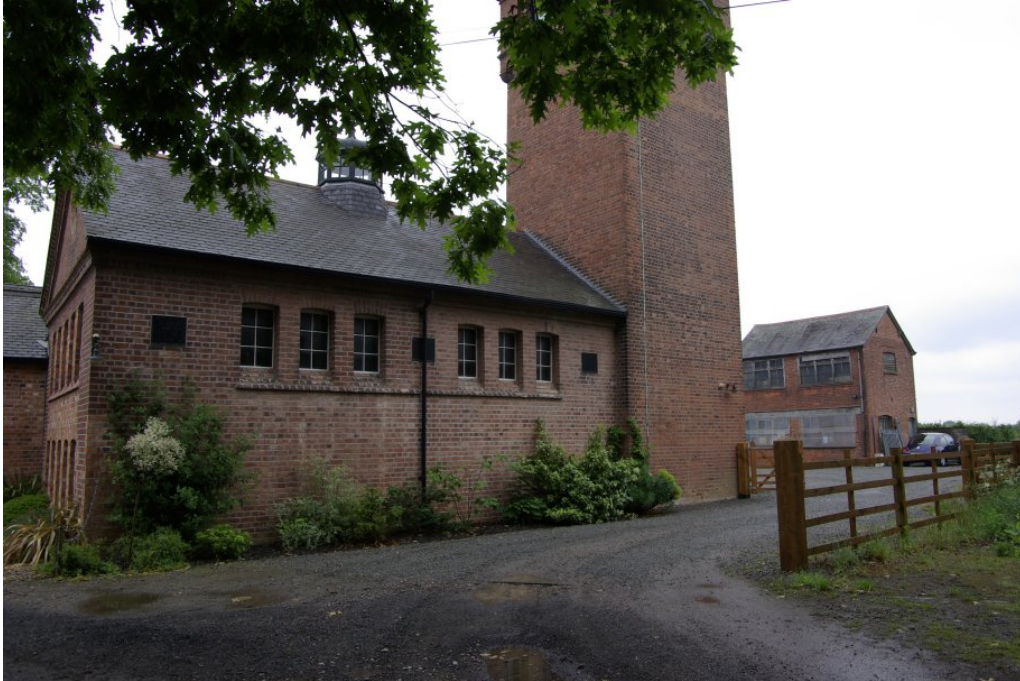
Plate 1 Water Tower with Building A to the right.
