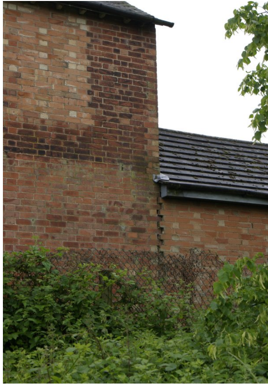
Plate 5 Northern elevation showing blocked window, evidence of lean-to & new brickwork.
