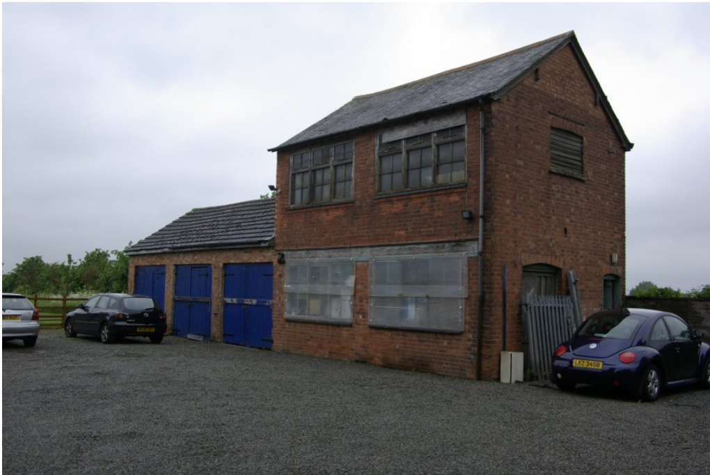
Plate 2 Buildings A (left) and B (right) looking north-west.
