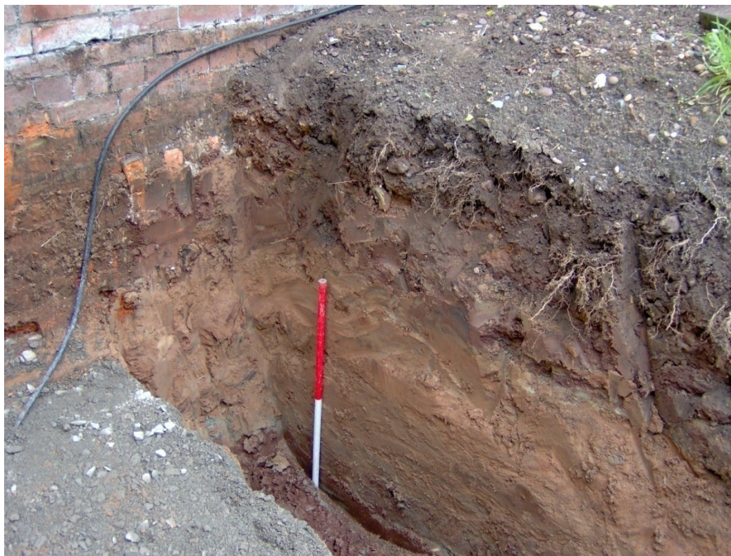
Figure 3: South-east facing section in retaining wall footing, looking west
