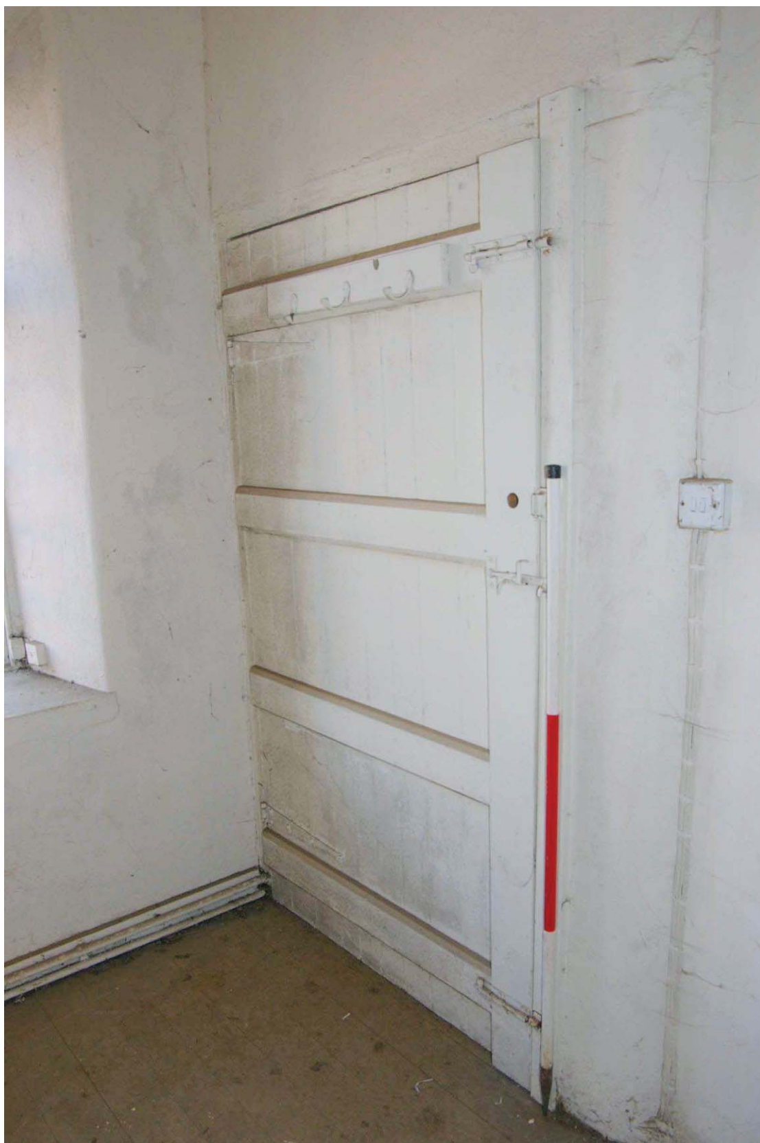
Figure 27 Top of stairs, first floor door detail Looking east, 1.5m scale
