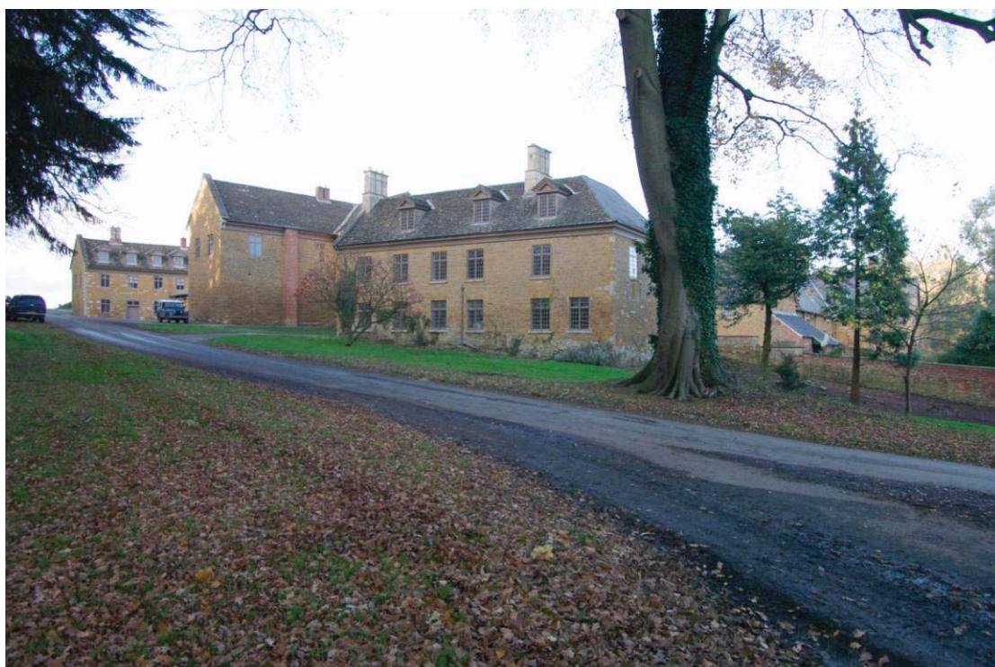
Figure 5 Laundry building and Main Stables Looking north
