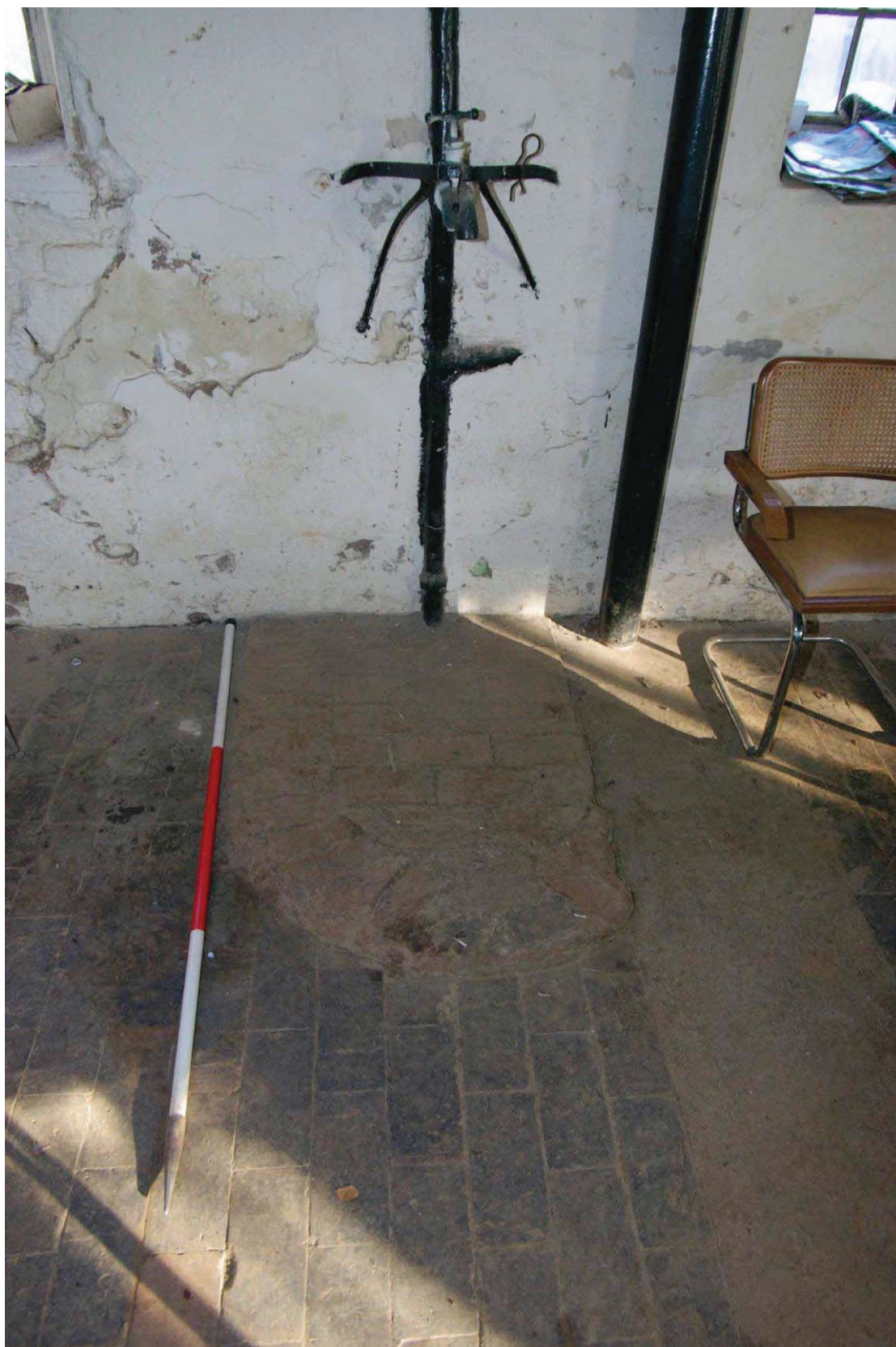
Figure 20 Ground floor, truncated brick base below tap Looking north-east. 1.5m scale
