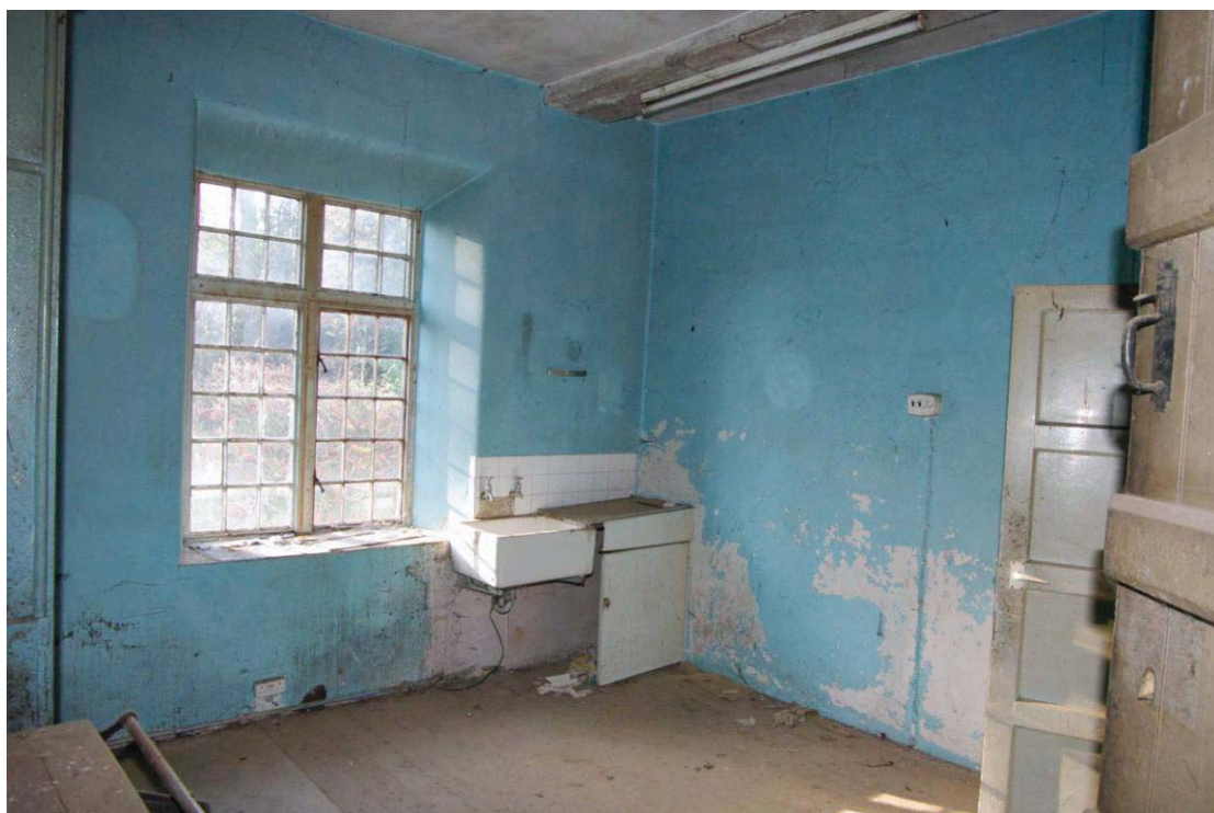
Figure 35 First floor, east end kitchen Looking west
