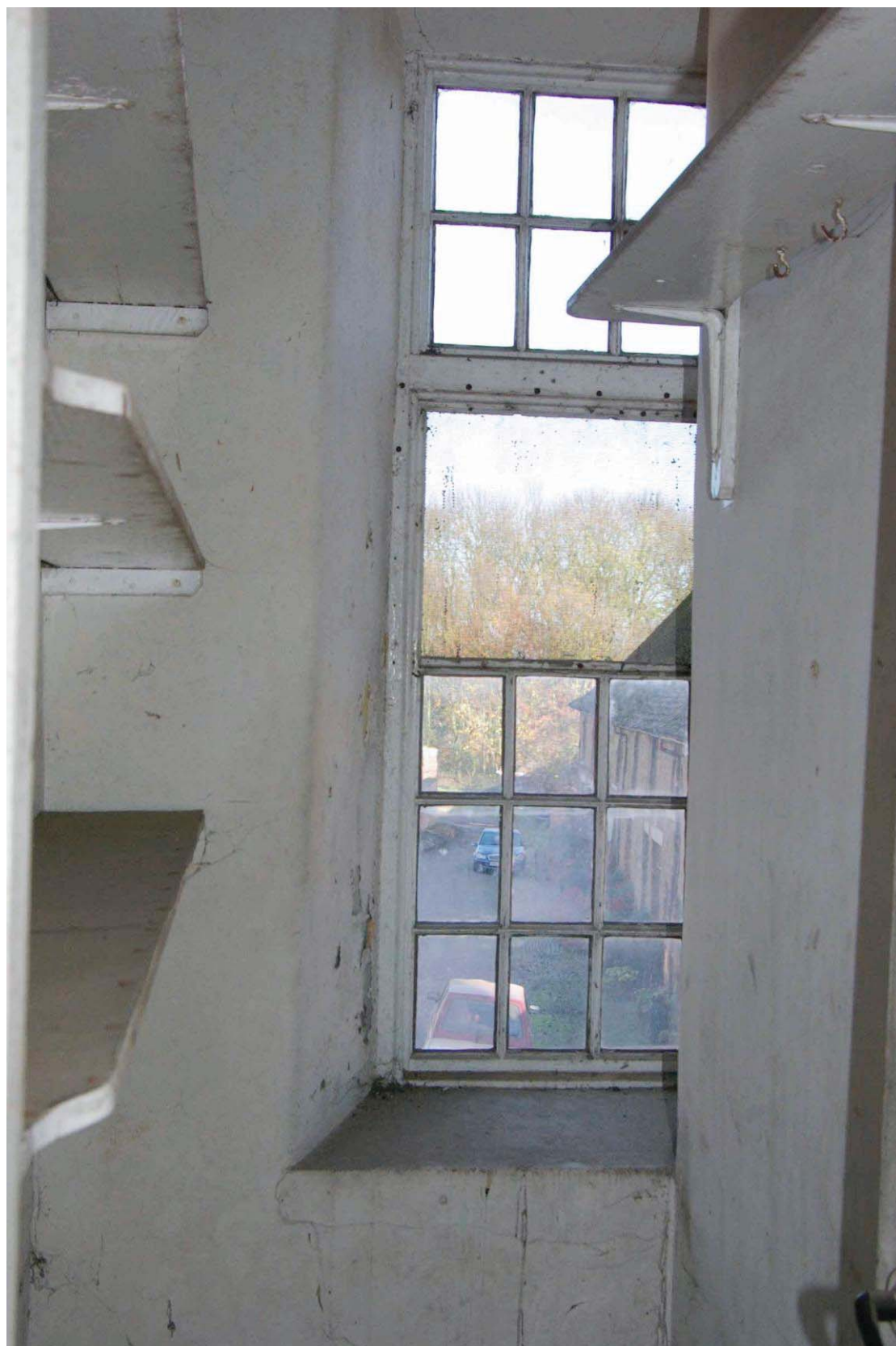
Figure 29 First floor, store room showing inserted wall across window Looking north-east
