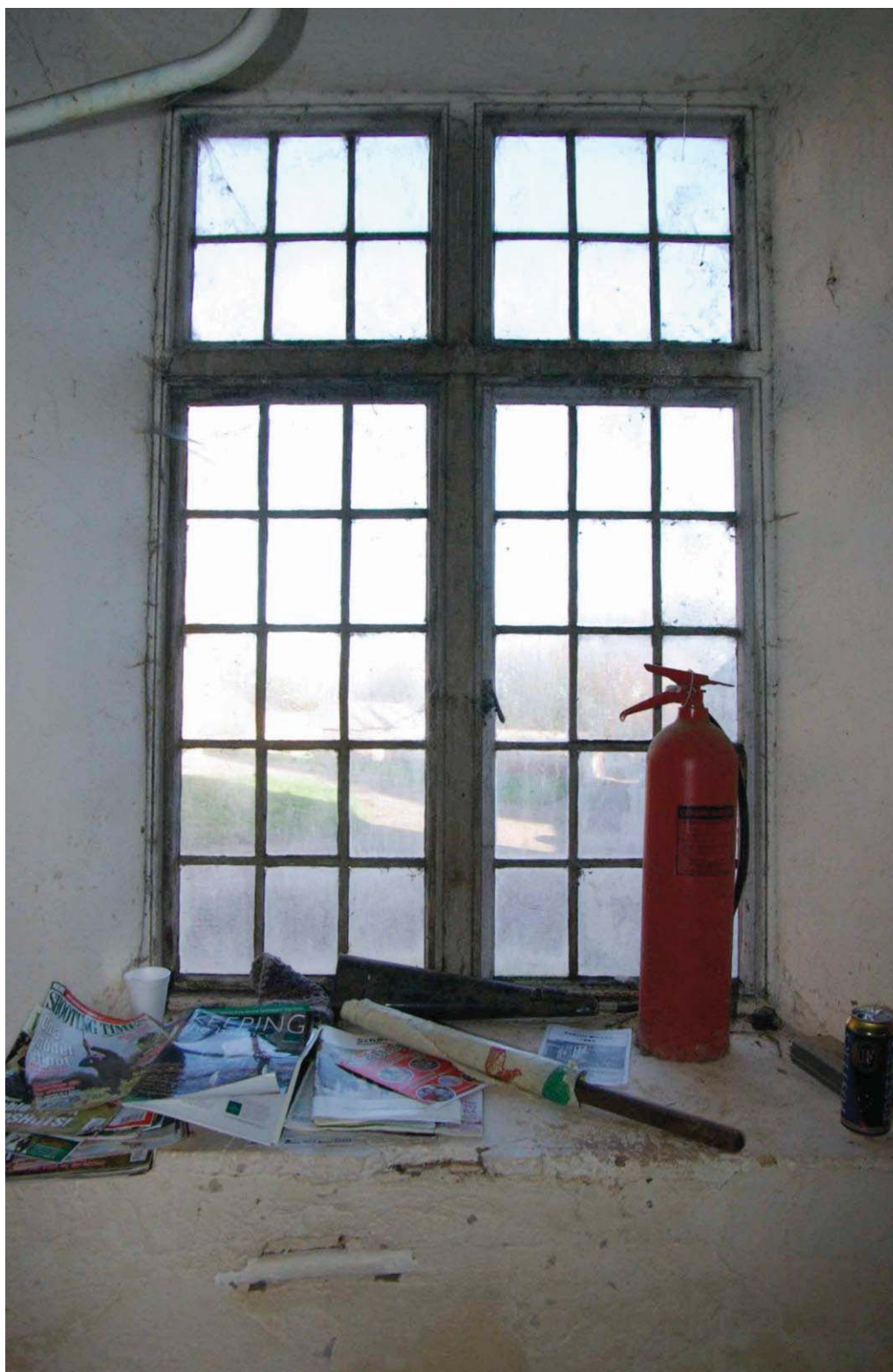
Figure 16 Ground floor window detail Looking south-west
