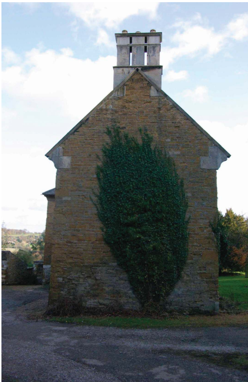
Figure 8 North-west gable end elevation Looking south-east
