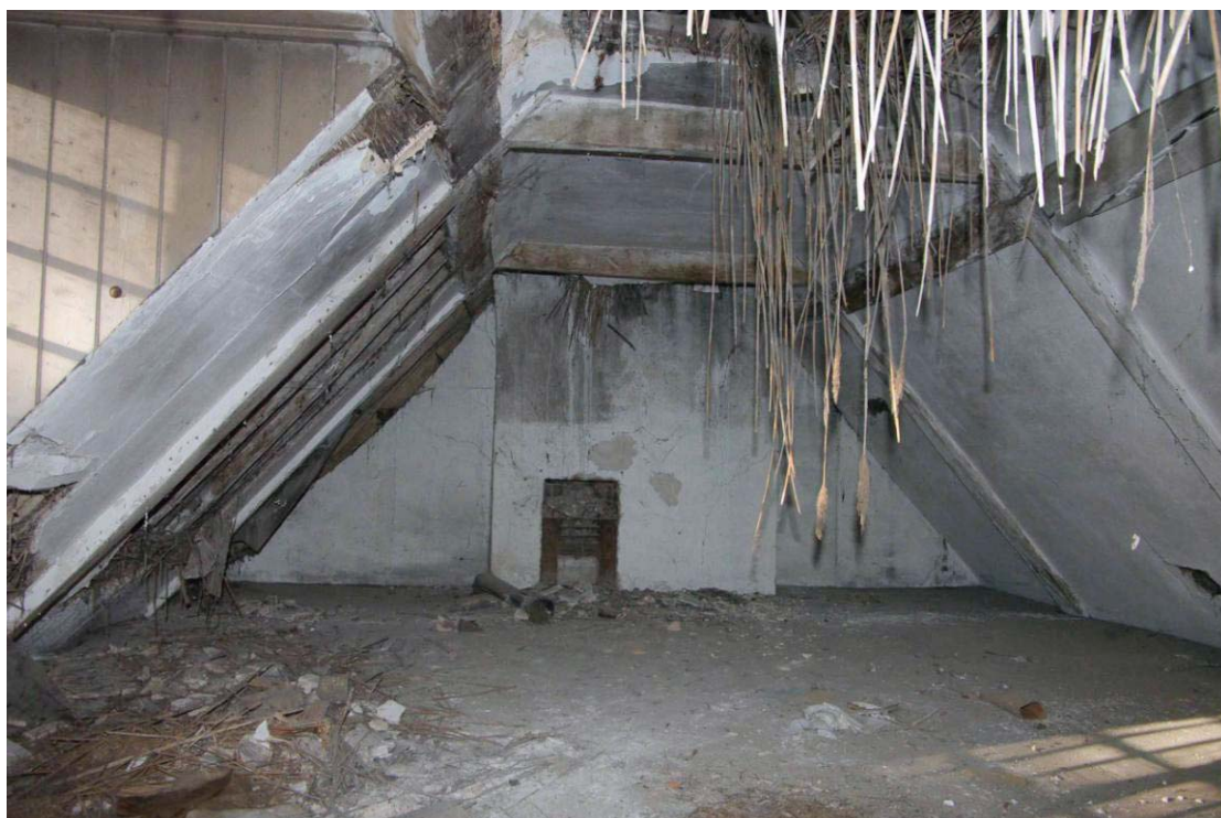
Figure 41 Second floor, west room Looking north-west
