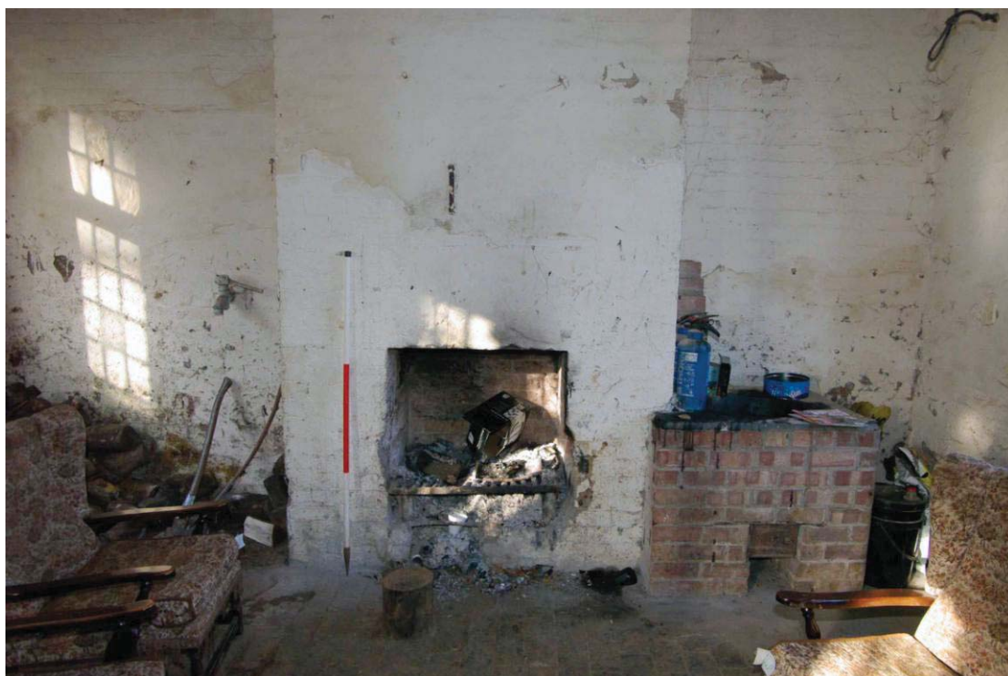
Figure 13 Ground floor fireplace and copper Looking north-west. 1.5m scale
