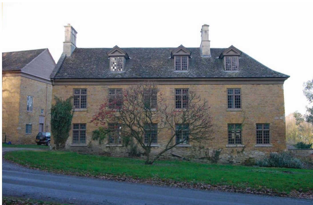
Figure 6 South-west elevation Looking north-east
