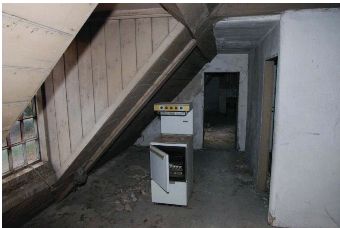
Figure 40 Second floor, corridor to west room Looking north-west
