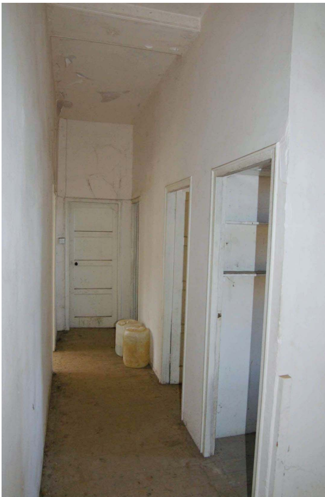
Figure 28 First floor corridor and inserted walls Looking north-west
