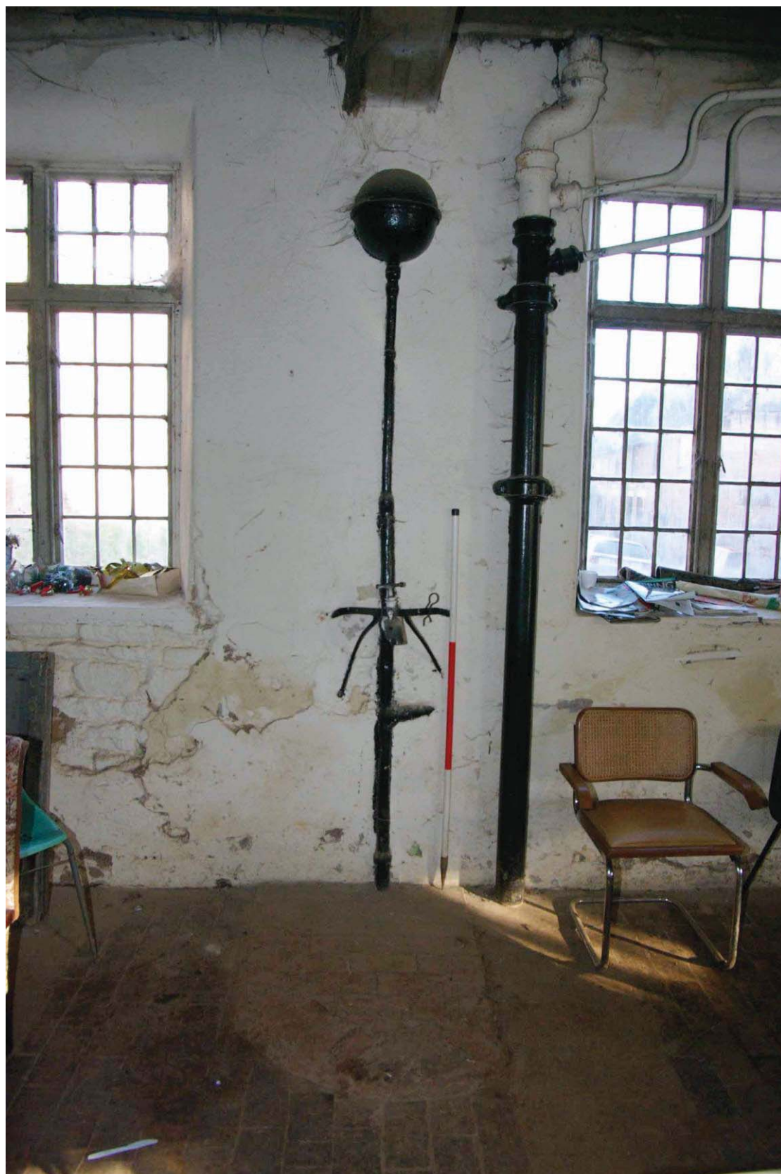
Figure 18 Ground floor, tap and cistern Looking north-east. 1.5m scale
