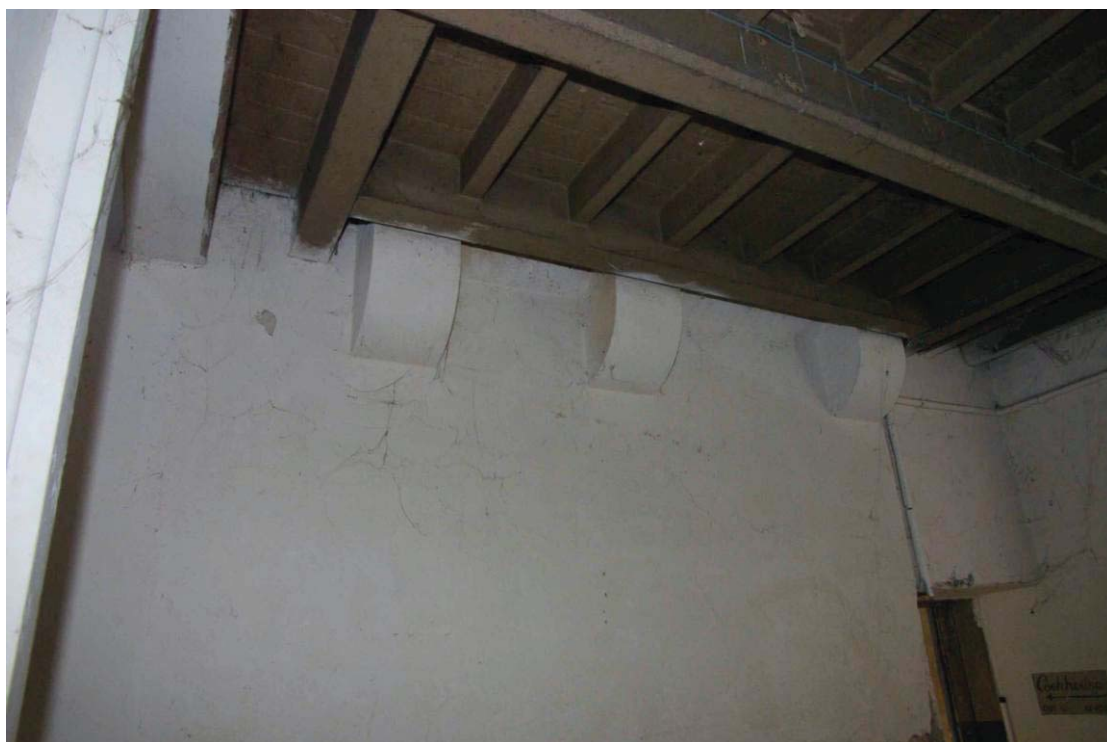
Figure 23 Ground floor, corbels on east wall Looking south
