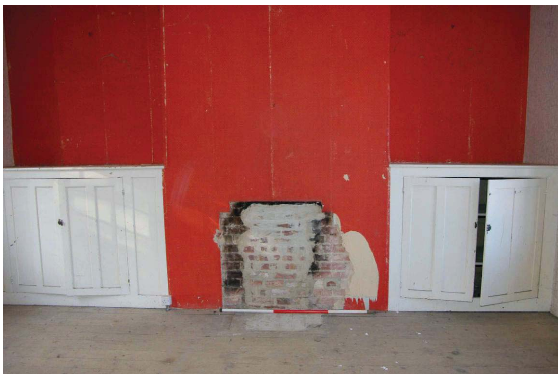
Figure 33 First floor, west bedroom fireplace Looking north-west, 1.5m scale
