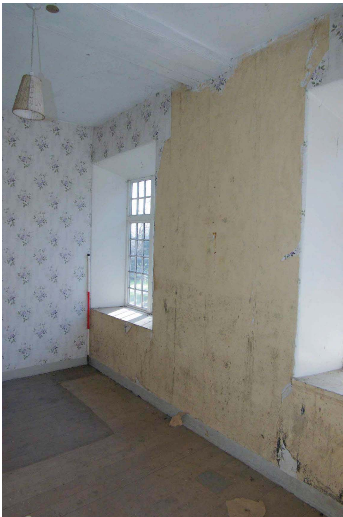
Figure 30 First floor, south bedroom Facing south-east, 1.5m scale
