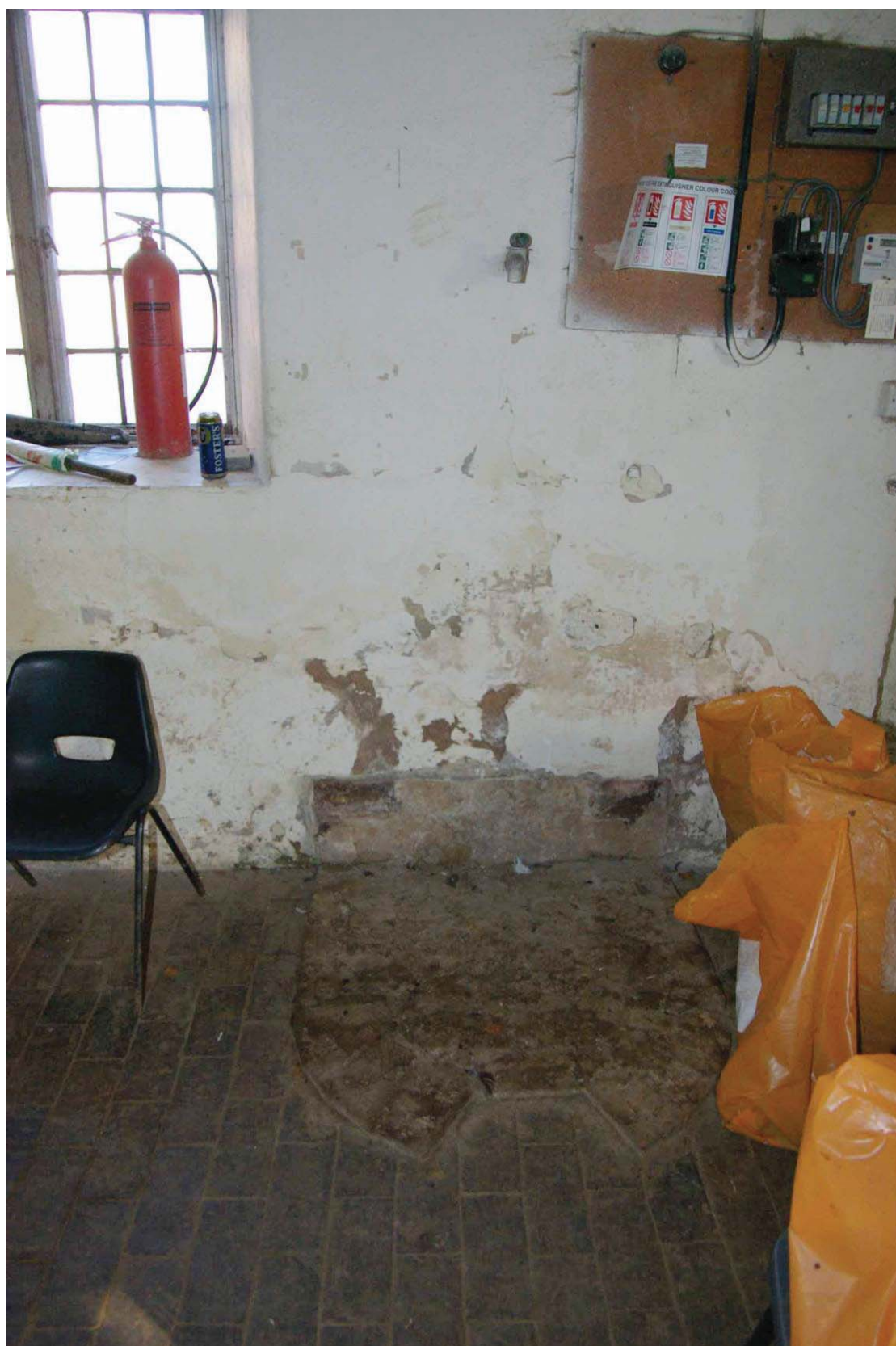
Figure 21 Ground floor, stone base and tap Looking north-east
