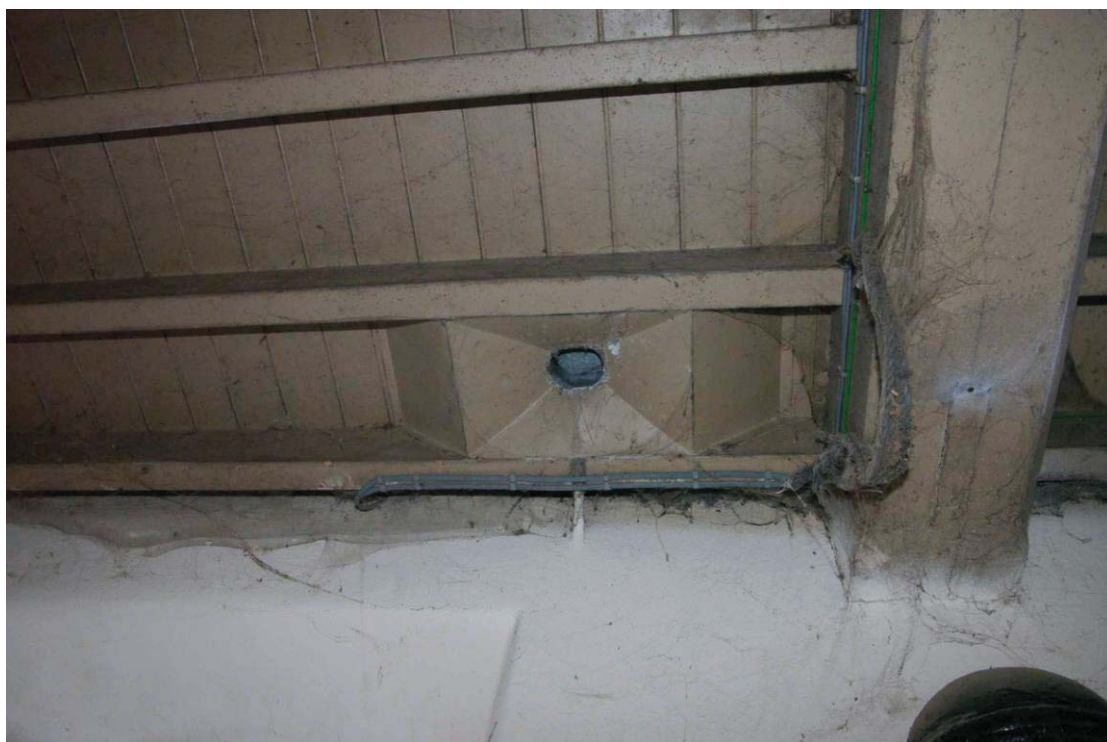
Figure 11 Ground floor ceiling detail Looking north-east
