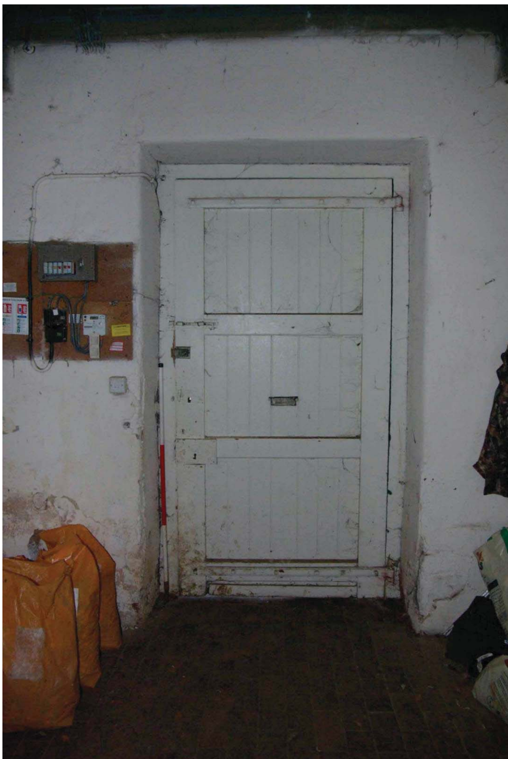
Figure 17 Internal detail of ground floor door Looking north-east. 1.5m scale
