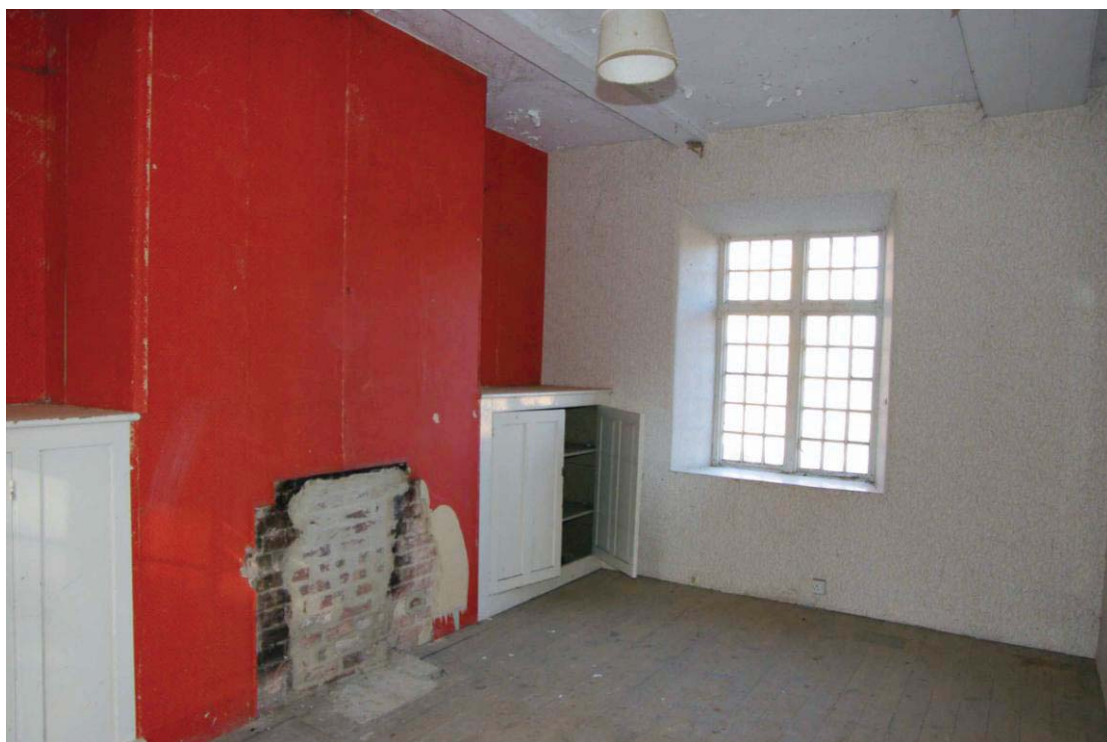
Figure 31 First floor, west bedroom Looking north
