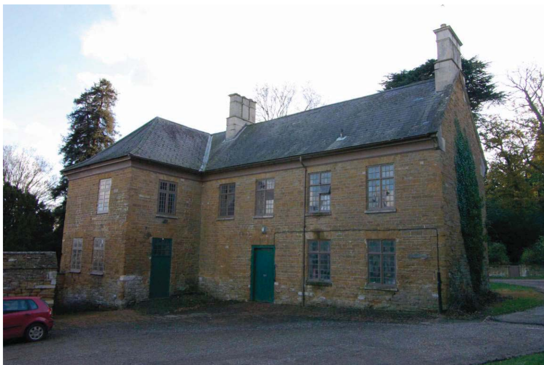
Figure 4 North-eastern elevation of Laundry Looking south
