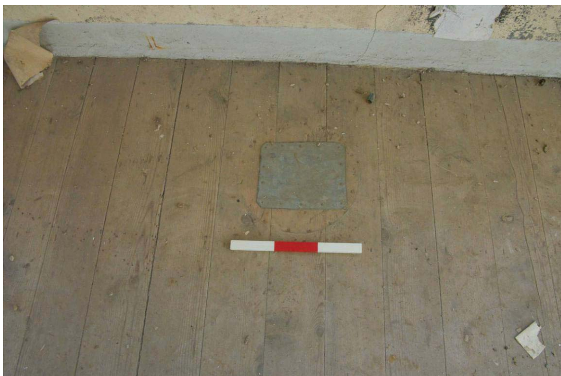
Figure 12 Blanked over feature on first floor 30cm scale
