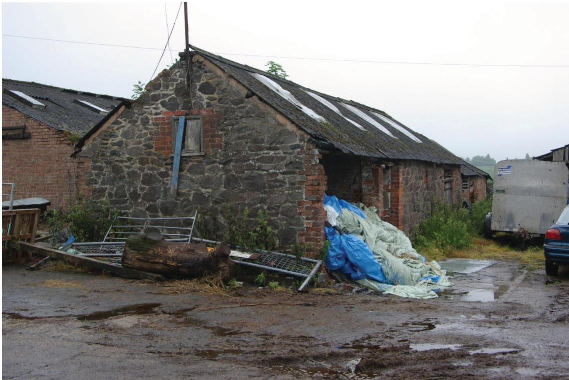
Colour Plate 2 Building 2 (looking east-north-east).
