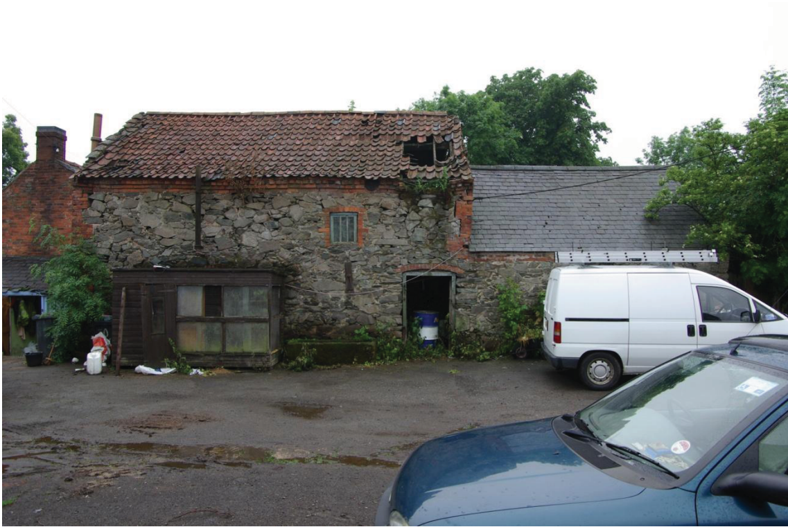
Colour Plate 1 Building 1 (looking south).
