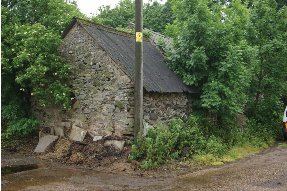
Colour Plate 3 Building 3 (looking south).
