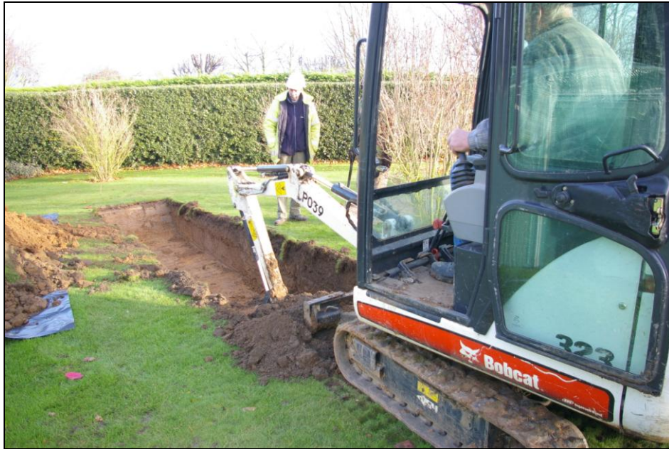
Figure 5: Machining of Trench 3 in progress
