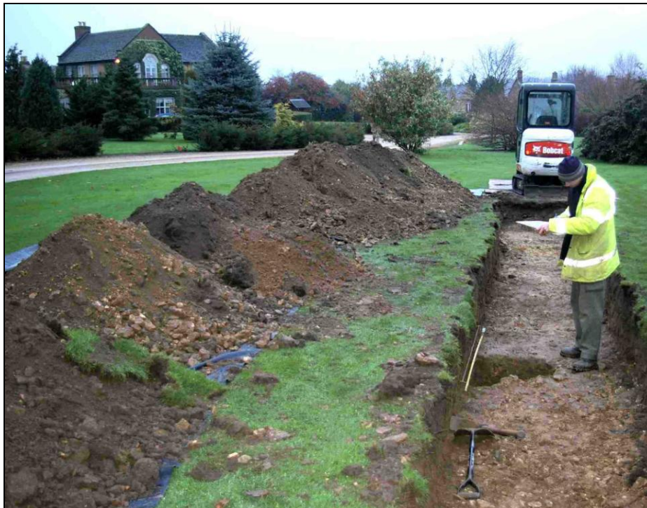
Figure 6: Work in progress on Trench 2
