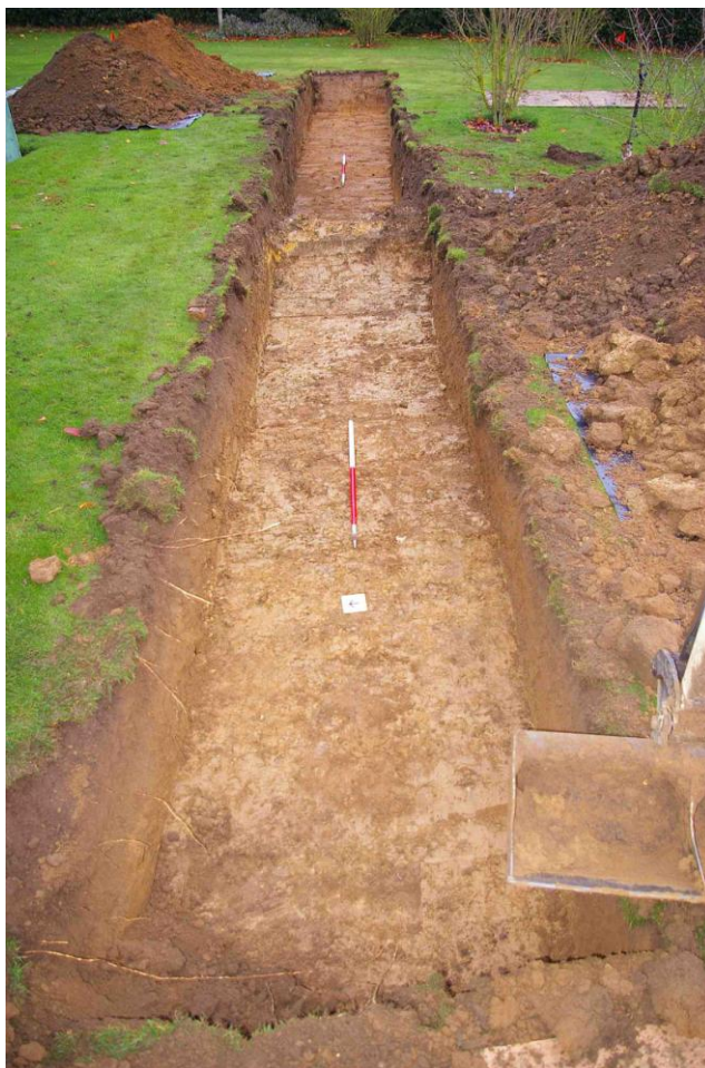
Figure 12: Trench 3: view south-west (1m & 1.5m scales)
