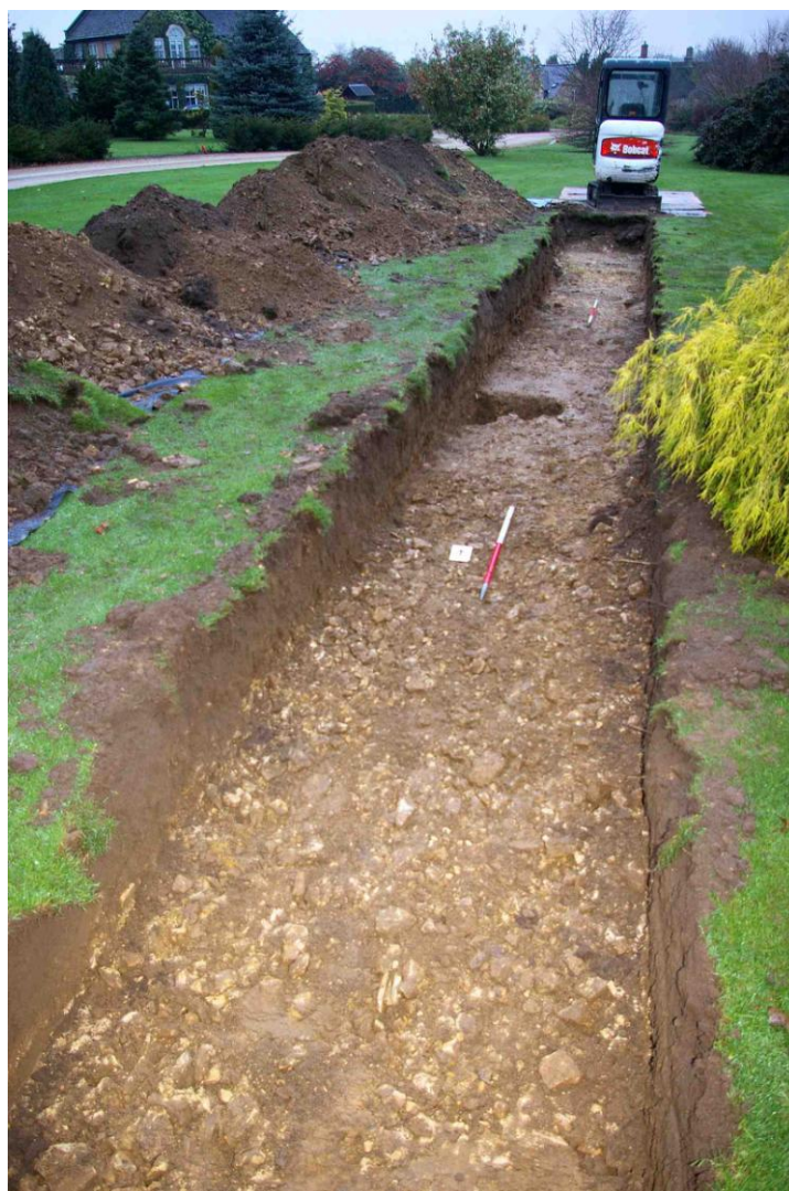
Figure 10: Trench 2: view looking north-west (1m & 1.5m scales)
