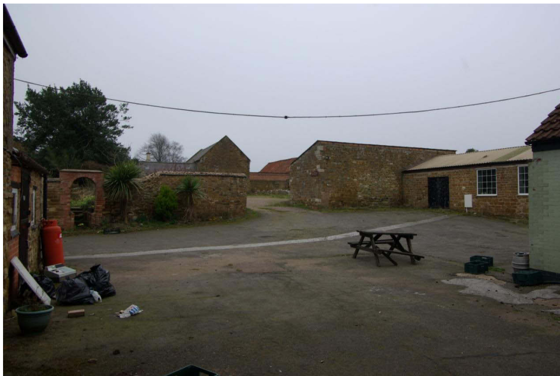
Figure 4 Courtyard and upper car park before development Lean-to stone barn and curving stone wall shown before demolition. Looking SW.
