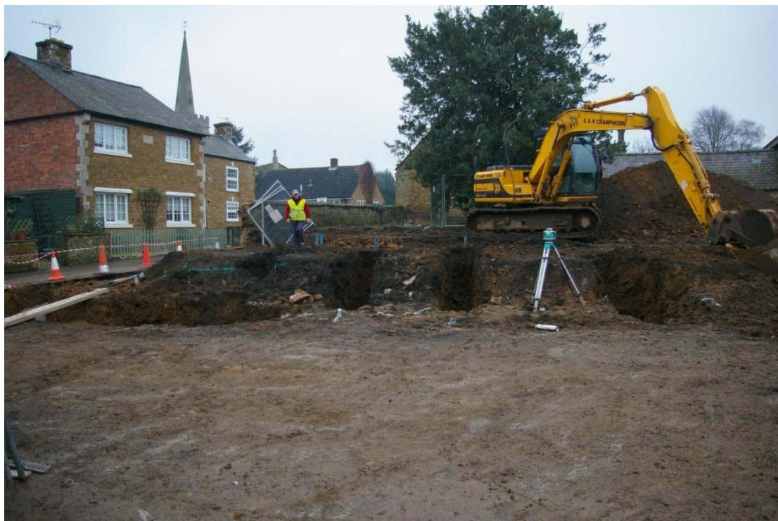
Figure 8 Detached house foundations Looking south
