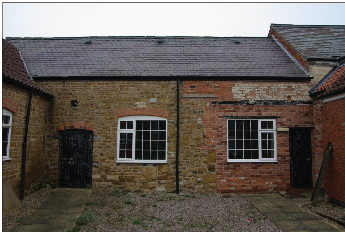
Figure 30 High Street barn from courtyard Facing north
