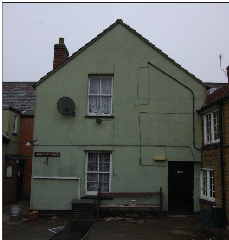
Figure 17 Rear of south extension Facing north
