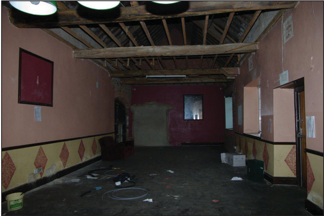
Figure 34 High Street barn Facing east
