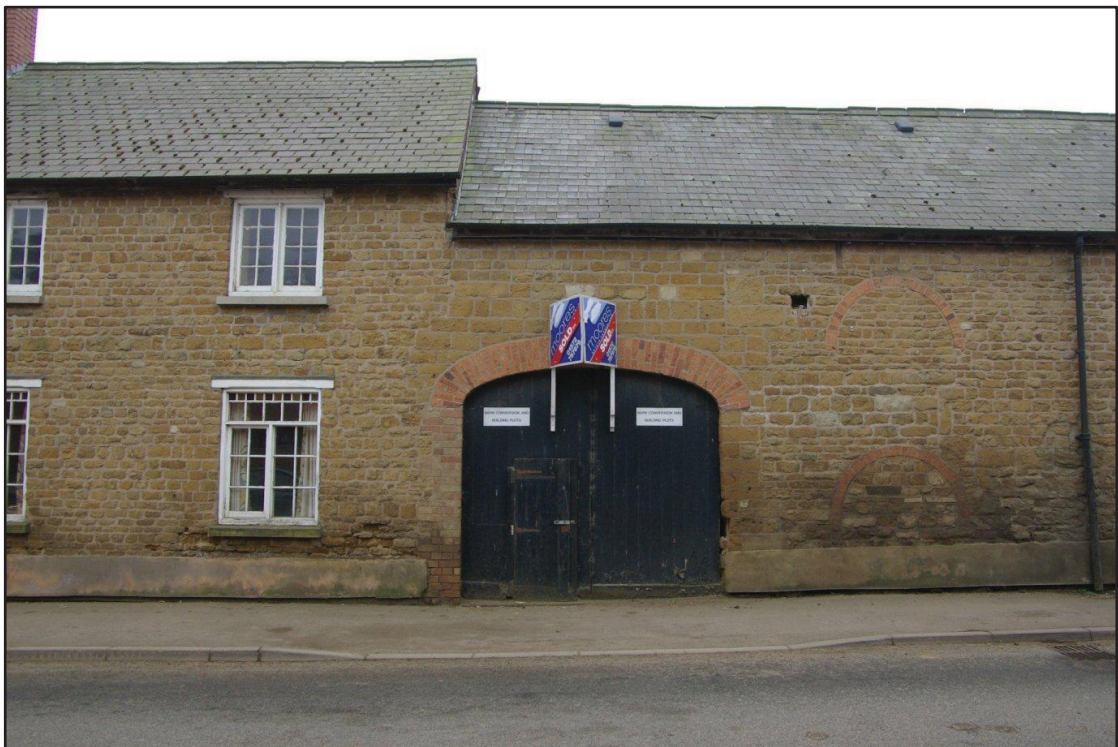
Figure 11 High Street barn entrance Facing south
