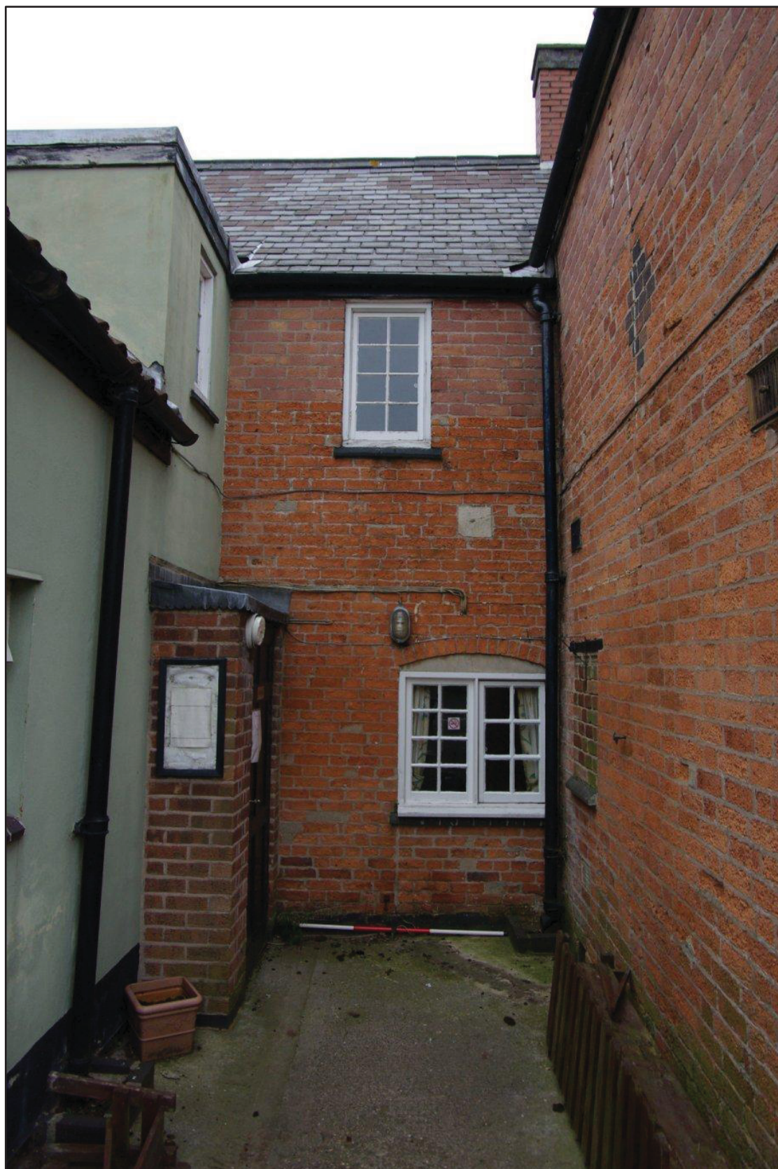
Figure 19 Rear face of High Street range Facing north
