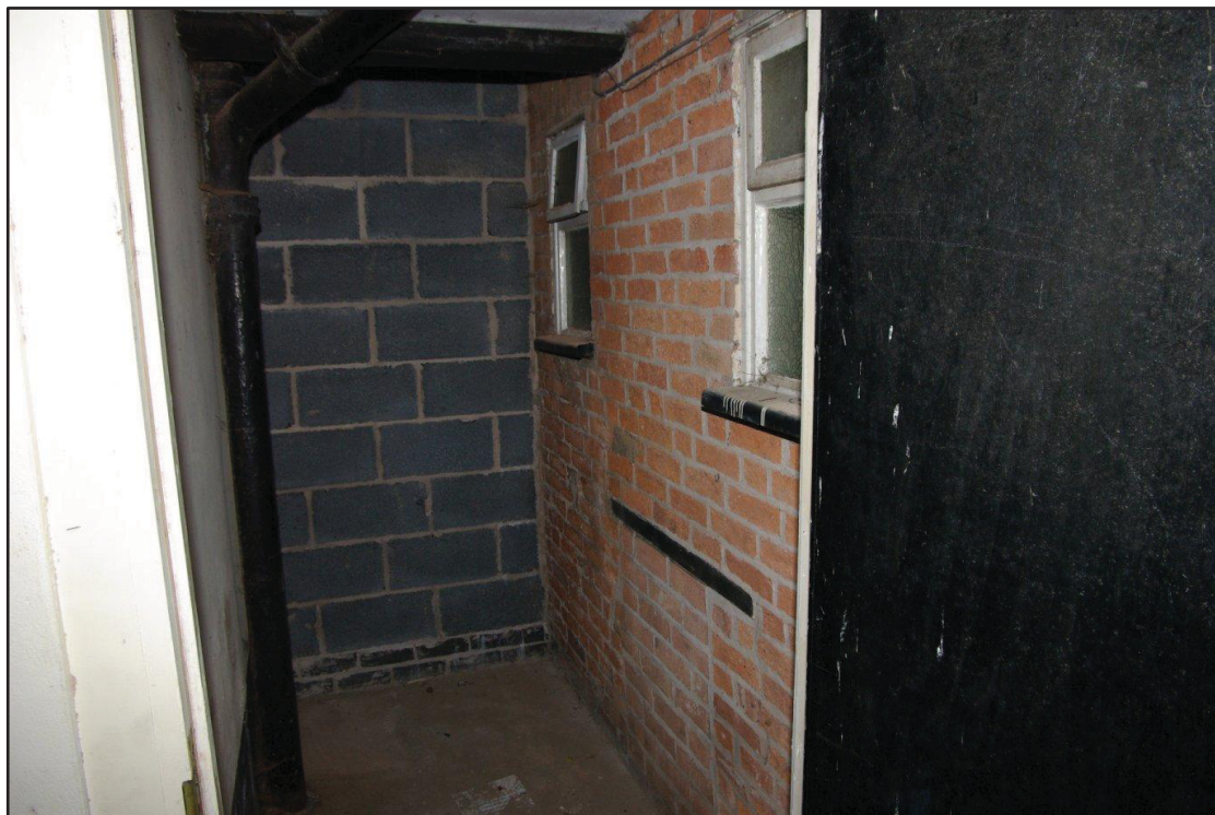
Figure 20 Blocked windows in rear wall of High Street range Facing north-west
