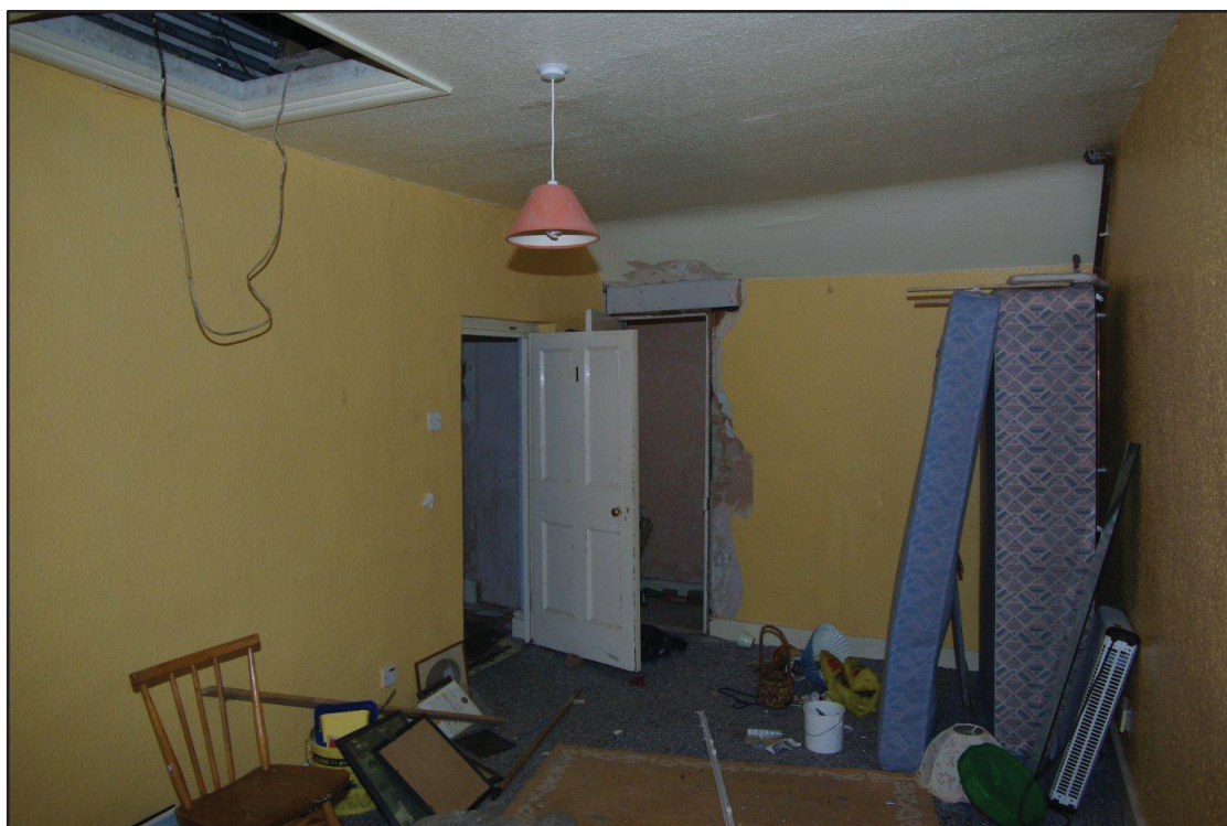
Figure 25 Bedroom One Facing south-east
