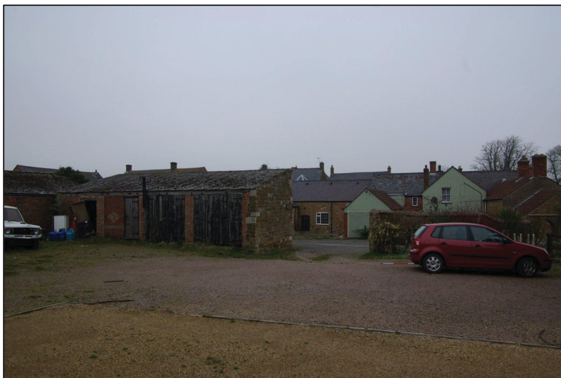
Figure 33 Lean-to structures and upper car park Facing north-west
