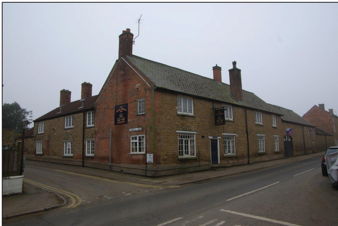
Figure 9 Three Crowns Inn Facing south-west
