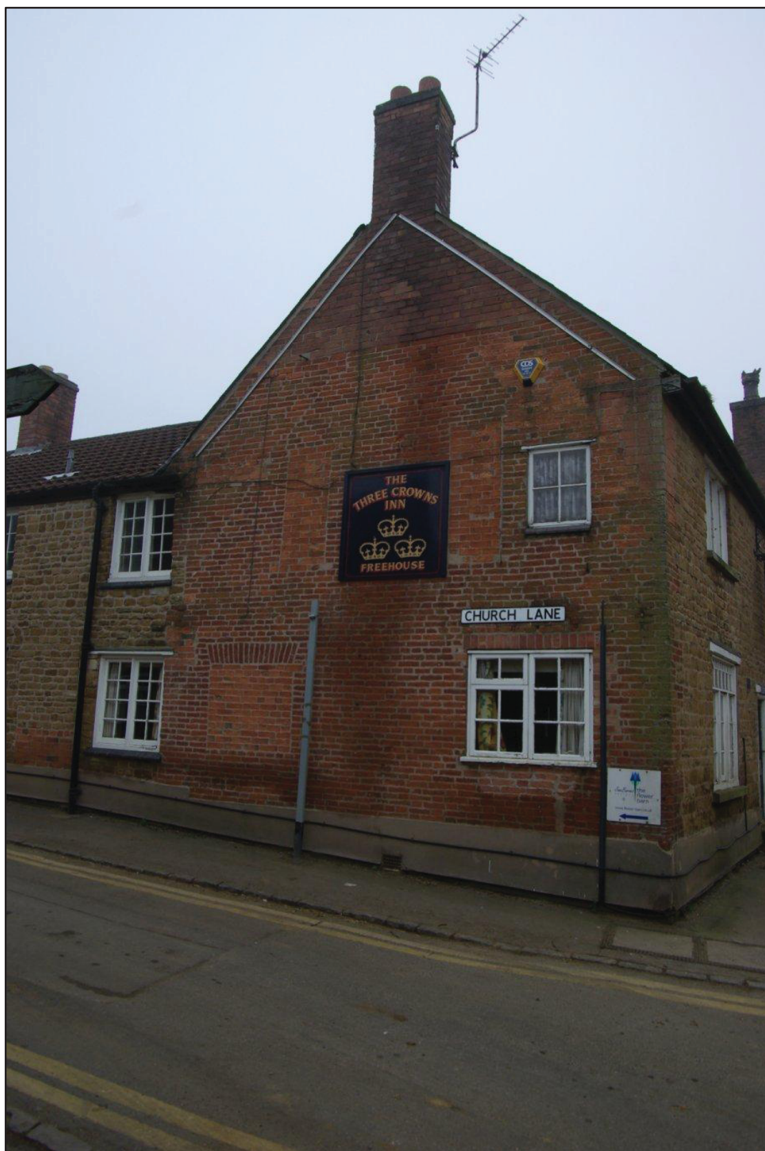
Figure 12 Church Lane gable end detail Facing south-west
