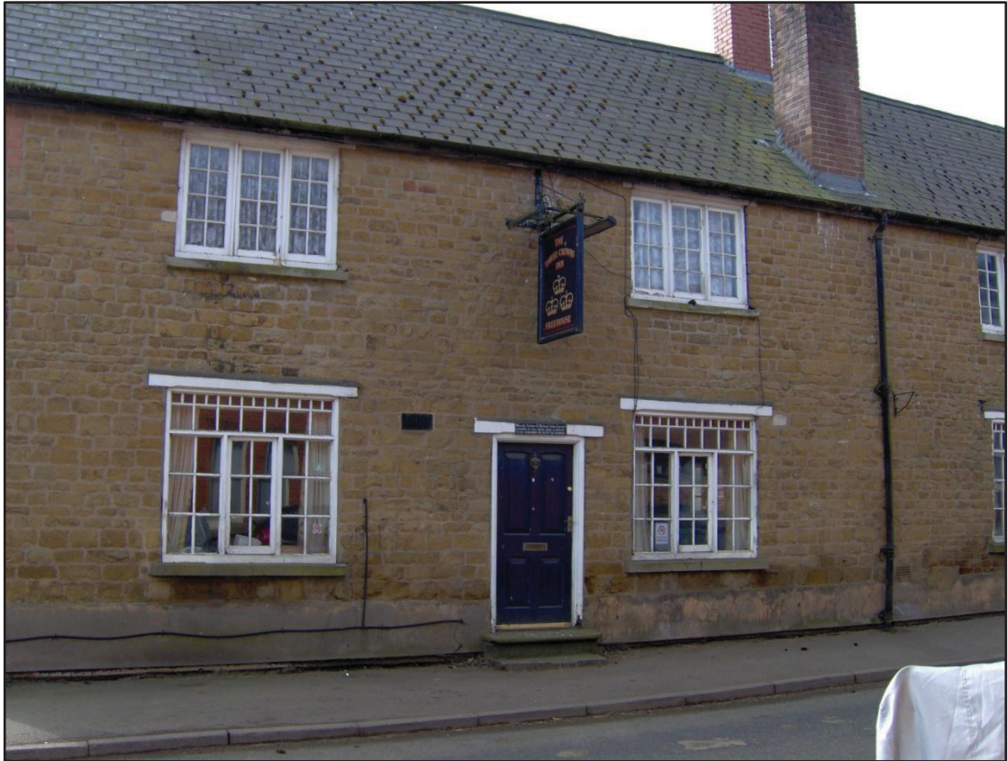
Figure 10 Main High Street frontage Facing south
