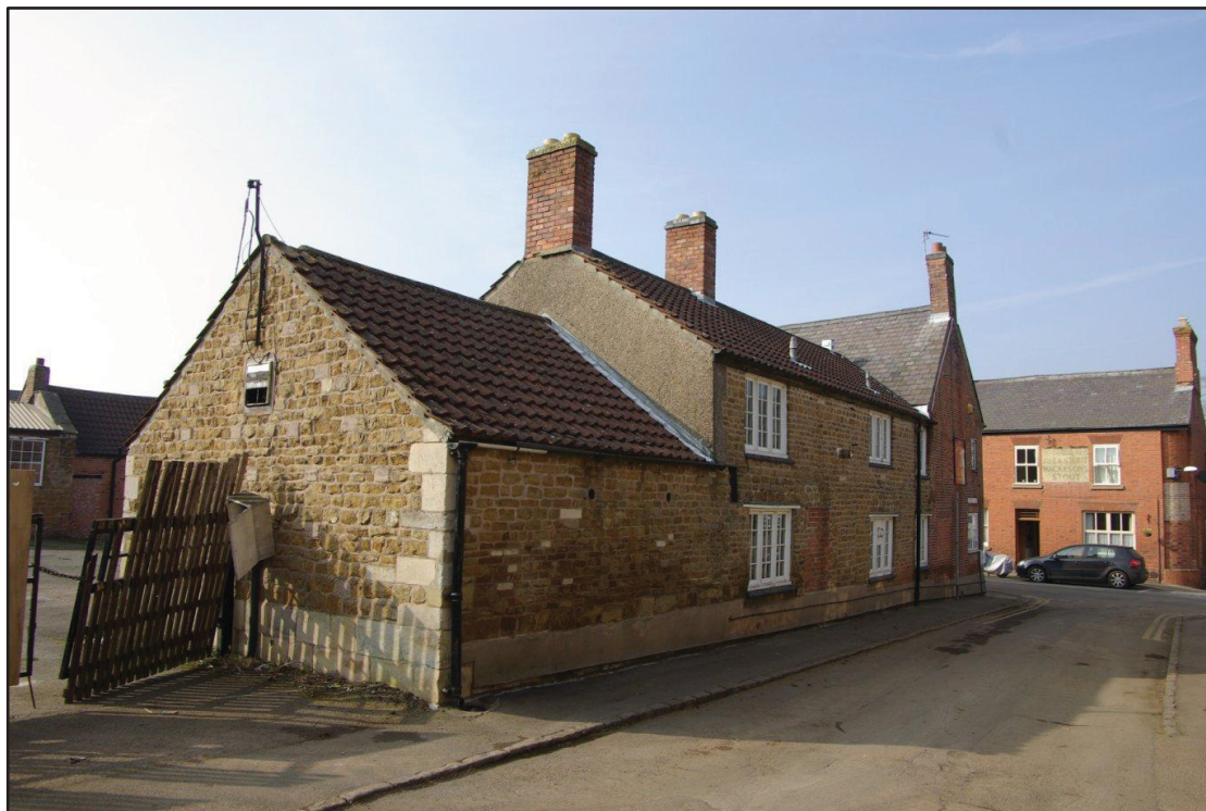
Figure 15 Church Lane range Facing north-west
