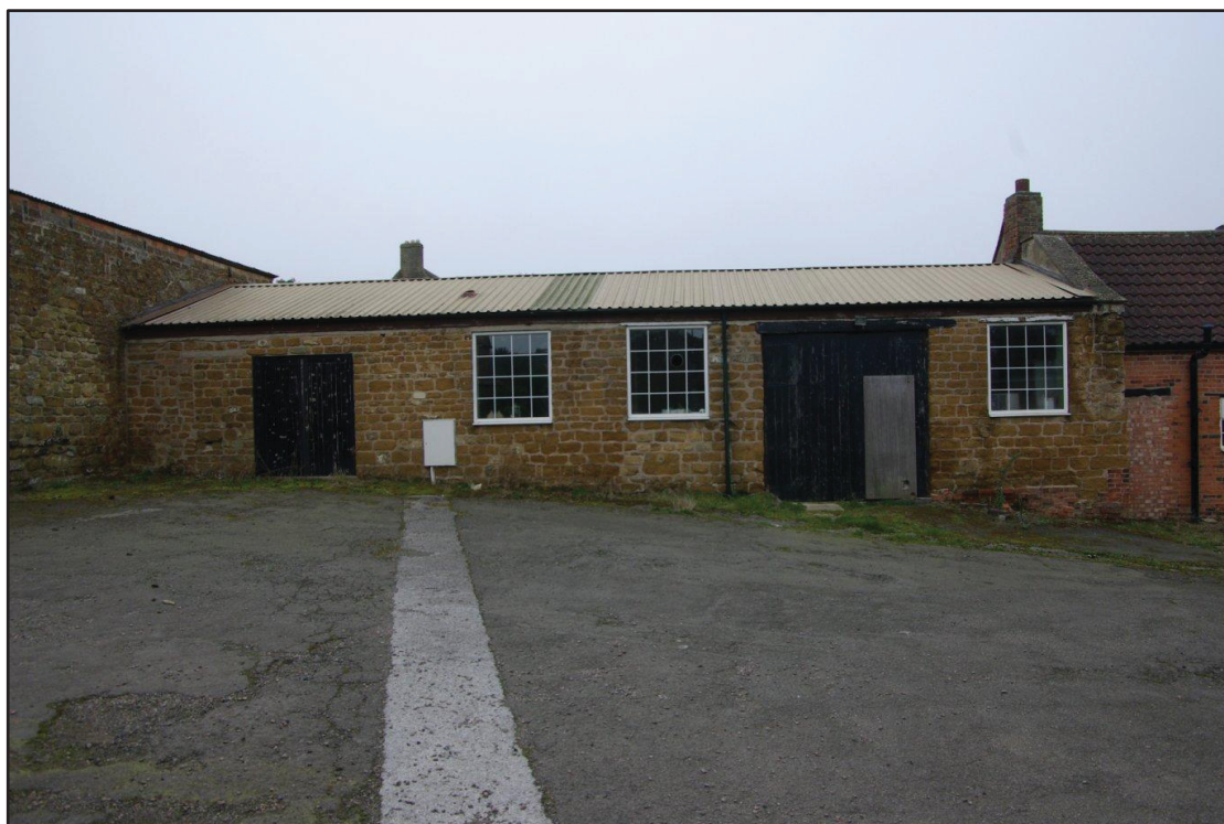
Figure 32 western barns, south end Facing west
