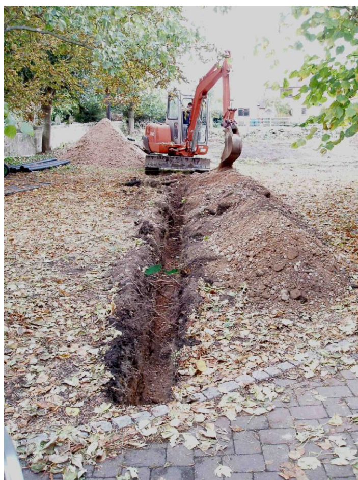
Figure 8: Machining of cable trench in progress; view north
