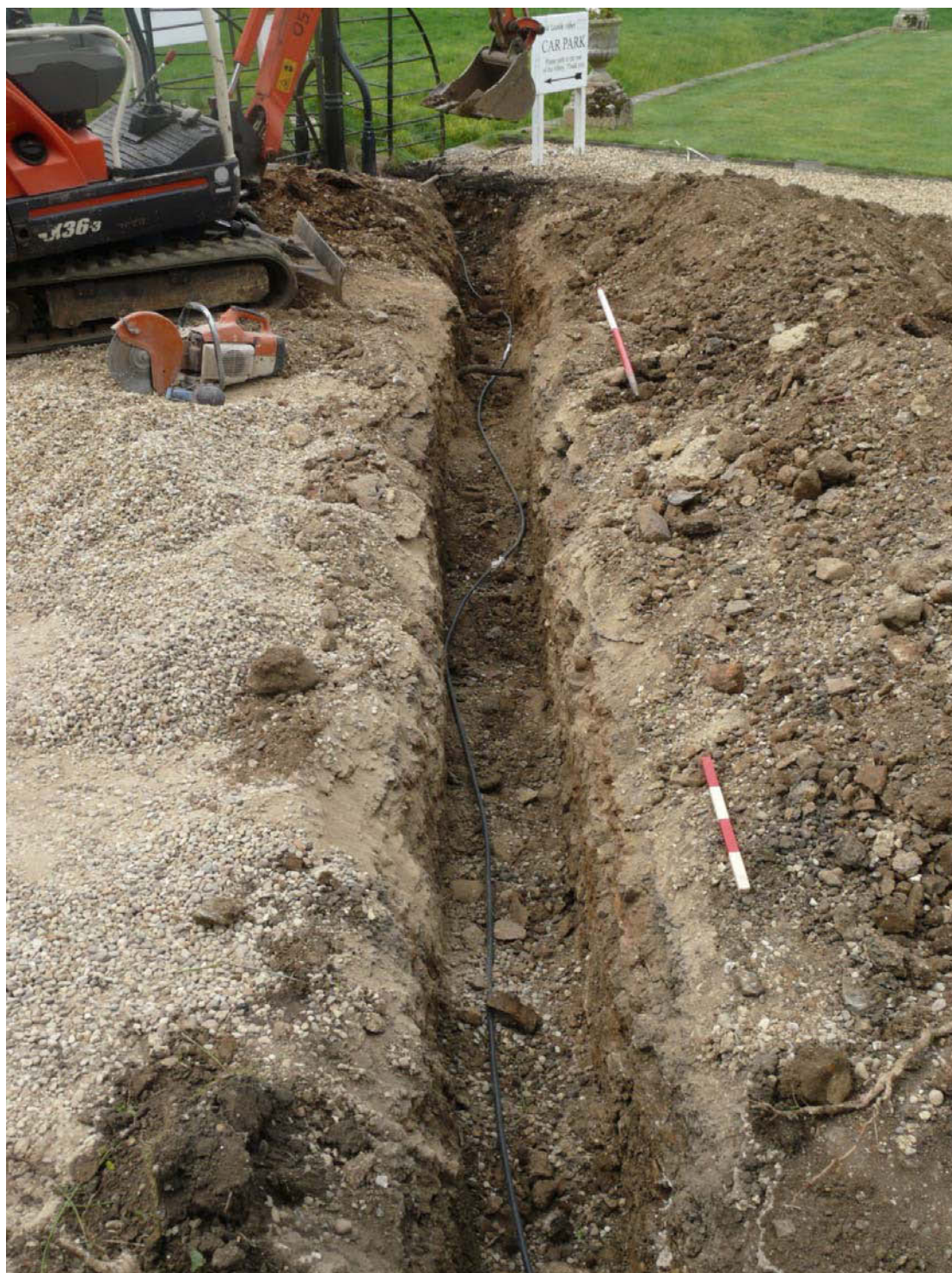
Figure 7 Cable trench from house to Ha-ha Facing north west. 1m and 50cm scales
