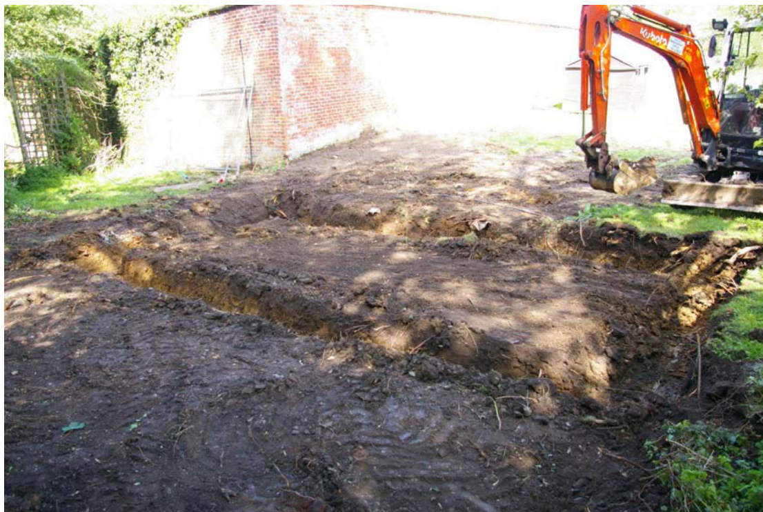
Figure 9 Foundation trench for Oxford and Cambridge Building Facing north east
