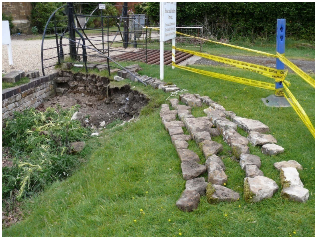
Figure 3 Side wing wall on south side of Ha-ha Facing north east
