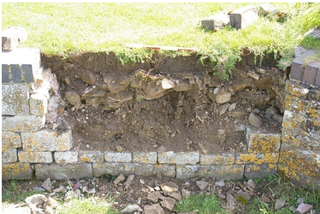
Figure 6 Southern end of north western portion of Ha-ha Facing east. 50cm scale
