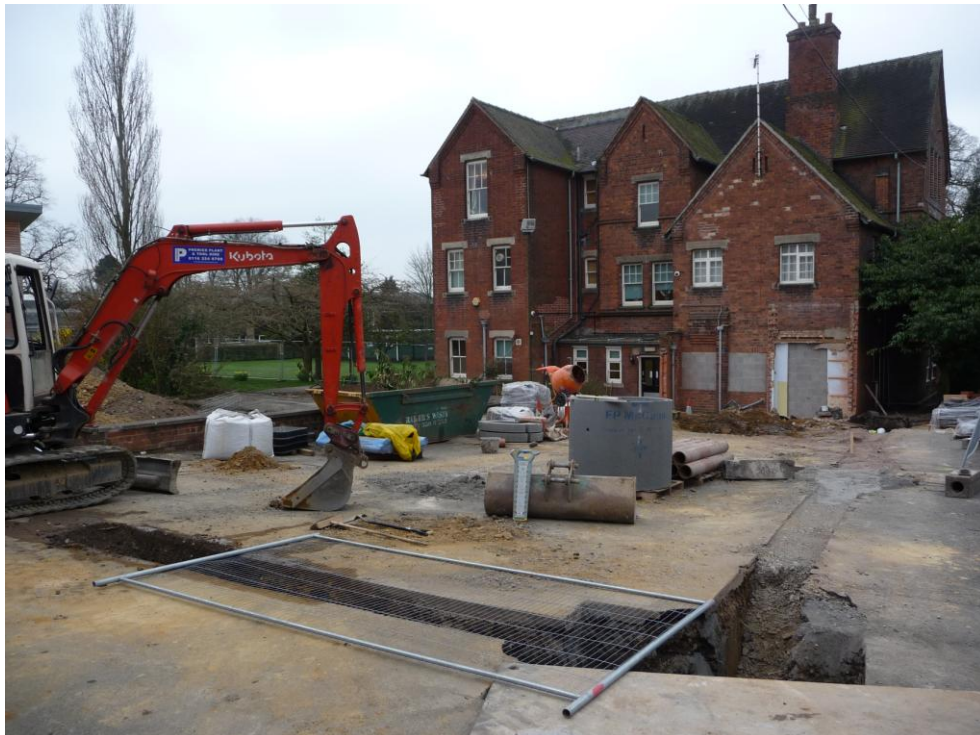
Figure 3: General view south-west across development area during installation of services
