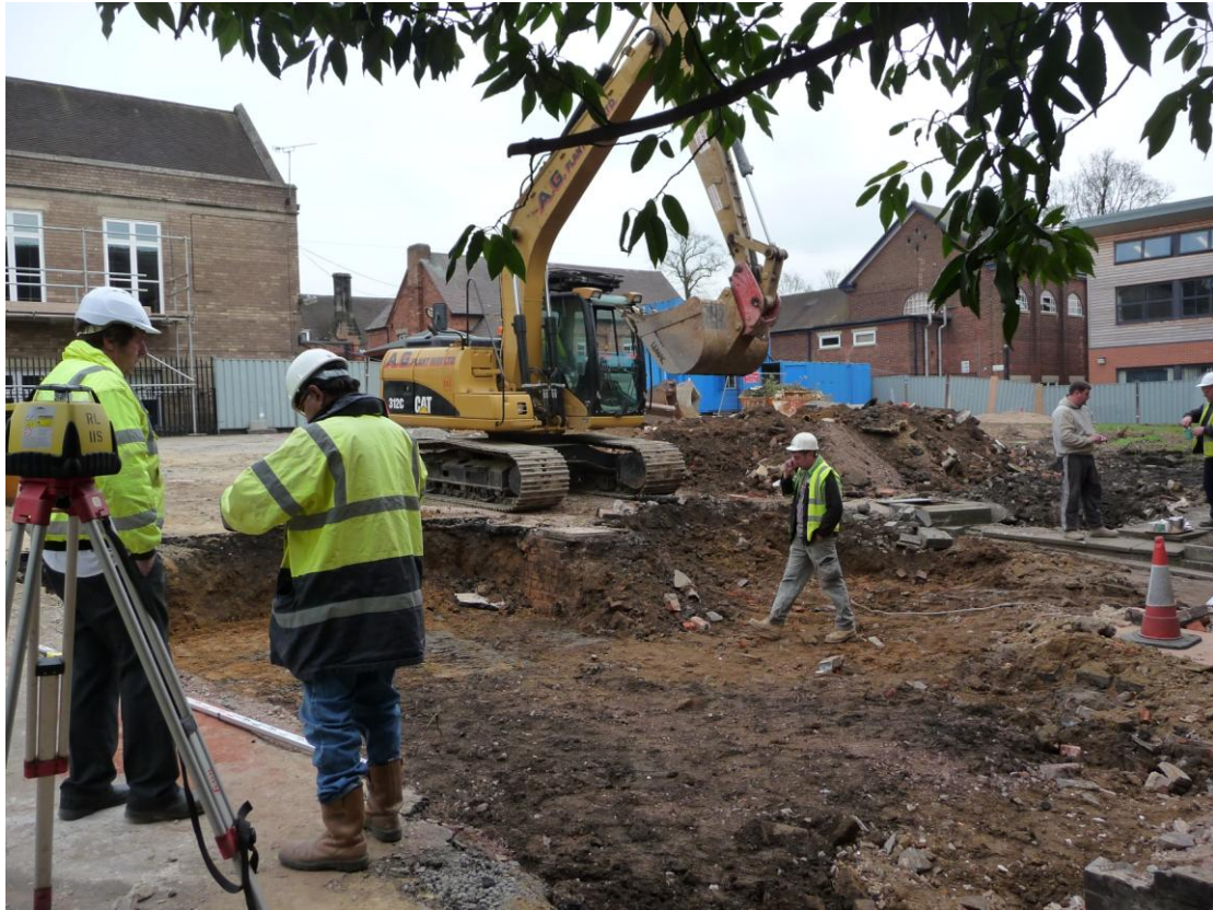
Figure 7: General view south-east during machining for floor slab
