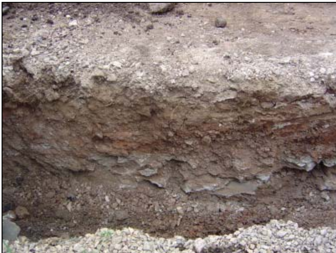
Figure 18 Foundation trench showing subsoil and natural strata.
