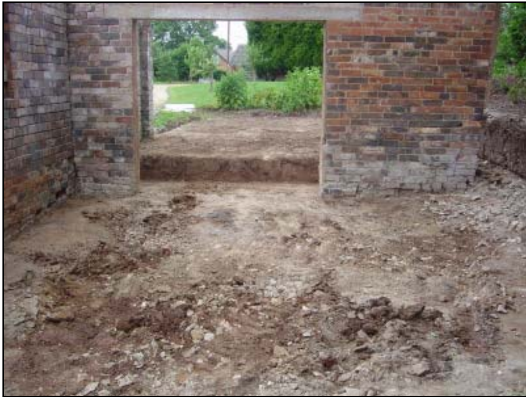
Figure 17 Interior of outbuilding during renovation.
