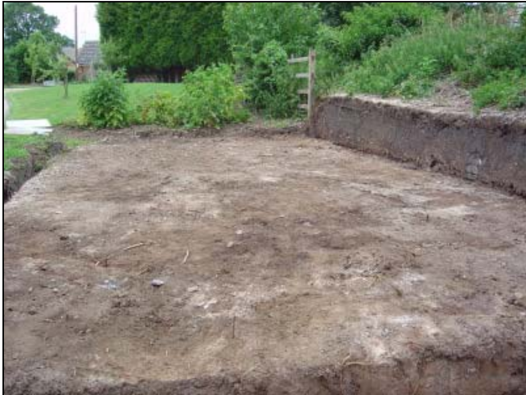
Figure 16 Conversion of outbuilding, prior to foundation trench excavation.
