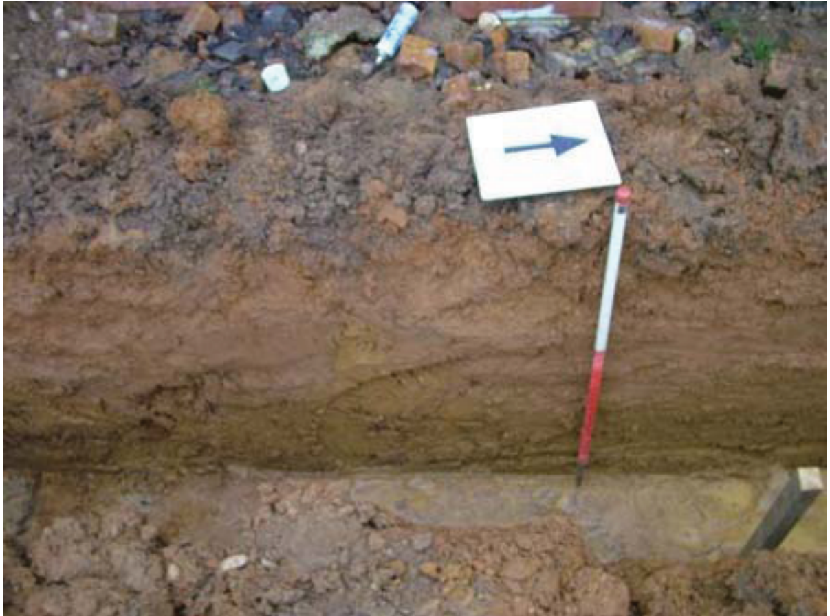
Figure 6. Excavated Foundation Trench Looking West.
