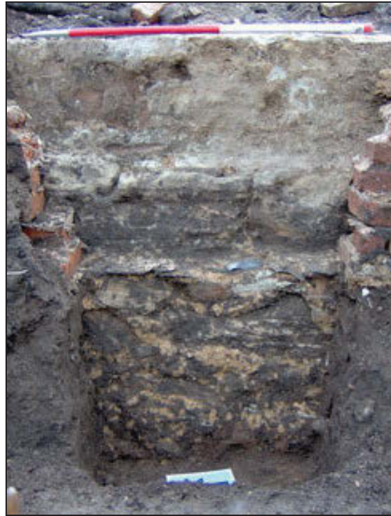
Plate 1 – The Newarke Wall in Trench three, illustrating damage, facing stone and foundation.
