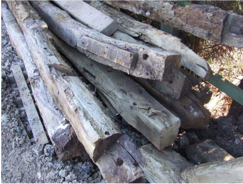
Figure 4 Detail of timbers
