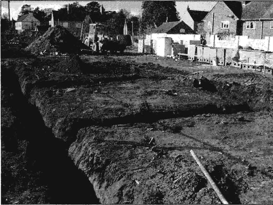
Figure 3: Working shot of site, looking west, showing excavated footings.
