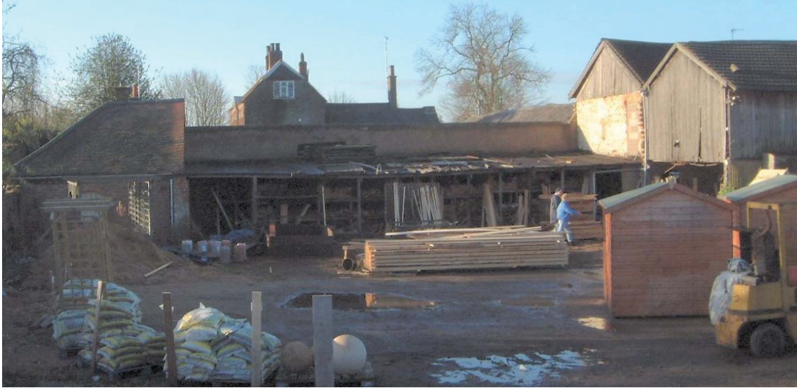
Figure 6 Pre-Demolition (Supplied by LCC).
