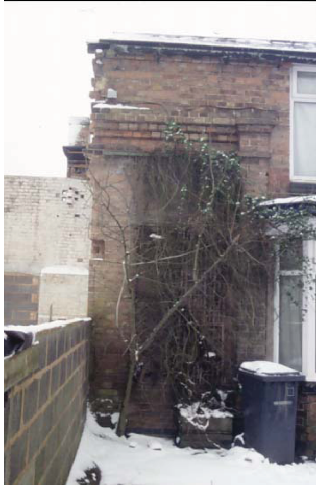
Figure 8. Decorative Brick Work on Adjoining Building
