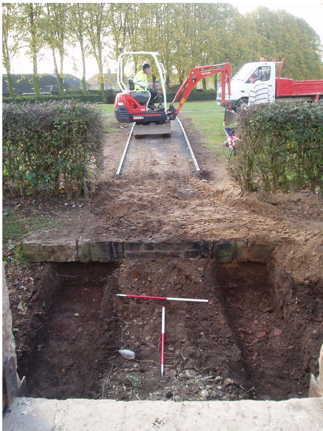
Fig.11. Trench across moat looking south
