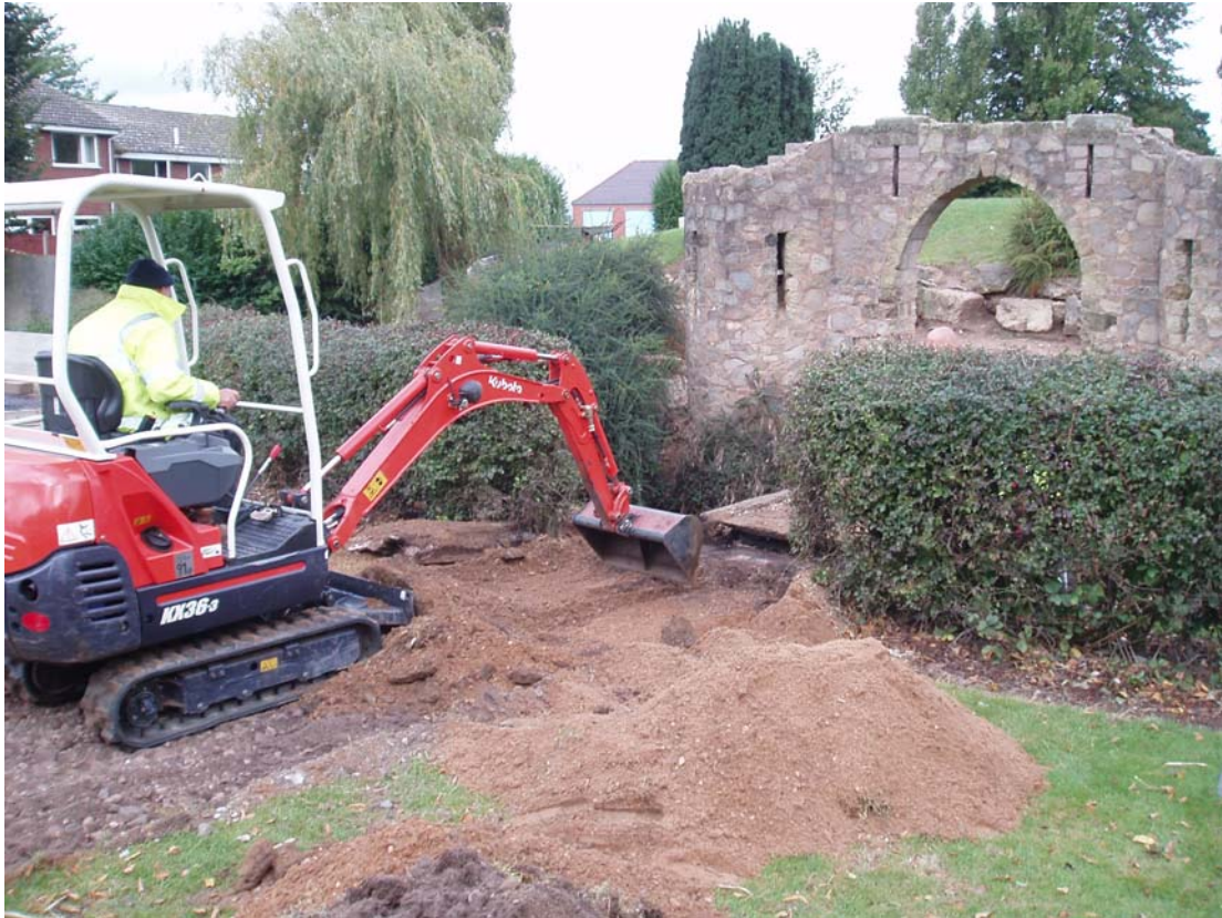
Fig.6. Working shot looking north-west
