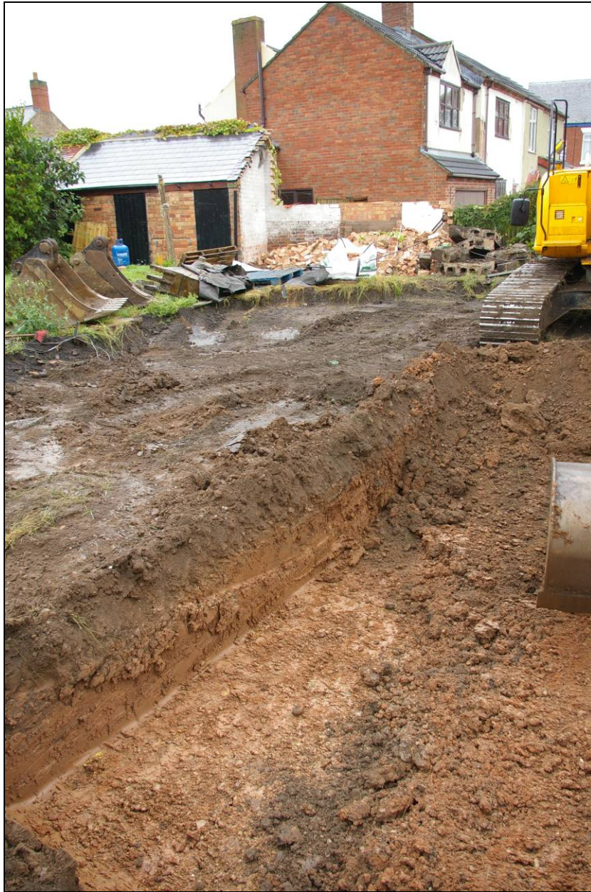
Plate 2 View of site during reduced level stripping, looking north west.
