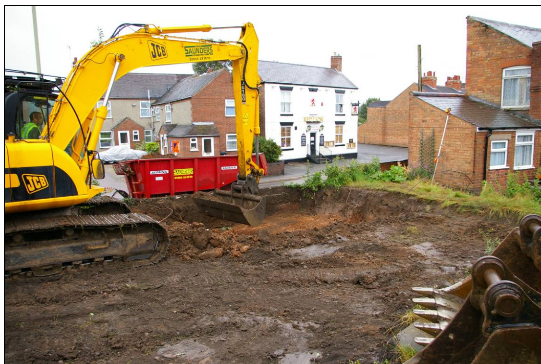
Plate 1 General view of site area during reduced level stripping, looking south east
