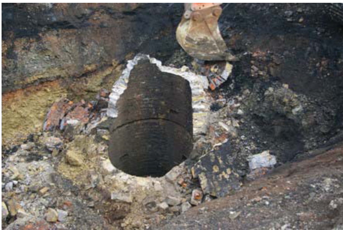
7. Demolition of Shaft (002) Showing 'Groove' and Putlog holes.
