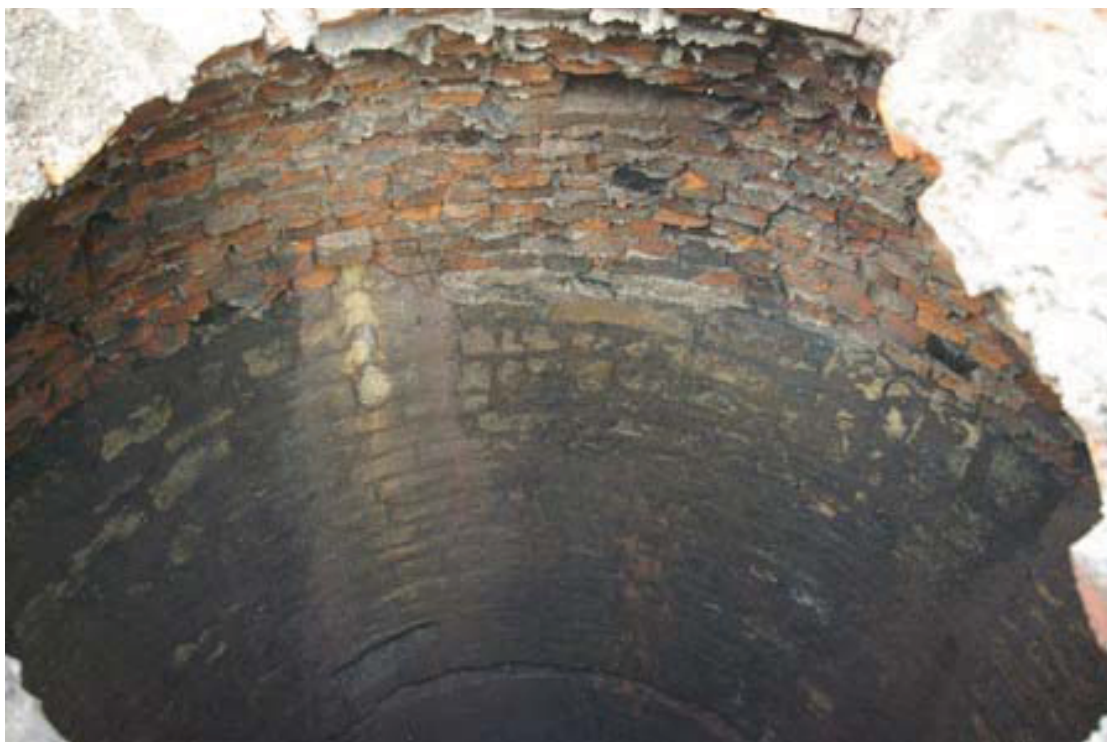
5. Looking inside the Shaft (002).
