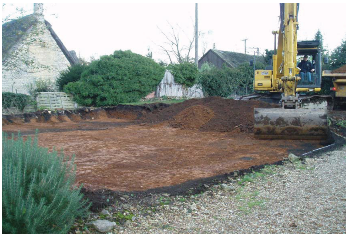
Figure 4 Controlled soil stripping. Looking East
