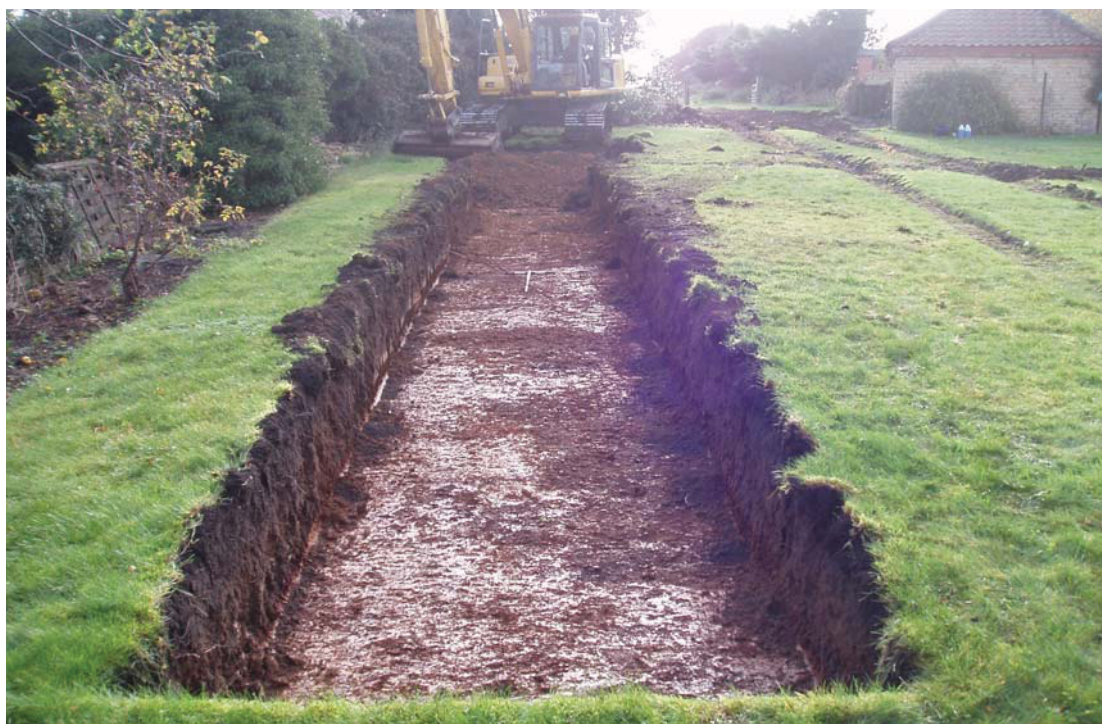
Figure 3 Preliminary Trial Trench Looking South East
