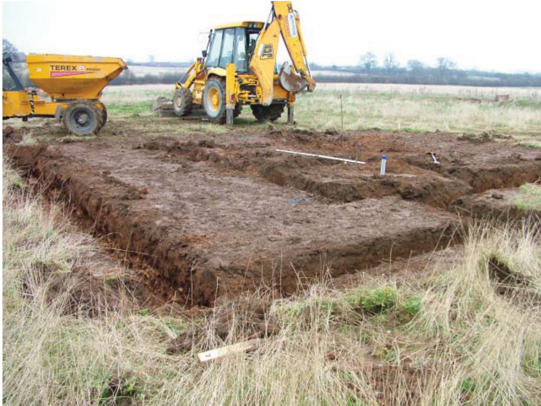
Plate 5: Close to completion, looking north east
