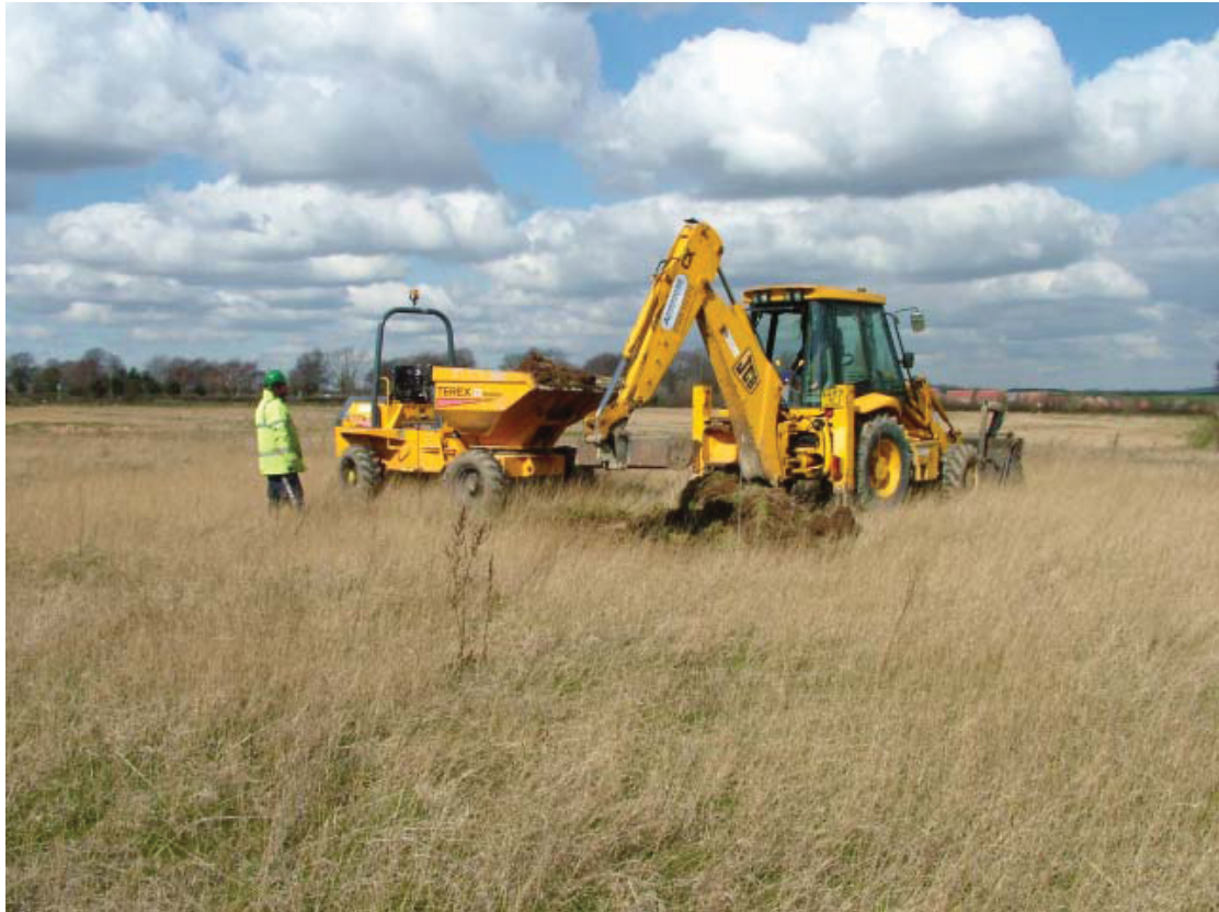
Plate 1: Work in Progress. Looking north west
