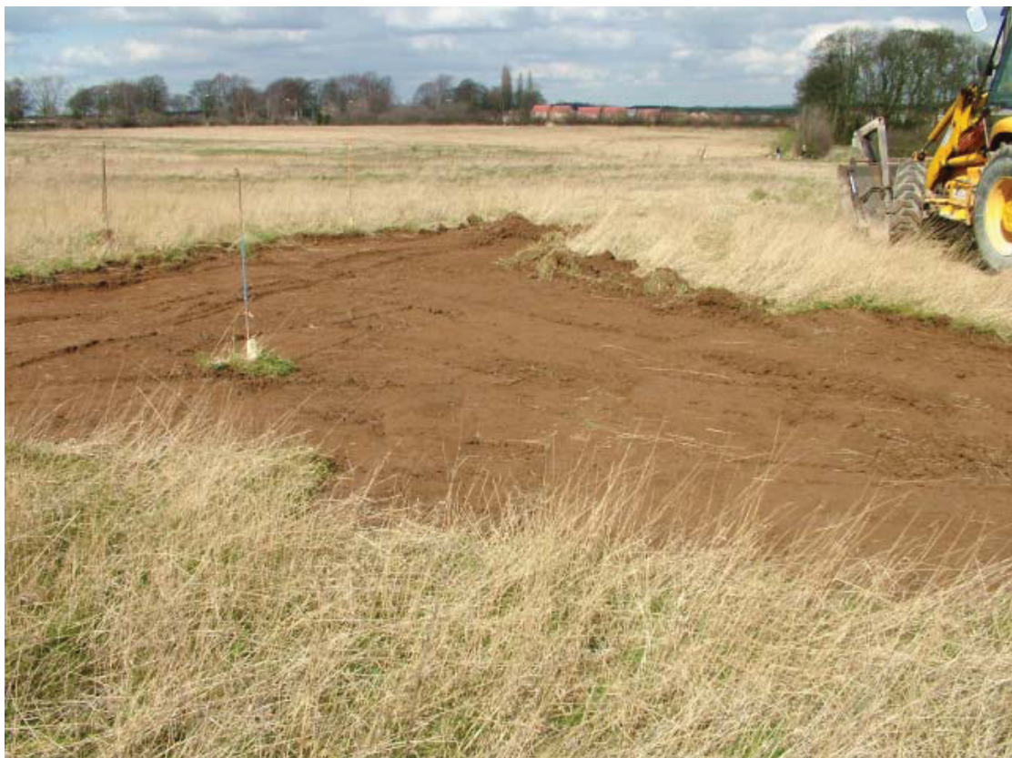
Plate 2: Area stripped prior to marking out, looking north west
