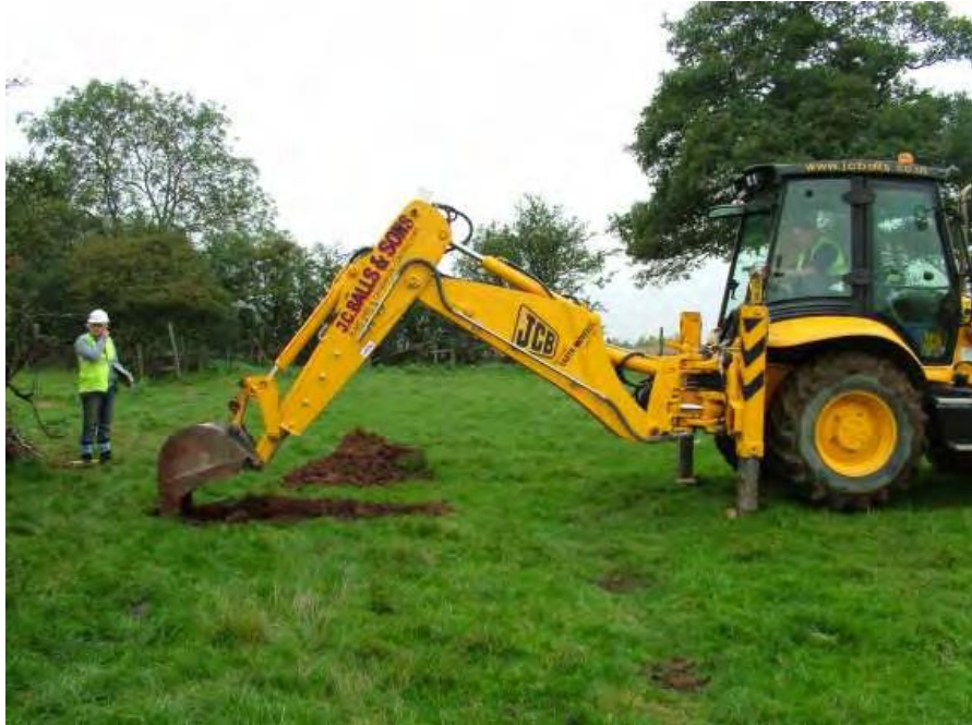
Plate 1: Work in progress on Trench 1070, looking south
