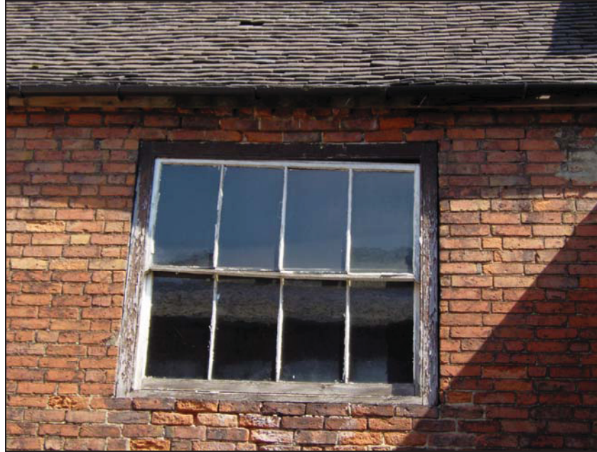
Figure 11: Large sash window facing the courtyard, Room G.
