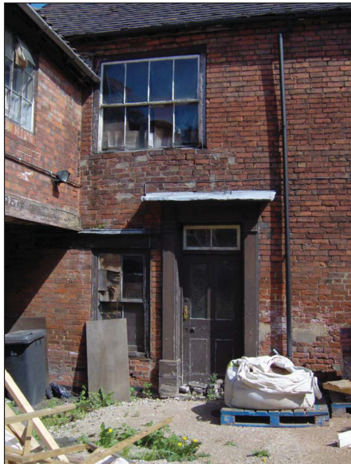
Figure 8: Sash window (Room A) and main courtyard entrance (Room B).
