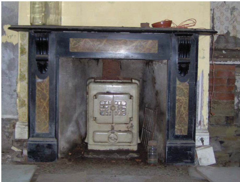
Figure 9: Room C, painted slate fire surround . Note the sandstone footings revealed to the right of the fireplace.
