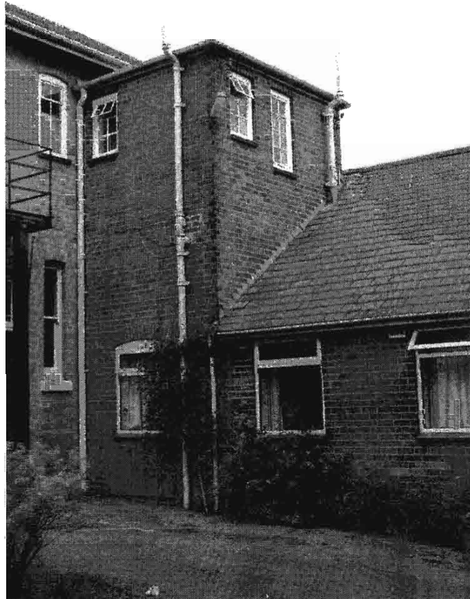
Plate 18. Two storey section of south-east extension looking north (see also Plate 7).
