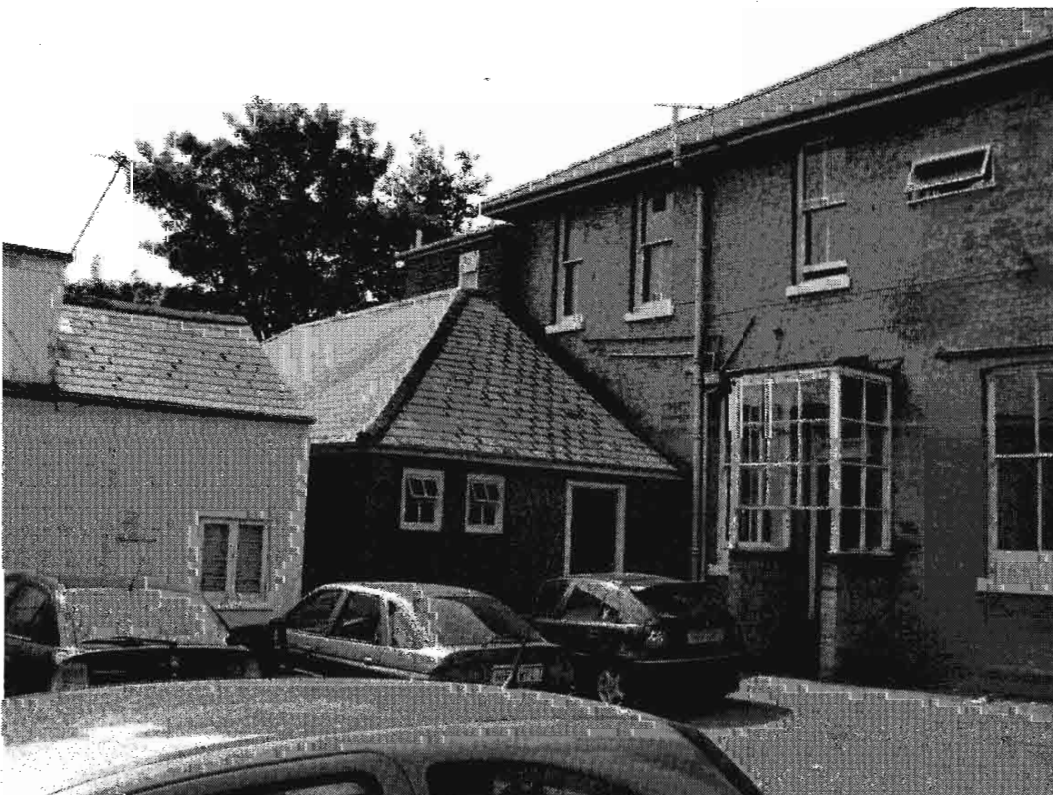
Plate 4. Later extension obscuring the eastern end of the north-east elevation.
