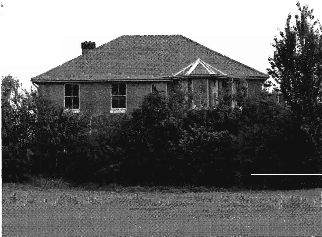
Plate 9. View of the south-west elevation taken from the recreation ground.
