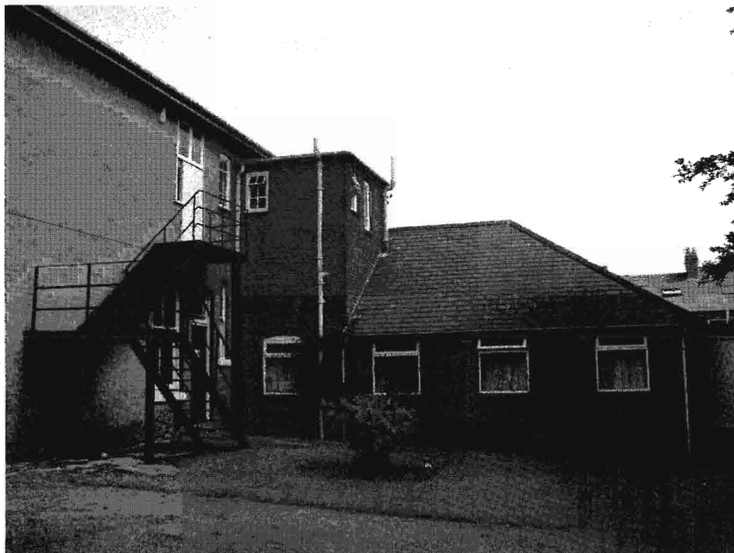
Plate 7. View of the south east elevation and later two storey south-east extension.
