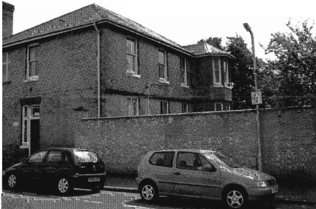
Plate 19. The southern section of boundary wall on Radmoor Road.
