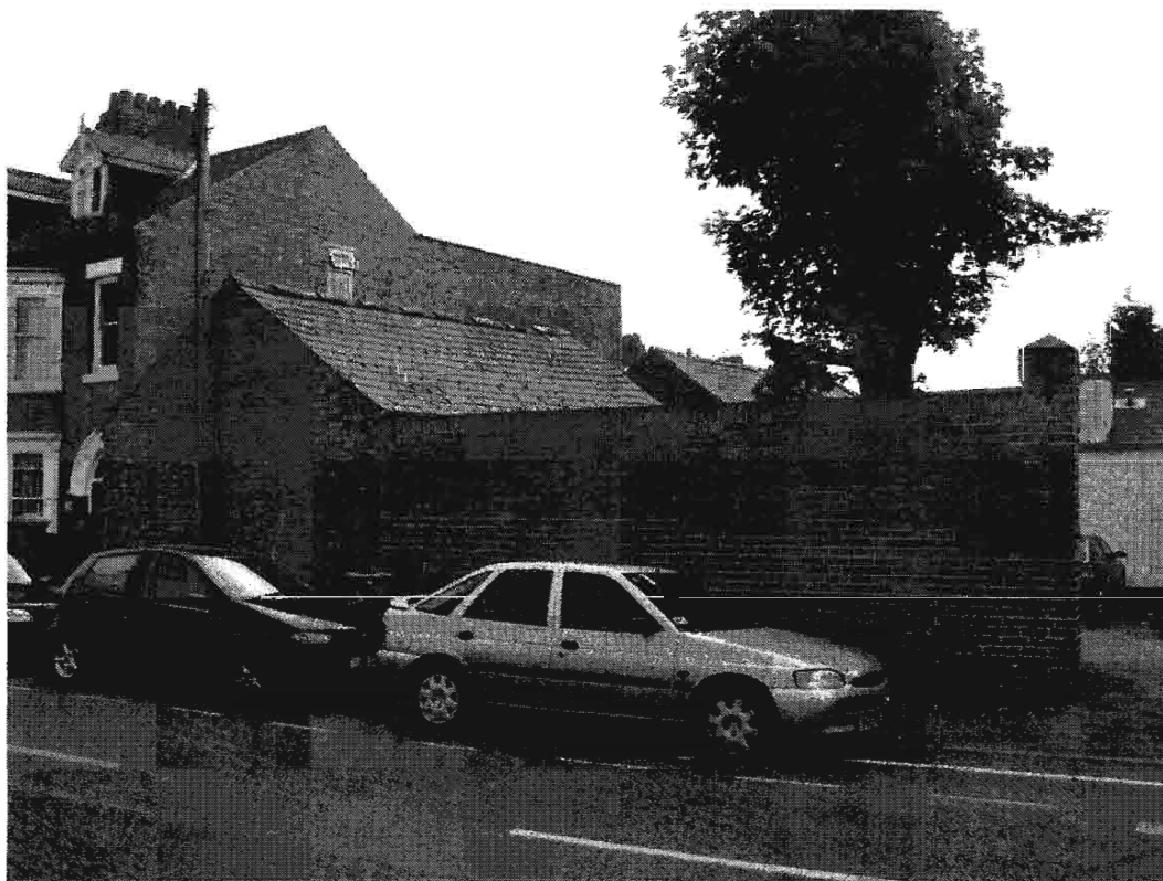
Plate 14. The northern courtyard building from Radmoor Road showing adjacent boundary wall.
