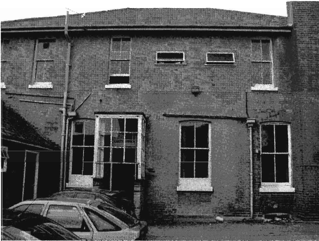
Plate 3. General view of central section of north-east elevation.
