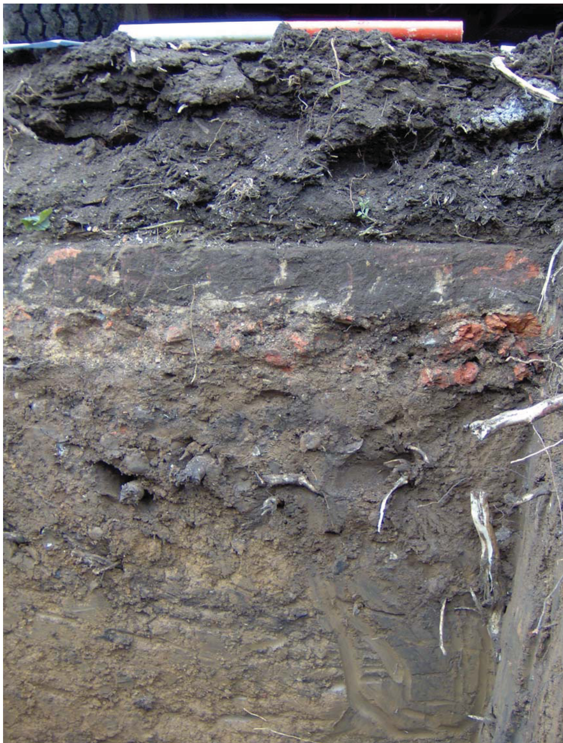
Figure 6 Section of foundation trench showing concrete, made ground and Liassic clay natural substratum
