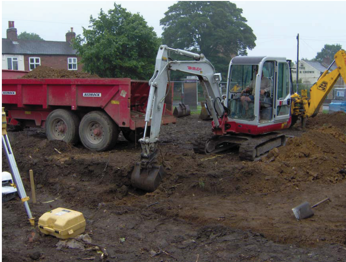
Figure 5 Excavation of foundation trench in progress
