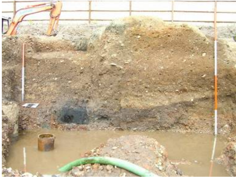
Plate 11: Section viewed north across structural timber (left) and rampart material (right, above)
