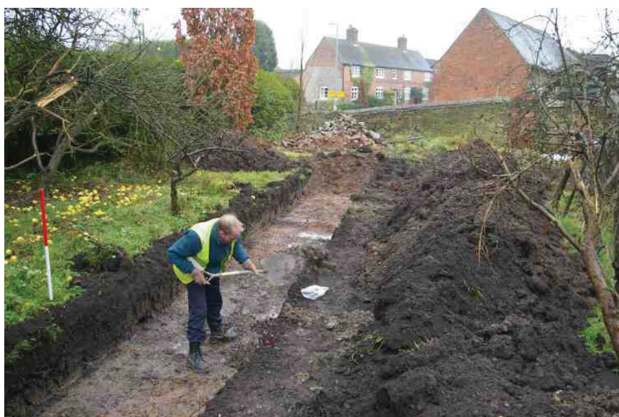
Figure 3: General view of site looking south-east
