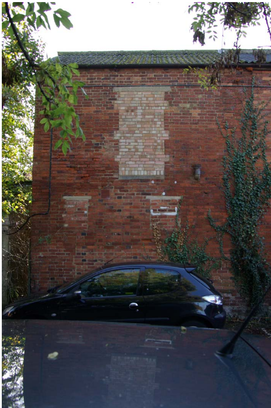
Figure 15 Unit B Detailed View of Rear (North) Elevation Showing Blocked Openings.
