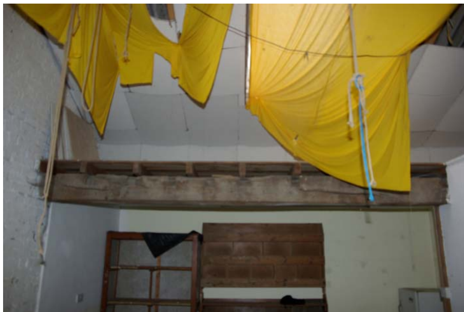
Figure 20 Unit B Wall Plate Showing Position of Original Wall.
