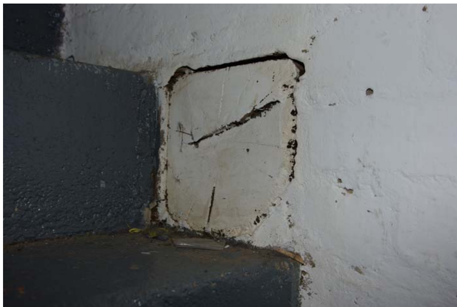
Figure 18 Unit B Axial Beam Seen in Stair Wall
