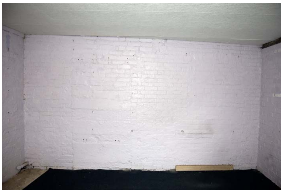
Figure 17 Unit A Blocked Openings in Right Hand (Eastern) Gable.
