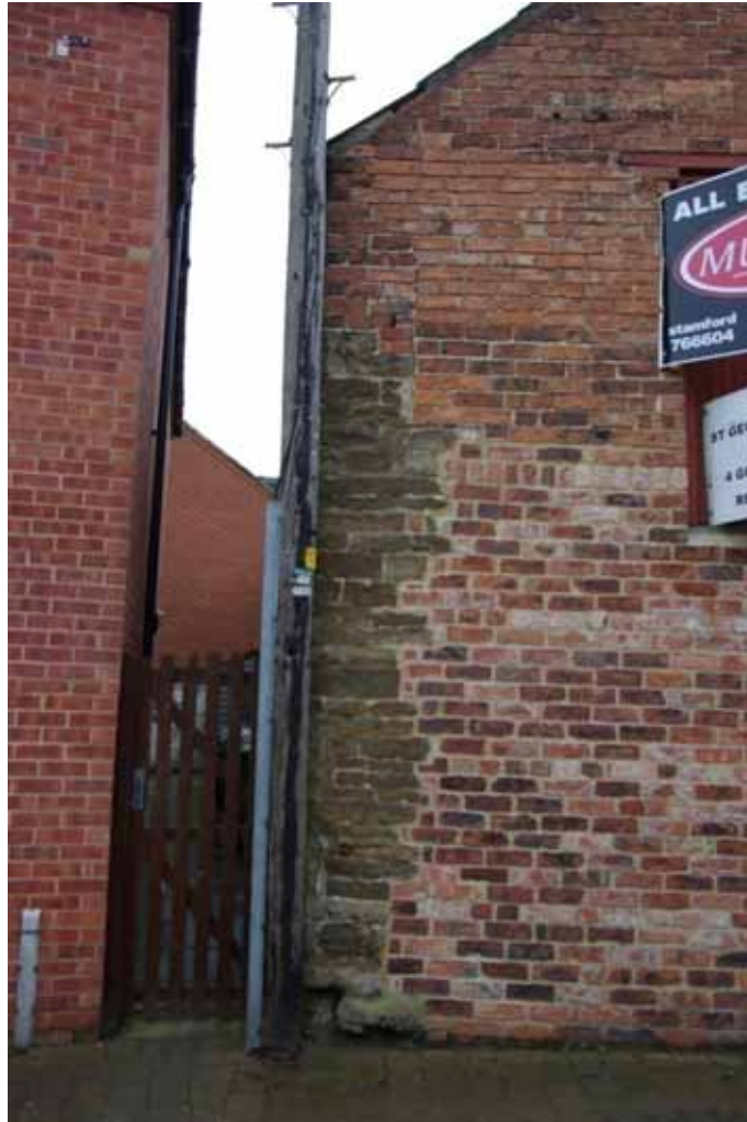
Figure 12 Eastern Gable of Building A Showing Different Building Phases.
