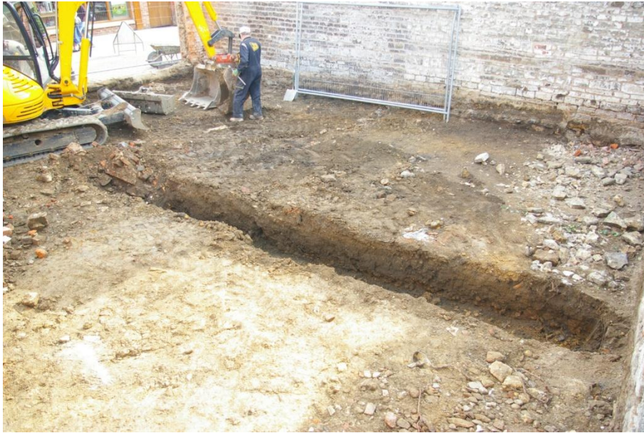
Figure 5 Work in Progress (looking south east).
