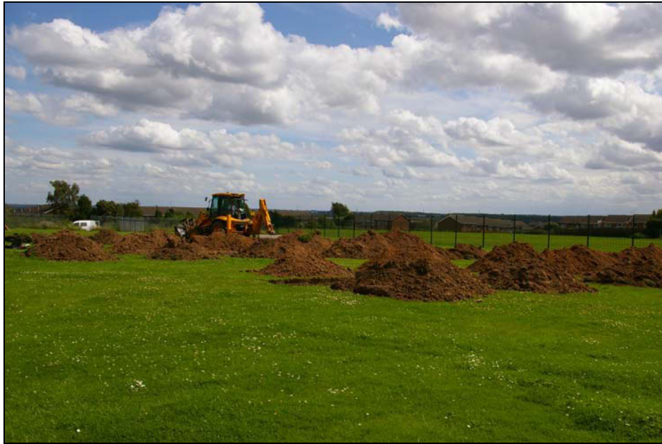
Figure 2: General view from south-east of site
