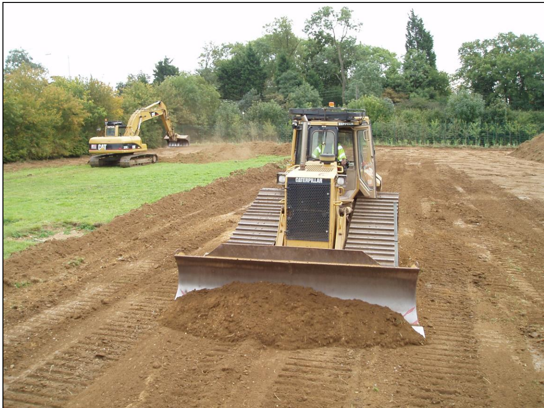
Figure 4: Topsoil strip in progress; view north
