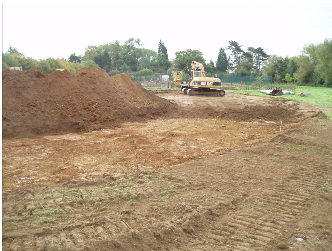
Figure 5: Machining of balancing pond in progress; view north-east
