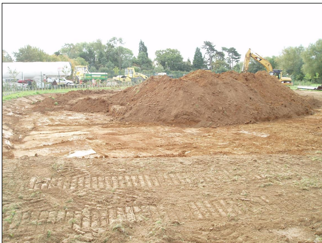
Figure 6: Machining of balancing pond; view north
