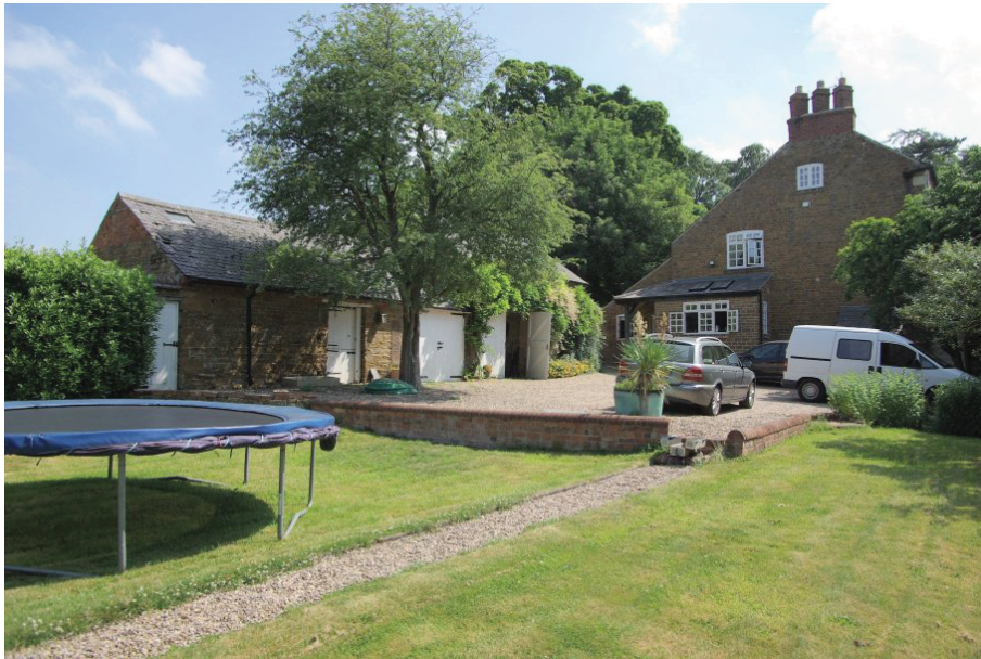
Figure 5 Outbuilding & Halstead Grange.
