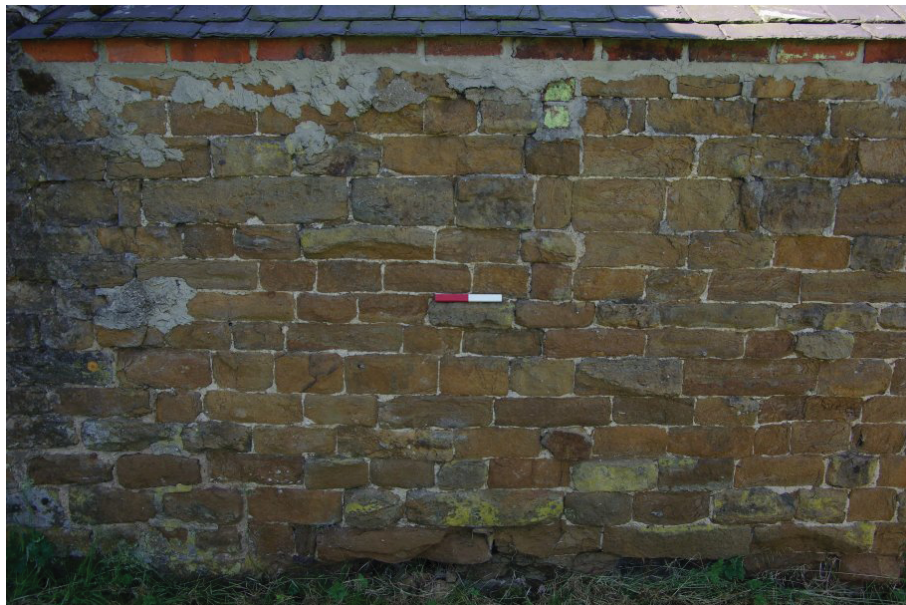
Figure 10 Quality of Stonework on Northern Wall.
