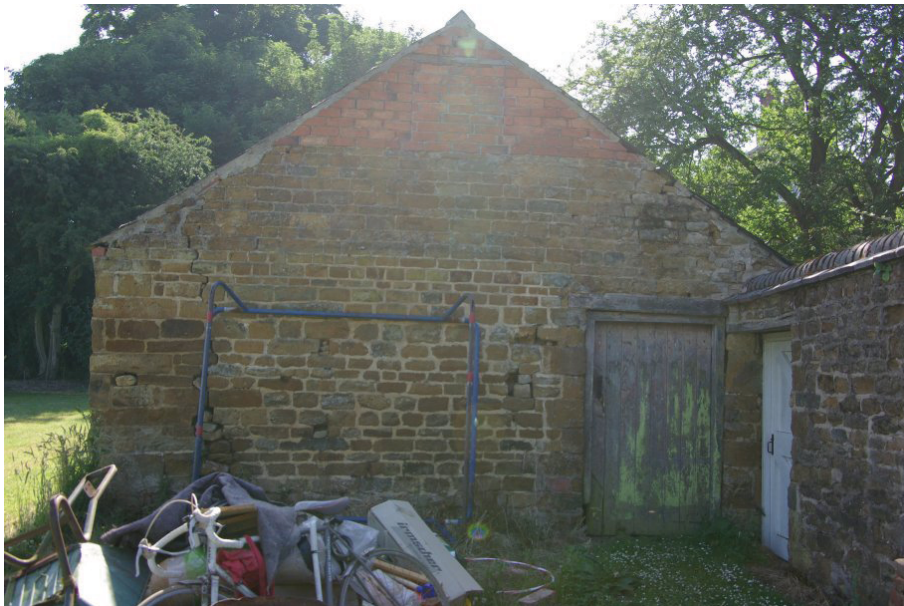
Figure 6 Western Gable With Additional Brickwork.
