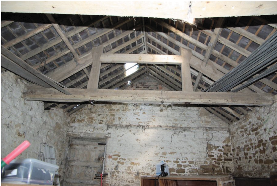
Figure 7 Queen Post Truss in bay a .
