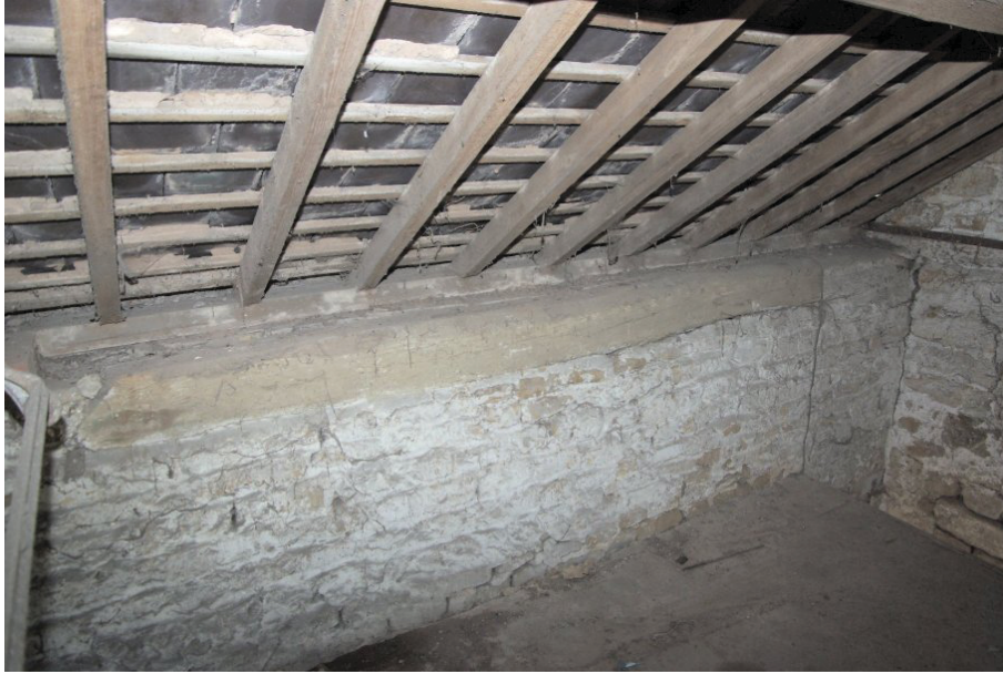
Figure 13 Re-used Tie Beam in Southern Wall of e .
