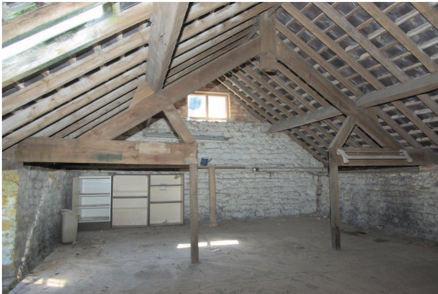
Figure 12 Modified Truss, e .
