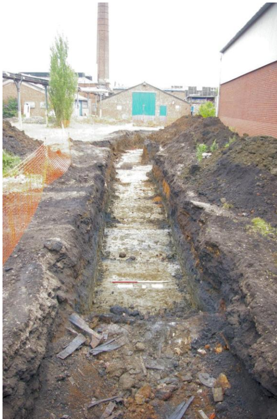
Figure 4 Trench 3 looking south.
