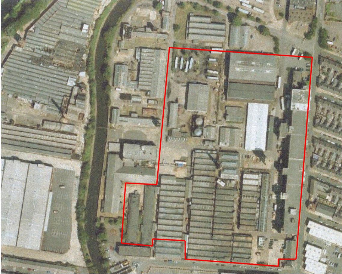
Figure 54 Aerial Image of Proposed Development Area Prior to Partial Demolition of Southernmost Buildings.
