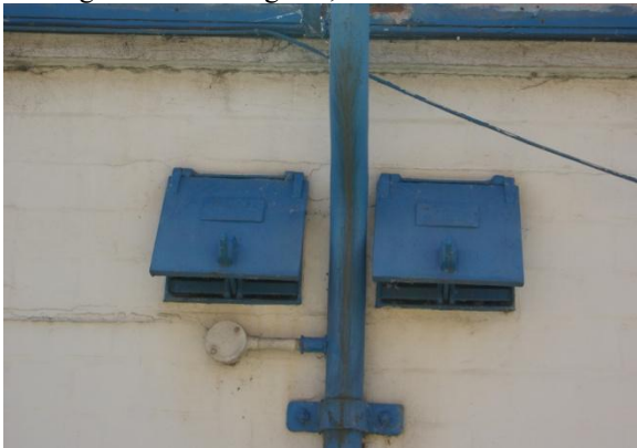
Figure 43 Building 72a; closing air vents.
