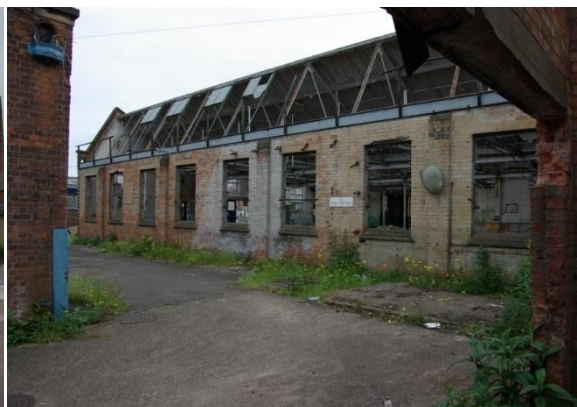
Figure 22 Building 46, Northern elevation with Camouflage.
