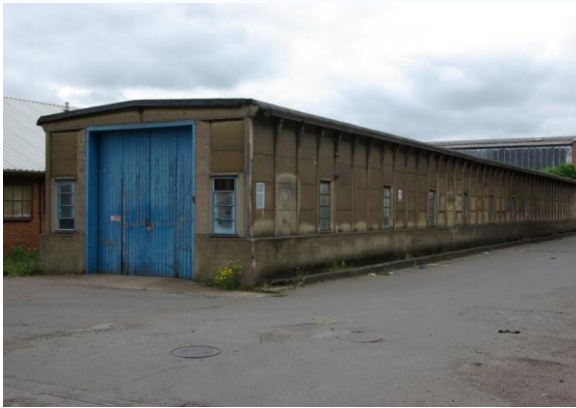
Figure 47 Building 110, southern & eastern elevations.
