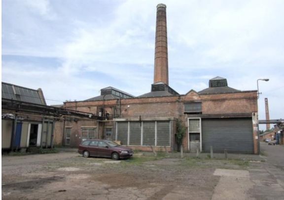
Figure 35 Building 68 boiler house.
