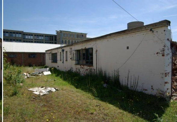
Figure 42 Building 72a, Northern elevation.
