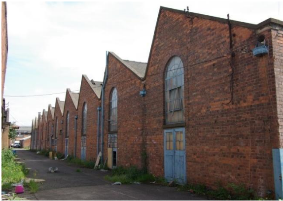
Figure 15 Building 42 Western Elevation.
