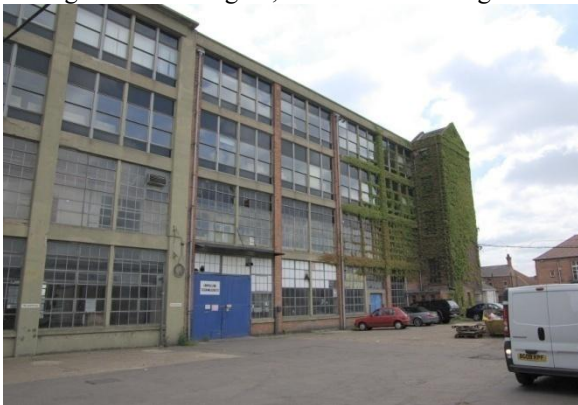
Figure 5. Building 32, Western Elevation.
