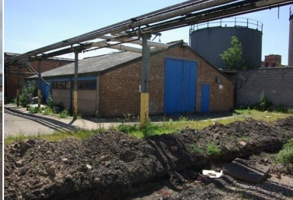
Figure 34 Building 67a, Northern elevation.
