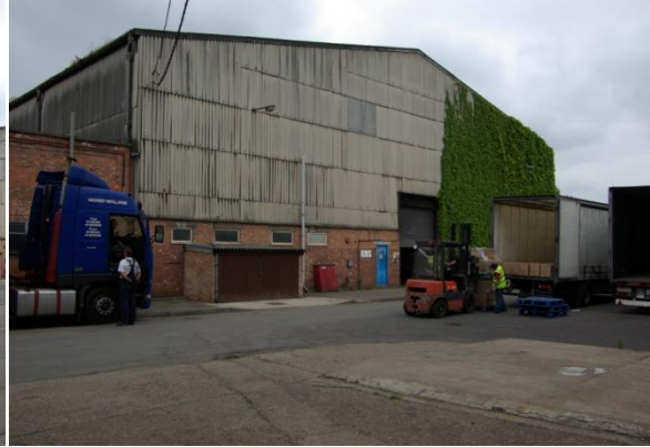
Figure 26 Building 51a, Eastern Elevation.
