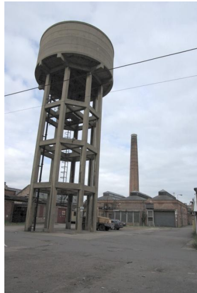
Figure 52 Water Tower, with chimney in Background.
