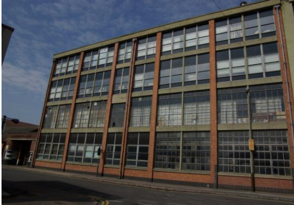
Figure 3 Building 32, Ross Walk Frontage.
