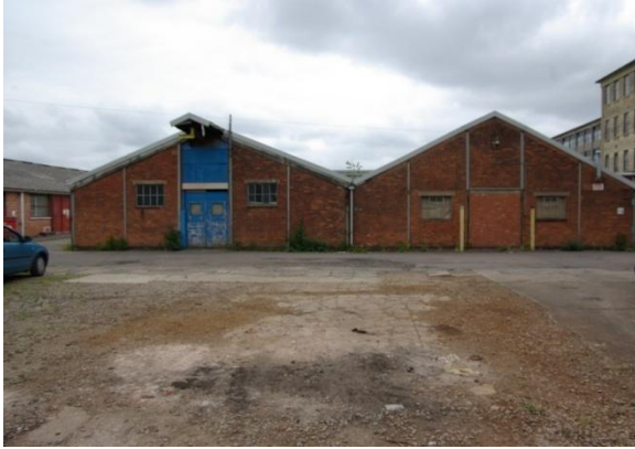
Figure 39 Building 72, Southern Elevation.
