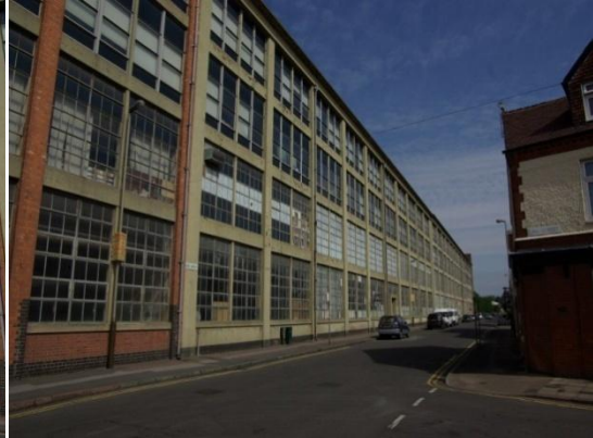
Figure 4 Buildings 39 & 96, Ross Walk Frontage.
