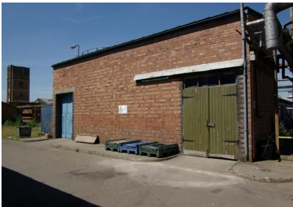
Figure 37 Building 71, southern elevation.
