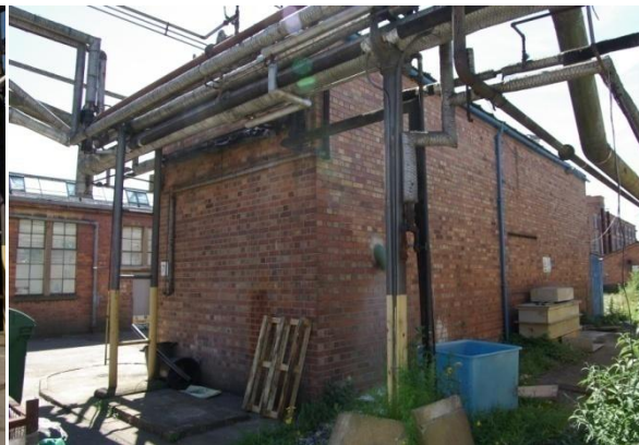
Figure 38 Building 71, northern elevation.
