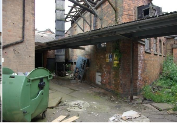
Figure 18 Building 44, showing the unusual angle of the northern gable.
