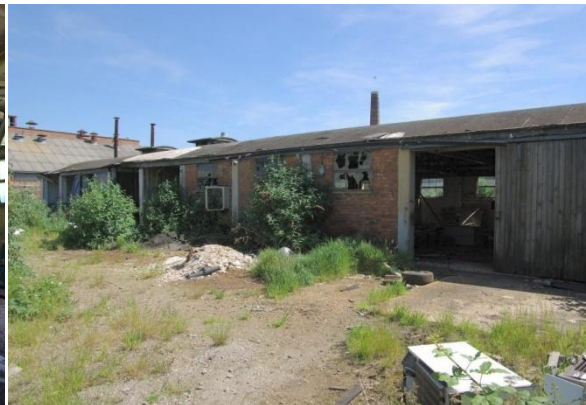
Figure 28 Building 55, Western Elevation.
