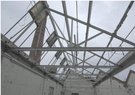
Figure 19 Building 44: Remains of roof structure.
