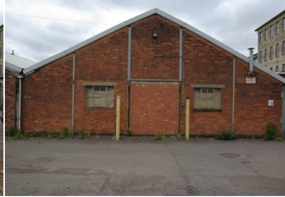
Figure 40 Building 72, Southern Elevation, Steel Frame.
