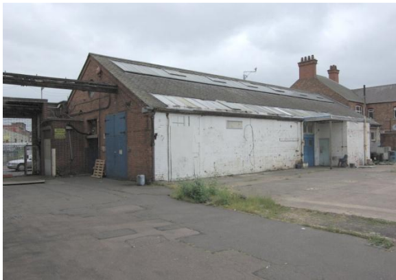
Figure 9 Building 33, West elevation.
