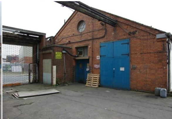
Figure 10 Building 33, Northern elevation.
