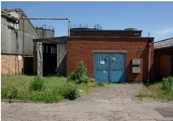
Figure 31 Building 65e, Western elevation.
