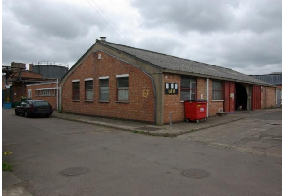
Figure 33 Building 67, Southern & Western elevations.
