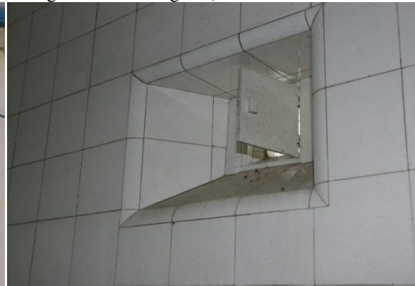
Figure 44 Building 72a: internal black out cover.
