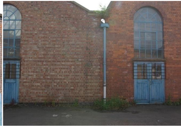
Figure 16 Building 42 Later Bay Added to the North.
