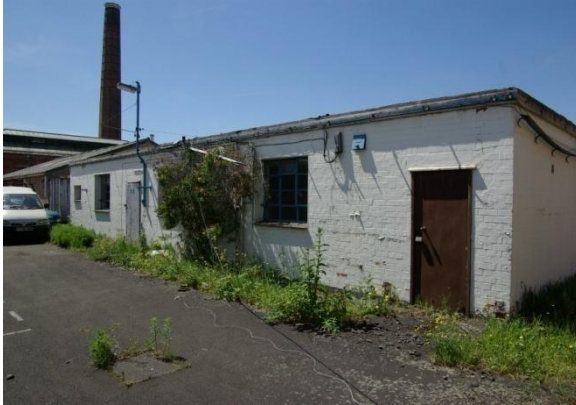
Figure 41 Building 72a, Eastern elevation.
