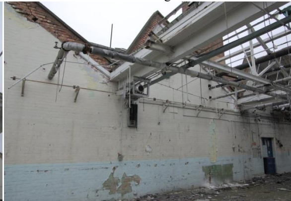
Figure 20 Building 44, original driveshaft.
