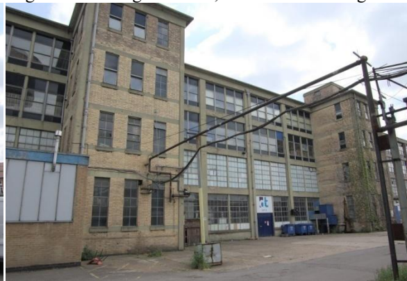
Figure 6. Building 39, Western Elevation.
