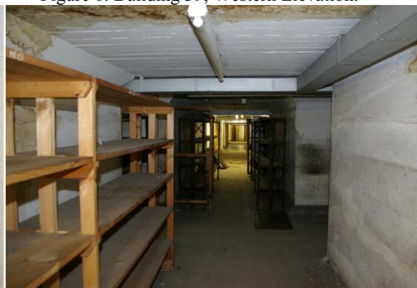
Figure 8 Building 96, General View of Cellar.
