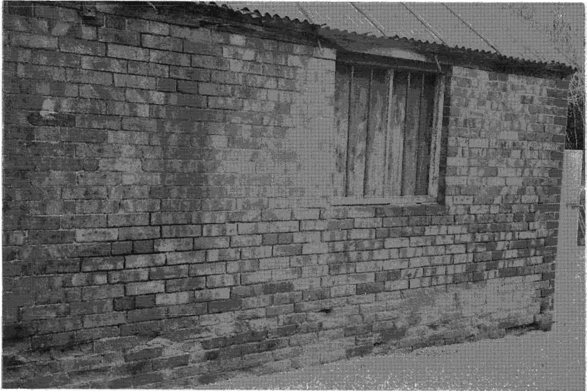
Plate 5 Brick side-wall of Bay 1, south-west elevation, showing the two-light window with metal glazing bars. The greater part of the brickwork is from the second phase and shows 'Haunchwood' brick being raised in a single bonding course of two headers and three stretchers alternating with three rows of stretchers, a variant form of Flemish Garden Wall Bond. The corrugated iron roof is also visible.
